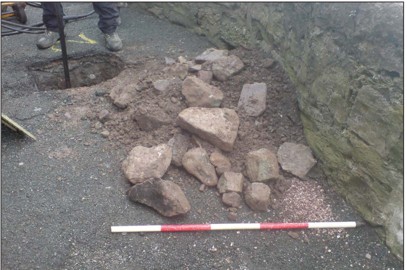
Plate 02 - Test pit measuring 0.50m x 0.50m opening the planned location of BH2 (SH4766762852)
