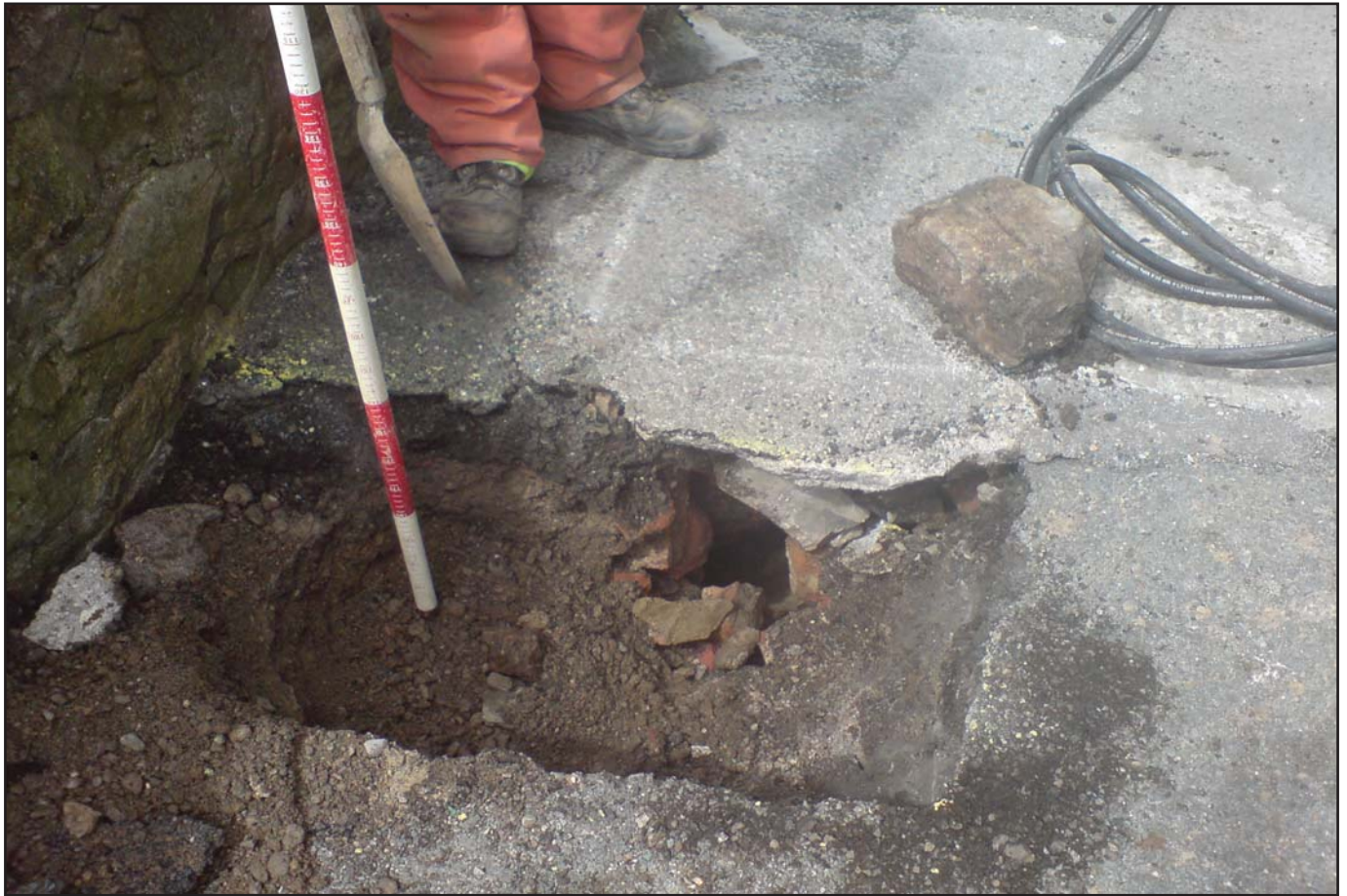
Plate 09: TP2A open in Porth Yr Aur Promenade showing the upper layers of the made ground behind the Promenade Wall and the opening of the void which extends northwards
