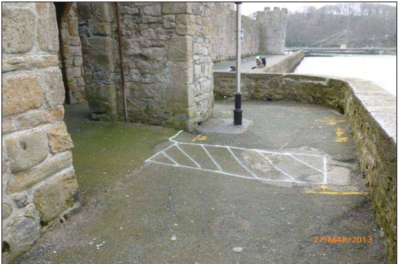
Plate 05: Intact cobbled surface uncovered immediately below the tarmac in TP1 within the Barbican of Porth Yr Aur.
