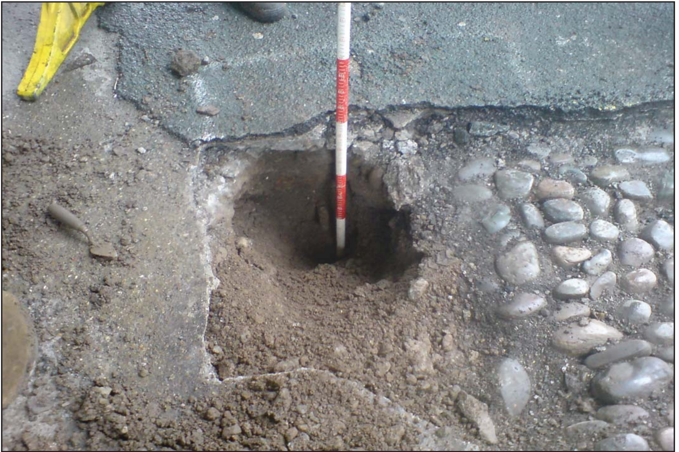
Plate 07: Test Pit opened in south eastern corner of TP1. The steel reinforcing bar is visible in the base of the test pit.
