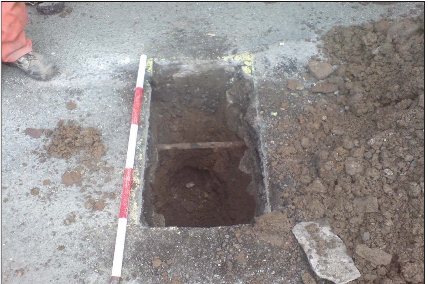
Plate 10: TP2B open in Porth Yr Aur Promenade showing the location of the service running north-south across the Pit
