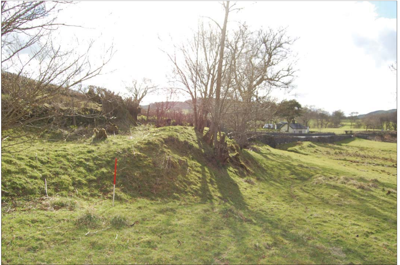
Plate 05 - Road embankment constructed against the face of the retaining wall at Chainage 290. Not indicated on Scheme Drawing S/206/DT 001 (DRAFT) as an embankment.
