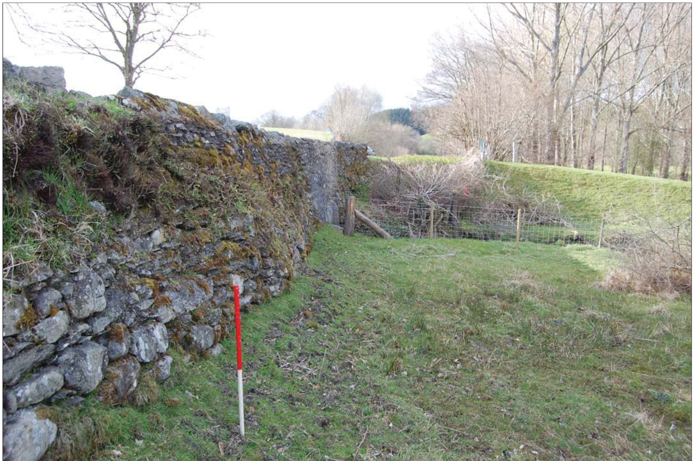
Plate 08 - The north face of the retaining wall at Chainage 530 showing different phases of repair identified during the archaeological assessment. In the centre of the image at Chainage 550 is the culvert under the A5(T) carrying Nant Heulog from south to north to discharge into the Afon Alwen.
