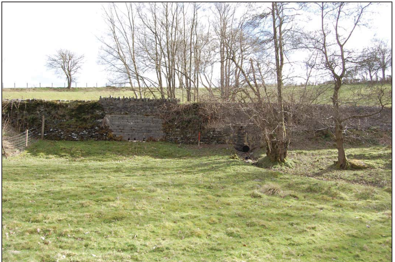
Plate 02 - The north face of the retaining wall at Chainage 140 showing different phases of repair identified during the archaeological assessment. Visible to the right of the ranging pole is the current road surface water drainage scheme at this point.
