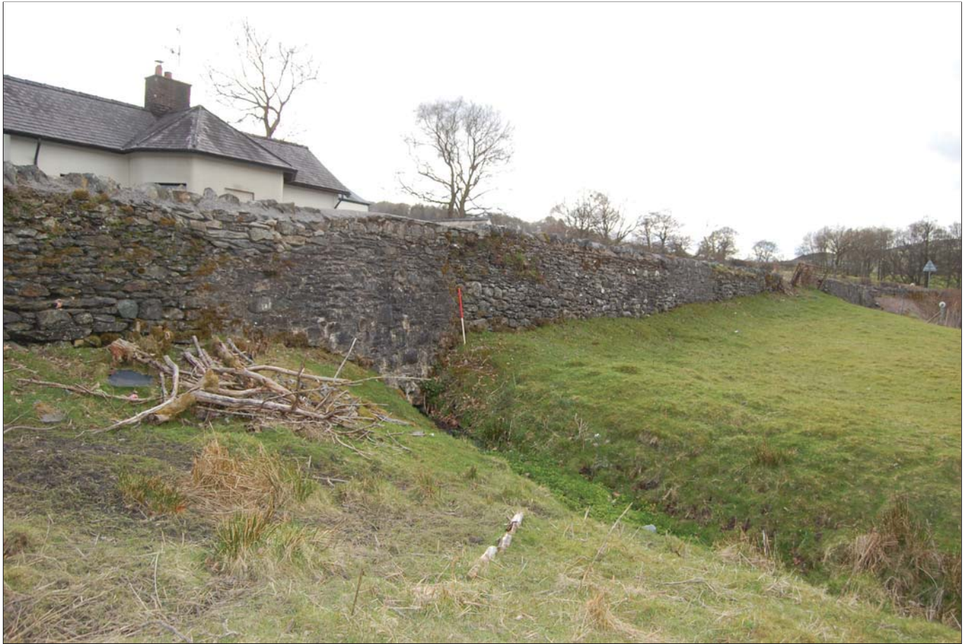
Plate 07 - The north face of the retaining wall at Chainage 400 showing different phases of repair identified during the archaeological assessment. Visible to the left of the ranging pole is the current road surface water drainage scheme at this point.
