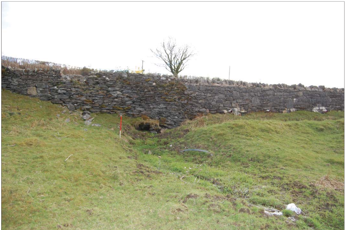
Plate 06 - The north face of the retaining wall at Chainage 350 showing the different phases of repair identified during the archaeological assessment. Visible to the right of the ranging pole is the current road surface water drainage scheme at this point, and appears to be an original Telford specification drain fed into by modern drainage.
