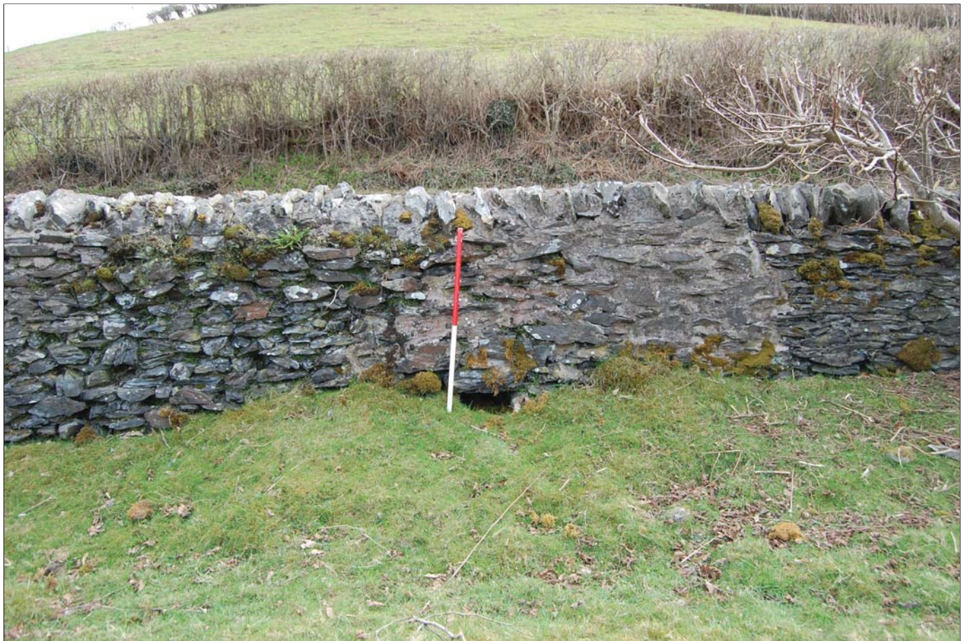
Plate 04 - The north face of the retaining wall at Chainage 170 showing the different phases of repair identified during the archaeological assessment. Visible to the right of the ranging pole is the current road surface water drainage scheme at this point, and appears to be an original Telford specification drain.
