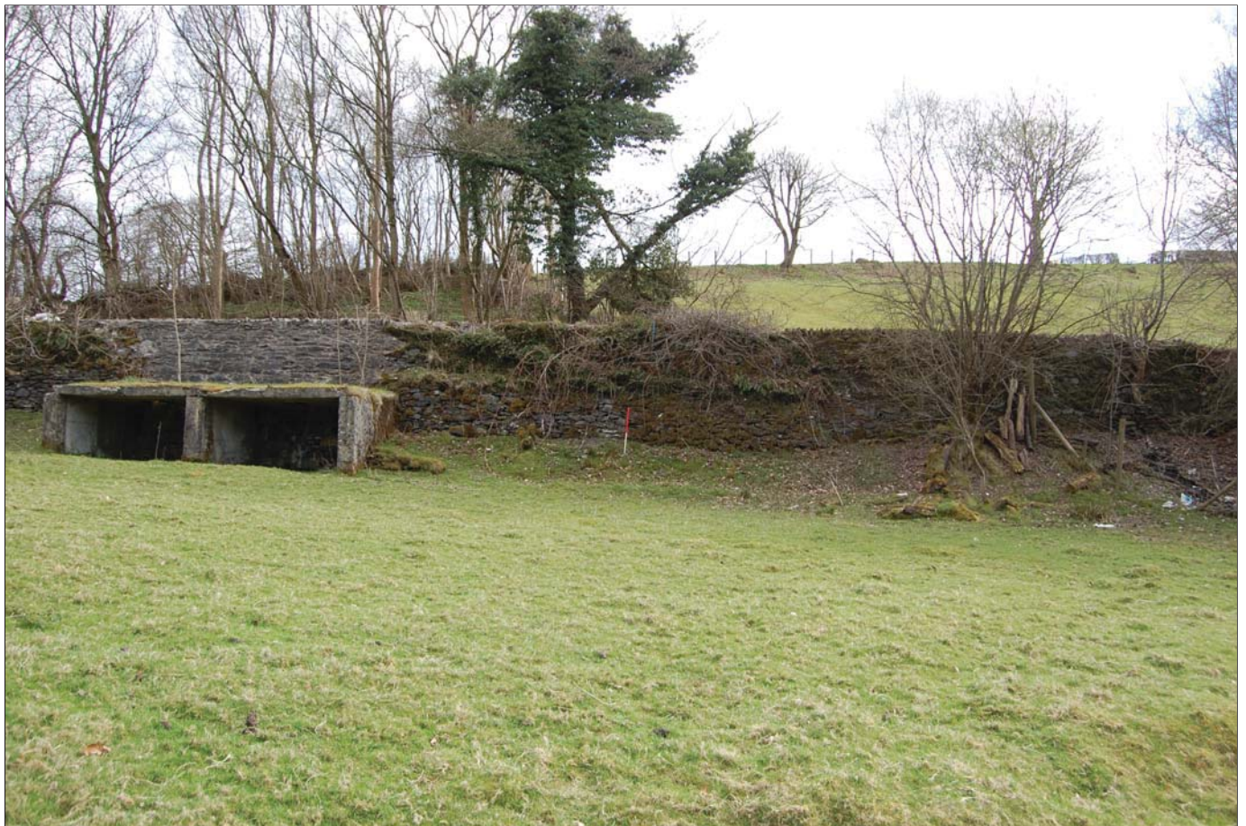
Plate 12 - The north face of the retaining wall at Chainage 120 showing different phases of repair identified during the archaeological assessment. The open fronted concrete structure is recorded on Scheme Drawing S/206/DT 001 (DRAFT) as 'Concrete pump house'.
