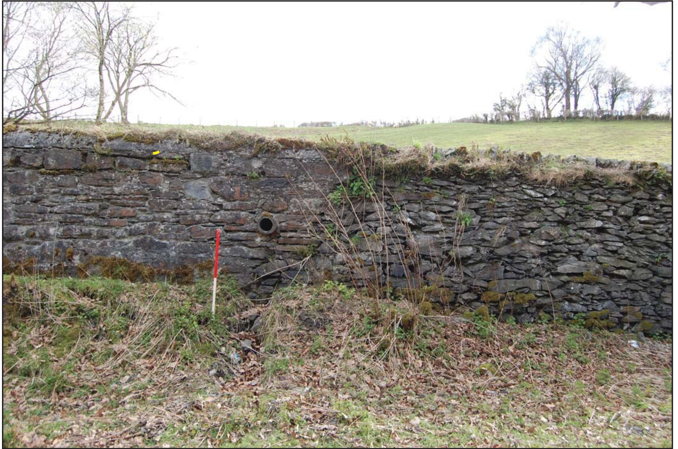
Plate 03 - The north face of the retaining wall at Chainage 160 showing the different phases of repair identified during the archaeological assesment. Visible to the right of the ranging pole is the current road surface water drainage scheme at this point.
