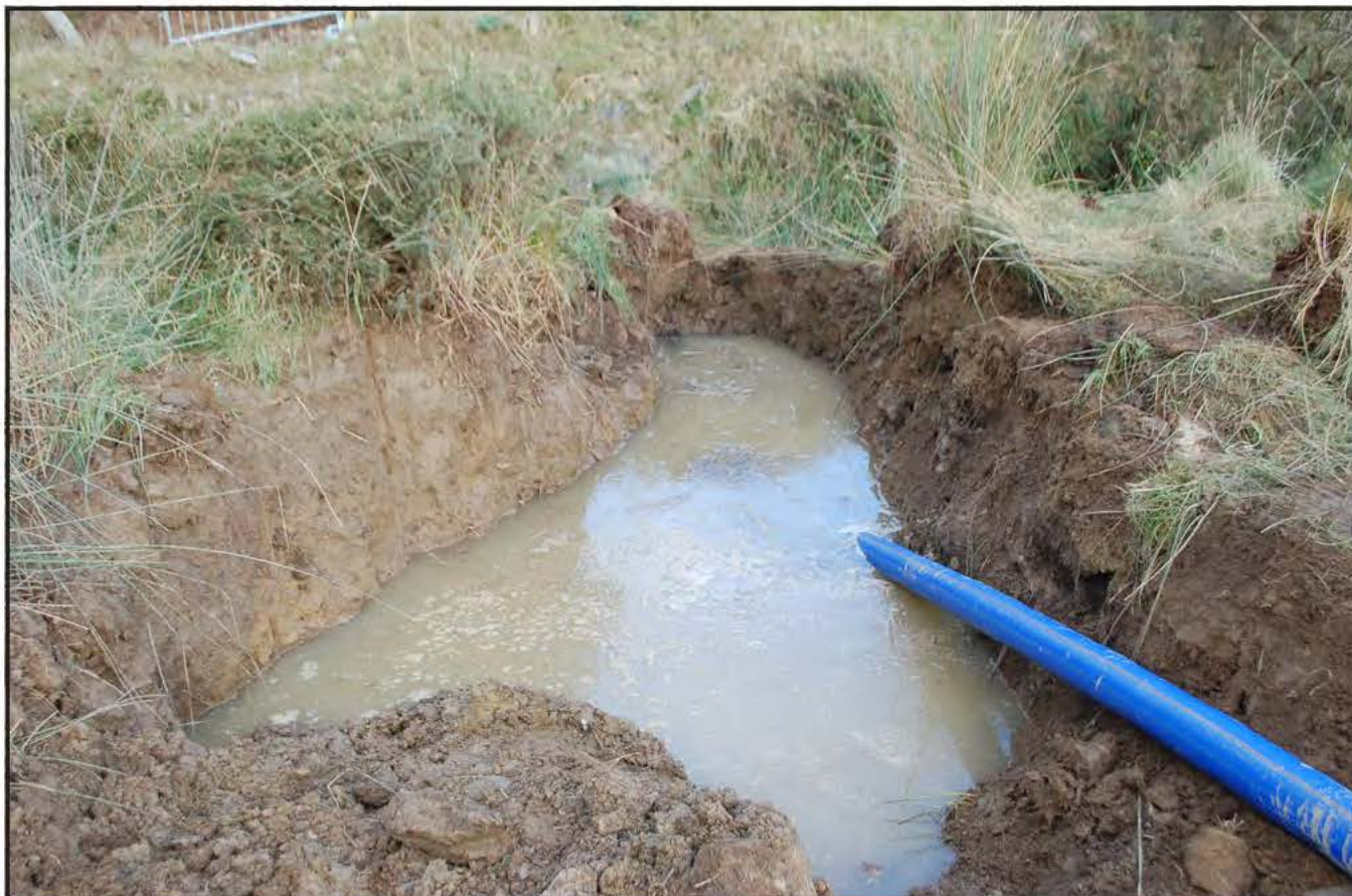
Plate 9: Pit 8/Field 7 - detailing topsoil, subsoil and ingress of water. The pit is located immediately to the south of a drainage ditch in a very wet field. The new main is visible on the right of the picture. View from the South.
