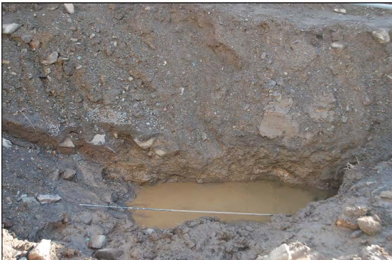
Plate 4: Pit 4/Field 3 - West facing section, detailing limit of excavation and water ingress. Visible in section is extensive overburden associated with a local residential build. Beneath the overburden is existing topsoil and subsoil. Scale = 1 metre
