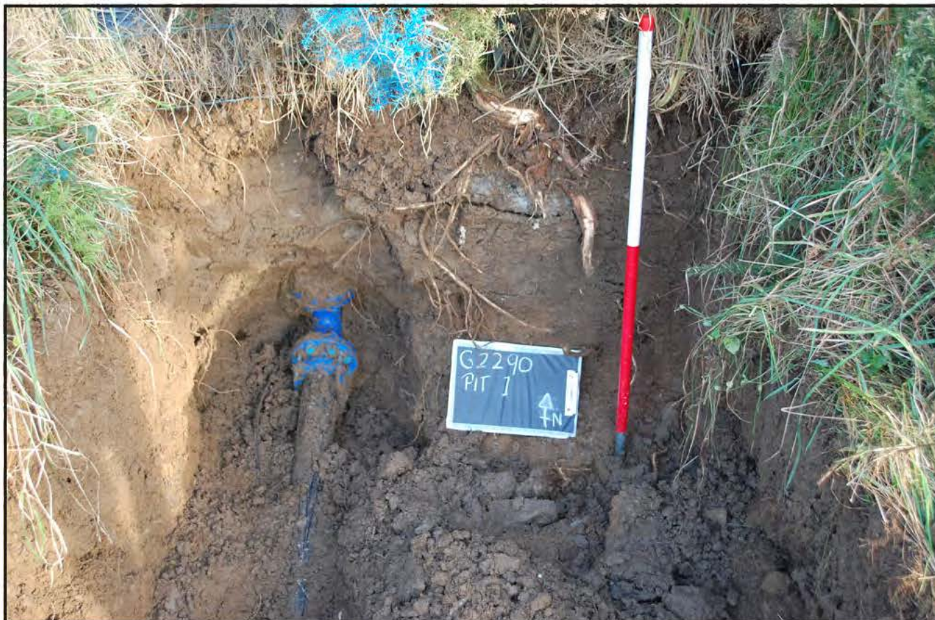
Plate 1: Field 1/pit 1 - south facing section detailing topsoil, subsoil, 1960' water main and valve. Scale = 1 metre.
