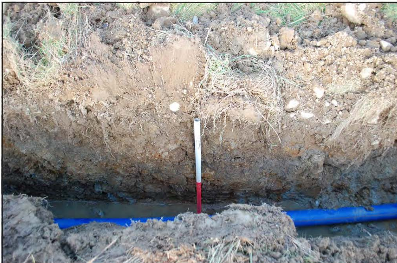
Plate 11: Open cut trench B/Field 7 - South facing section detailing topsoil, subsoil, the new pipe can be seen in the base of the trench which was waterlogged. Scale = 1 metre.
