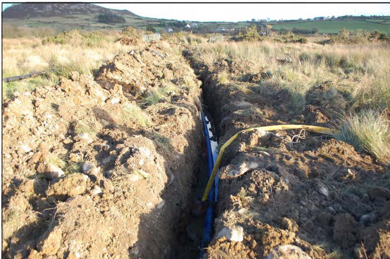
Plate 12: Open cut trench B/Field 7 - view to the East North East showing new pipe in the bottom of the trench. The trench had been waterlogged and was pumped out with a submersible pump which can be seen in the foreground alongside the pipe. The trench was approximately 40 metres long, 0.5 metres wide, and between 1 metre and 1.2 metres deep. Scale = 1 metre.
