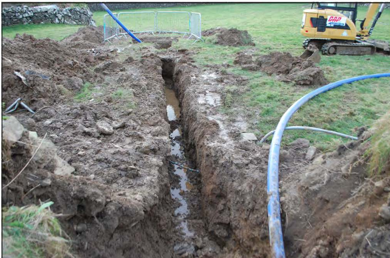
Plate 10: Open cut trench A/Field 4 - view to the South and Pit 5 from the Northern boundary wall. A domestic service pipe can be seen crossing the trench which is waterlogged at the base.
