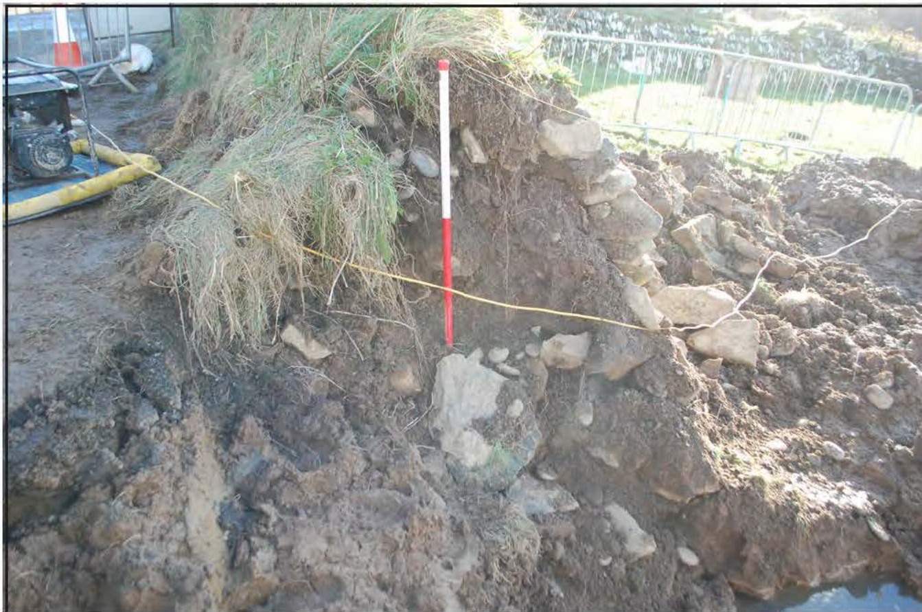
Plate 5: Breakthrough of wall at Northern end of Field 4 showing West facing section. The wall forms a boundary with the local road which is visible on the far left of the picture. Scale = 1 metre.
