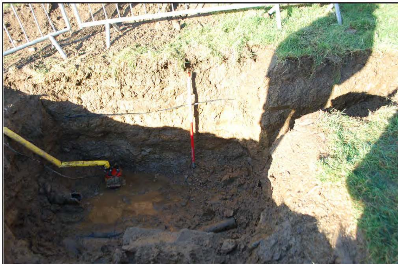
Plate 6: Pit 5/Field 4 - East facing section, detailing topsoil, subsoil and 1960's water main. The pit was waterlogged and a submersible pump is visible at the bottom of the pit. Scale = 1 metre.
