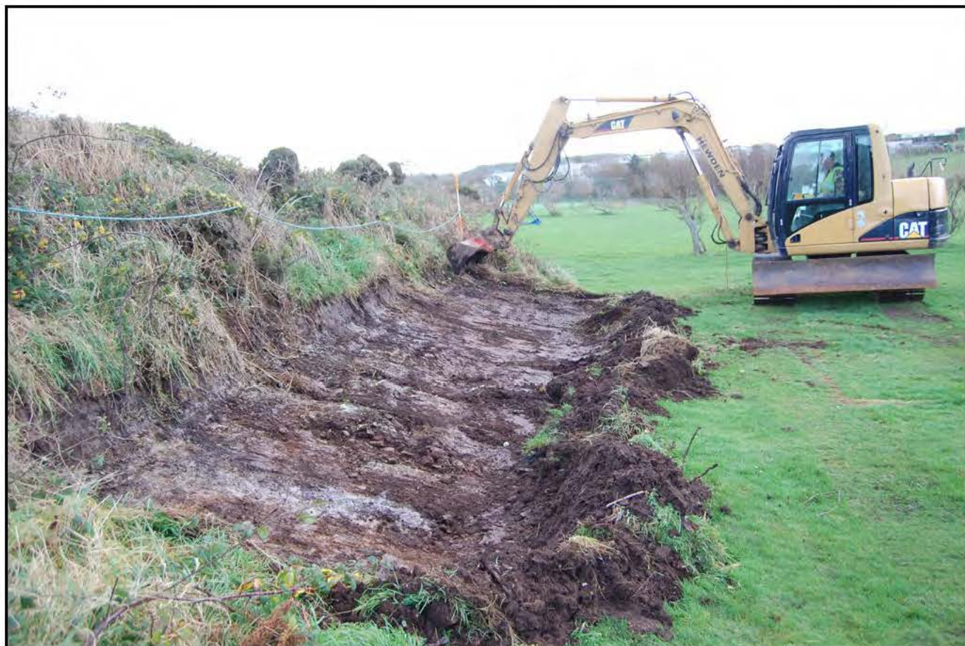
Plate 04 - Controlled stripping of the north end of the proposed development - exposing the dip of the rockface under the topsoil, subsoil and natural.
