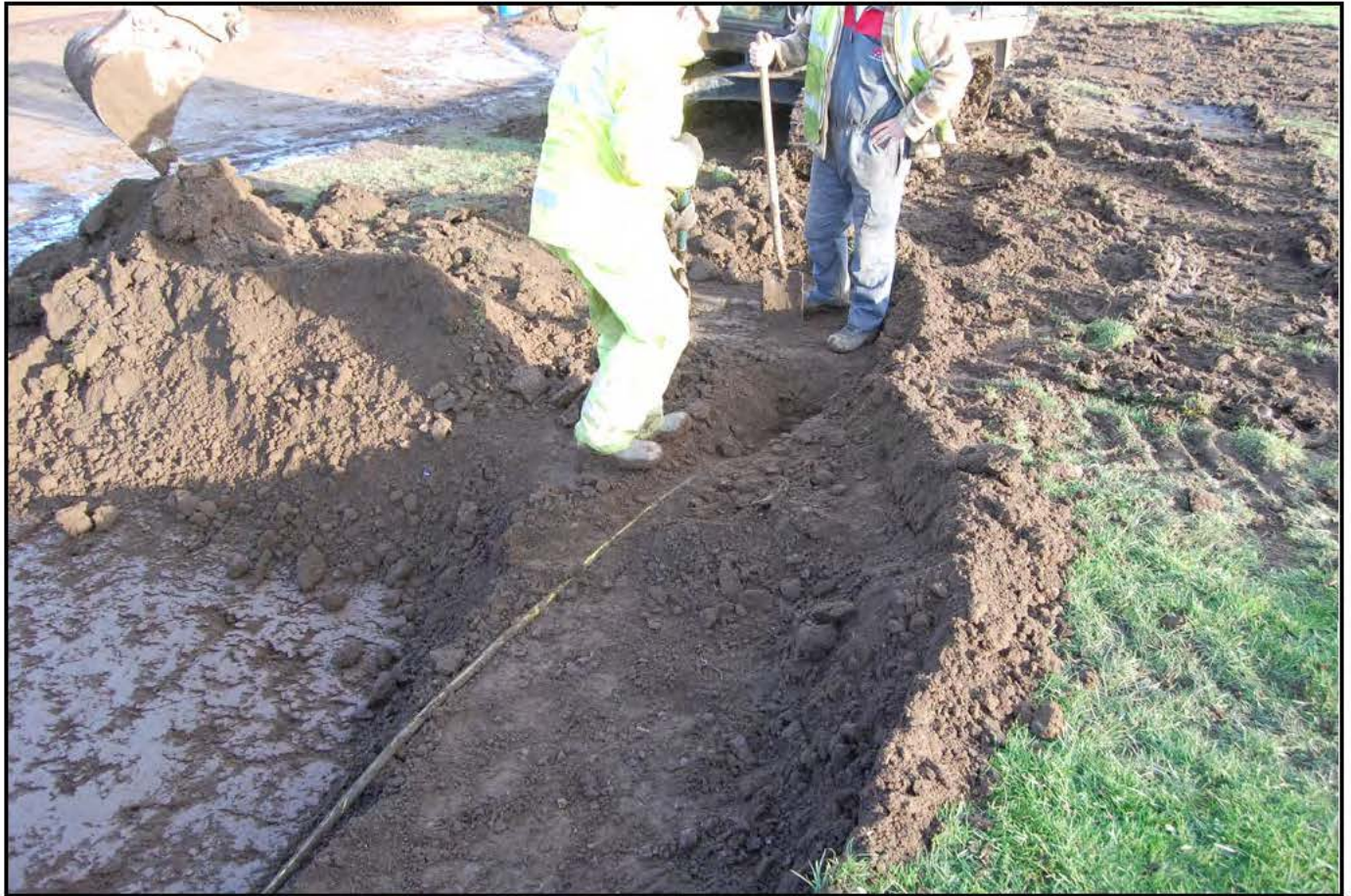
Plate 11 - Exposure of the local services Liquid Propane Gas (LPG) pipe running west to east across the stripped area.
