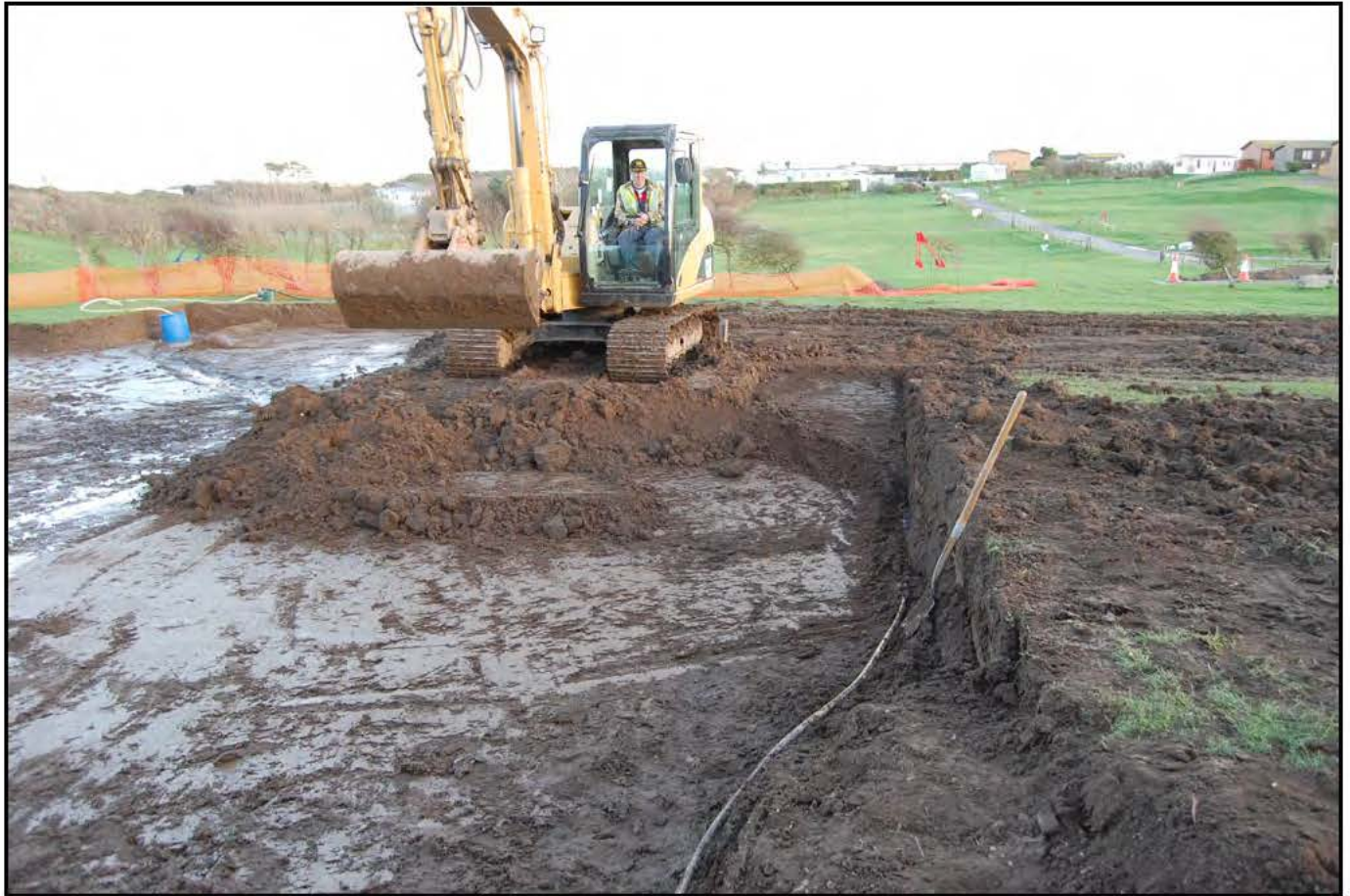
Plate 05 - Exposure of the local services Liquid Propane Gas (LPG) pipe crossing the area of controlled stripping. A sump excavated to aid drainage is visible in the background.
