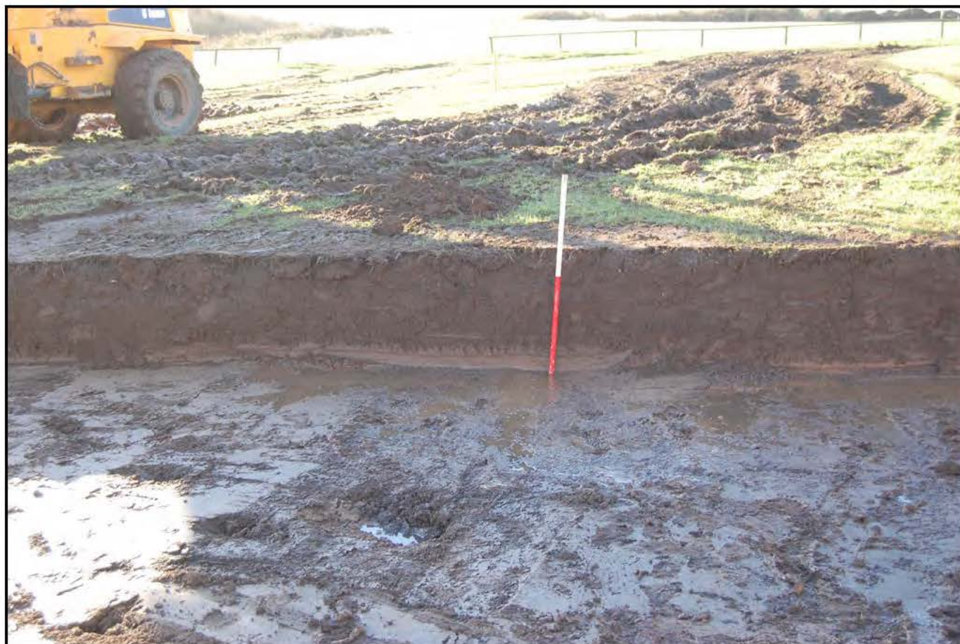
Plate 08 - Typical section through the controlled stripping works - exposing the depth of topsoil and subsoil above the natural.
