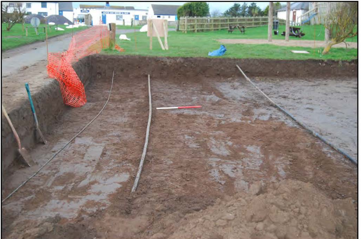
Plate 12 - Exposure of local services Electricity cable and two Water pipes running west to east across the stripped area.
