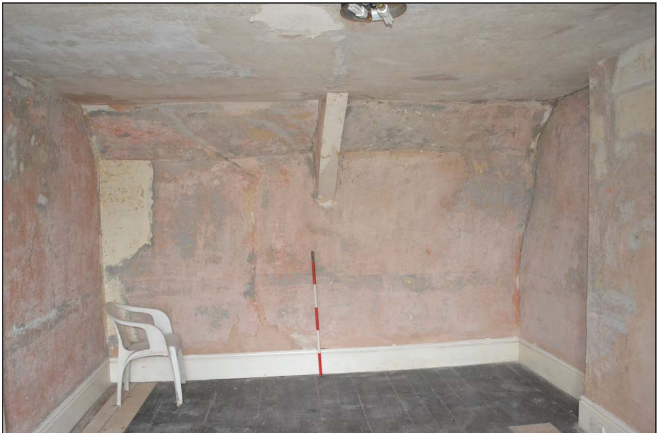
Plate 18: Bedroom 1 from the northwest showing base of truss, 1.0m scale.
