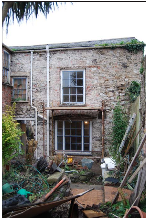
Plate 26: Removal of render on the northwest elevation showing replaced first floor window.
