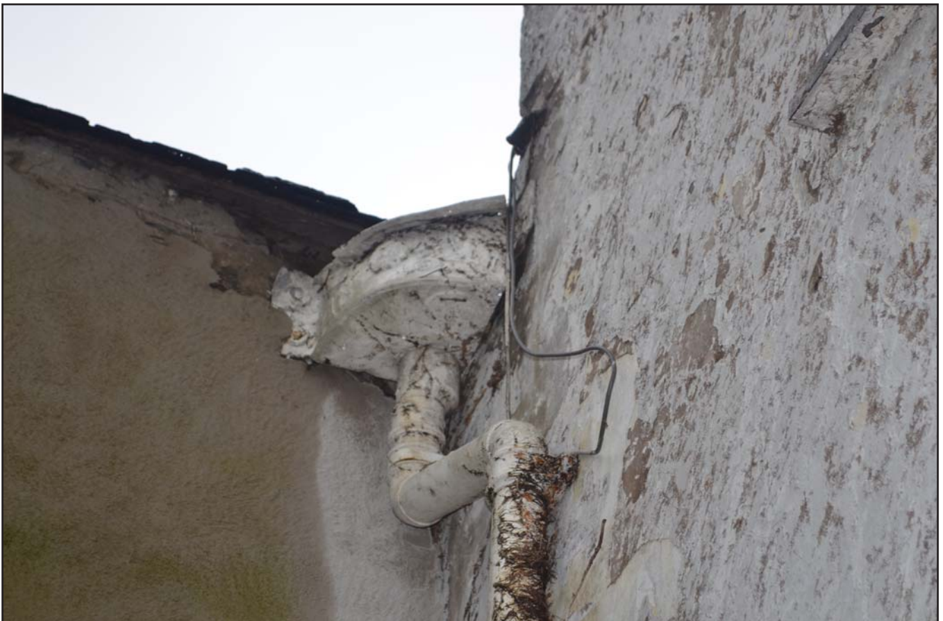
Plate 08: Rain hopper on the northwest external elevation, showing the date 1834.
