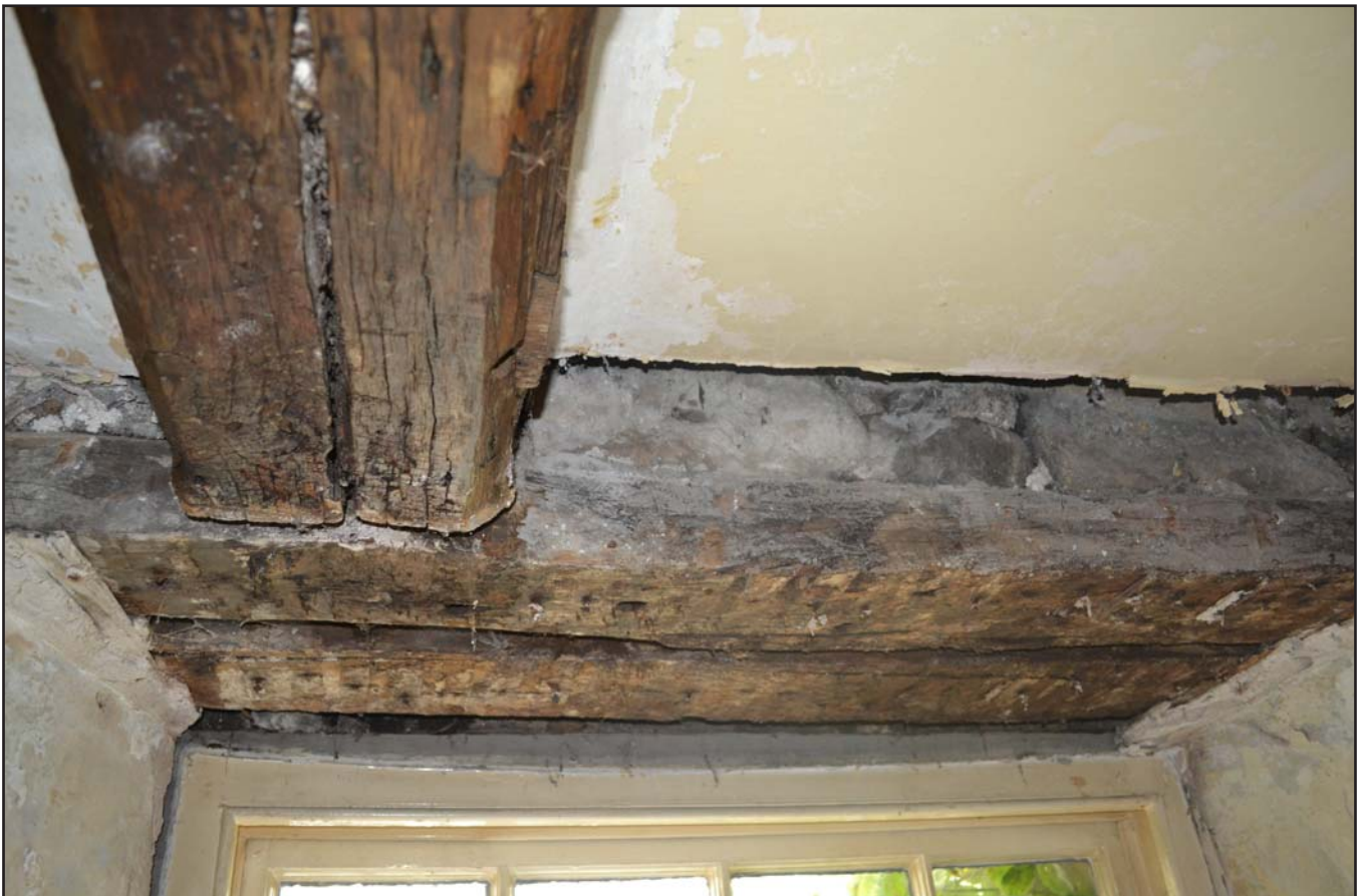
Plate 30: Roughly hewn beam with chamfers and stops in the kitchen, from the northwest
