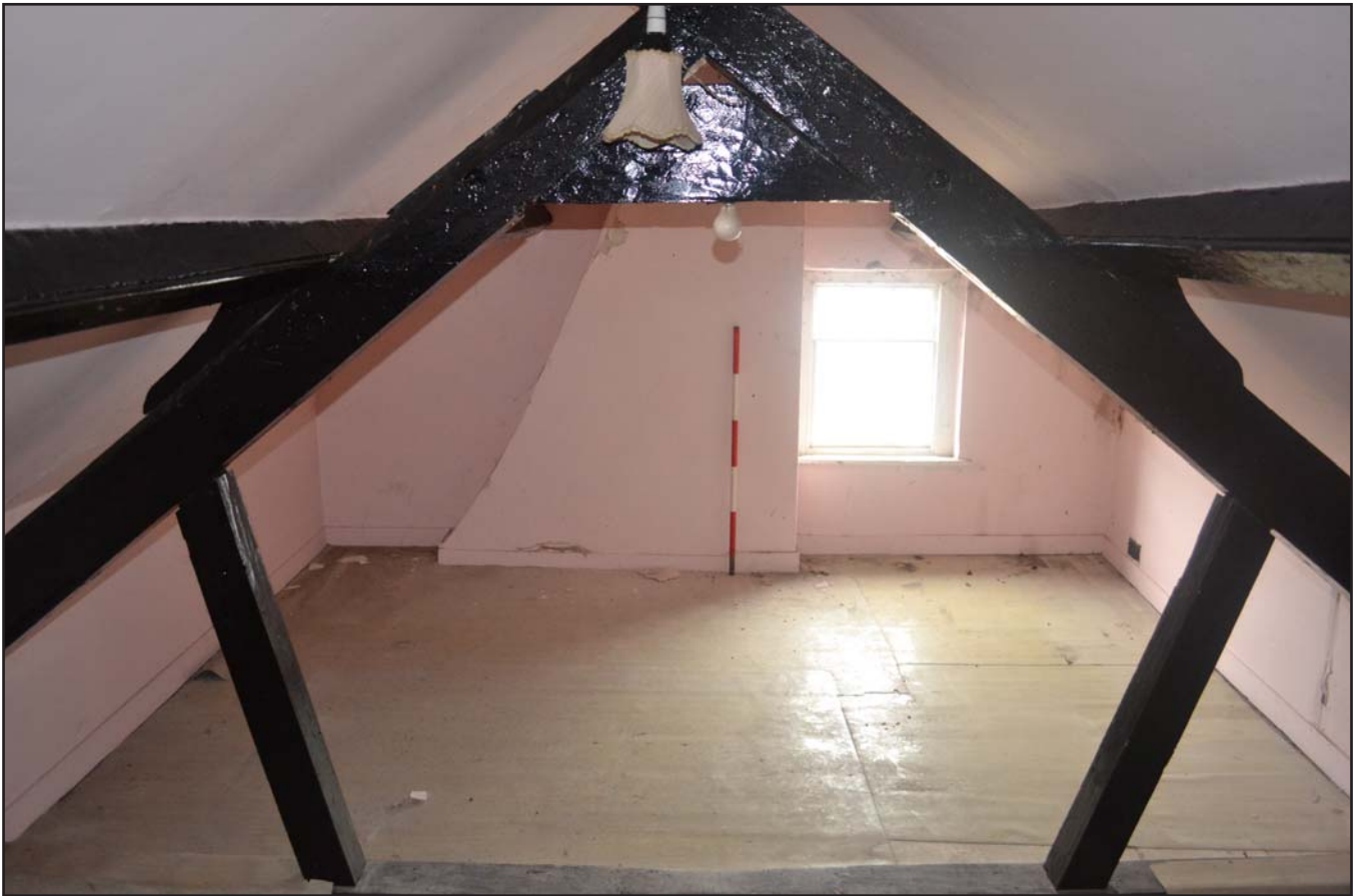
Plate 23: Bedroom 6 from the southeast showing truss, 1.0m scale.
