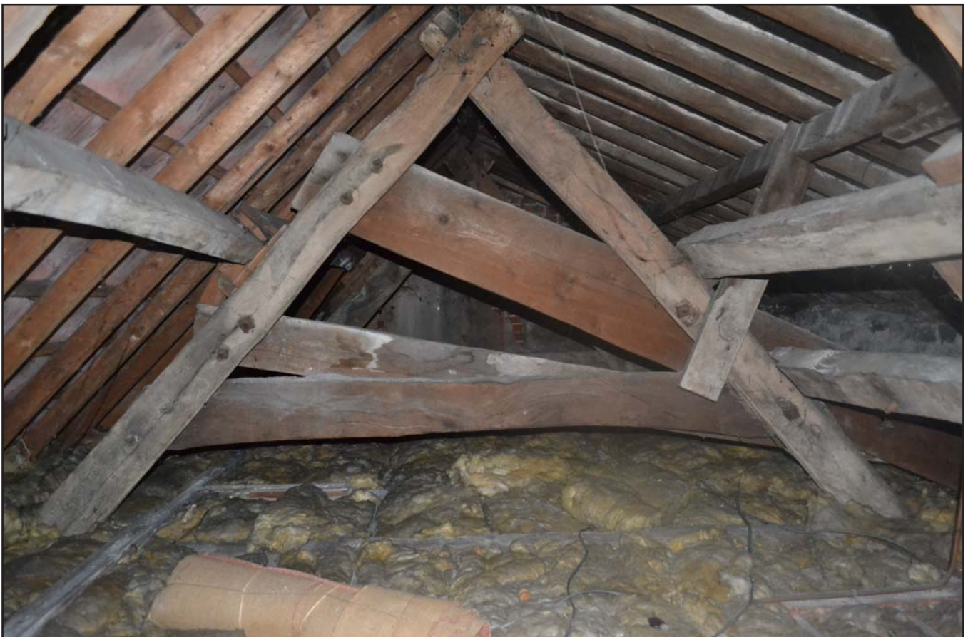
Plate 22: Roof Void from the northeast showing truss and raised roof pitch.
