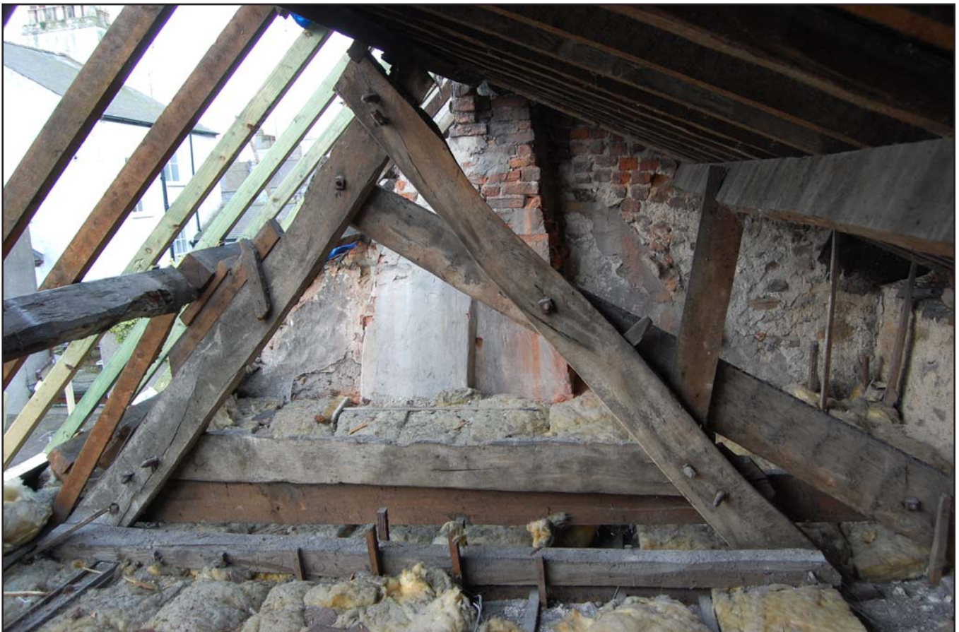
Plate 28: Exposed roof trusses showing roof extension from the northeast.
