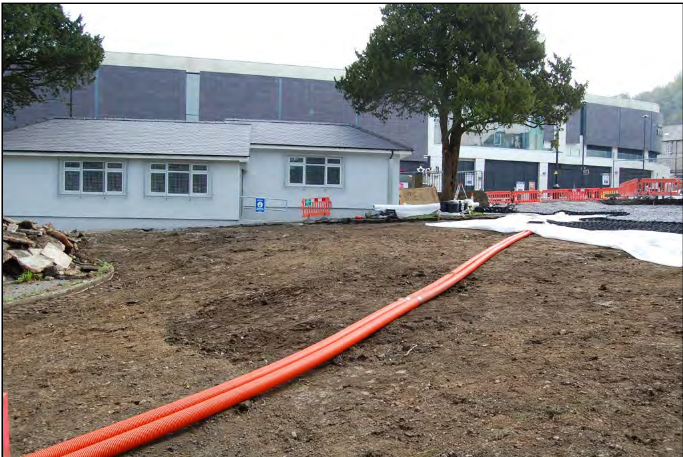
Plate 08 - Detailed view of the centre/eastern corner of the park, after completion of the topsoil strip. Note the shallow excavation depth (less than 100mm) and the orange ducting laid beneath the geotextile membrane: the ducting was used for running cables that powered illuminated bollards; the ducting was not buried into the stripped are, but laid onto the surface. The darkened area is a shrub plantation previously removed (cf. Plates 01 and 02).
