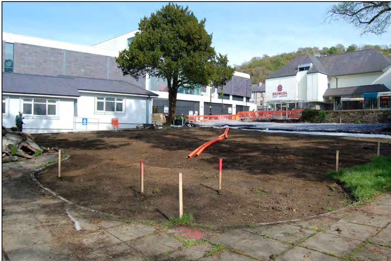
Plate 07 - General view of the centre/eastern corner of the park, after completion of the topsoil strip. Note the shallow excavation depth (less than 100mm) and the orange ducting laid beneath the geotextile membrane: the ducting was used for running cables that powered illuminated bollards; the ducting was not buried into the stripped are, but laid onto the surface.
