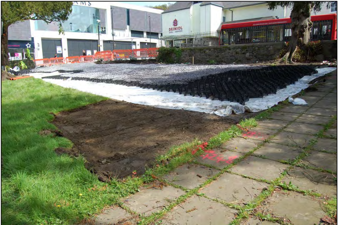
Plate 06 - General view of the eastern corner of site during the foundation groundworks for the new pathway. Note the use of geotextile membrane, followed by a geocell that was sealed by imported slate waste (used as a sub-base). A small portion of stripped ground can be seen in the foreground: the limit of excavation was 100mm or less. the pathway slabs also visible in the foreground were also removed and replaced.
