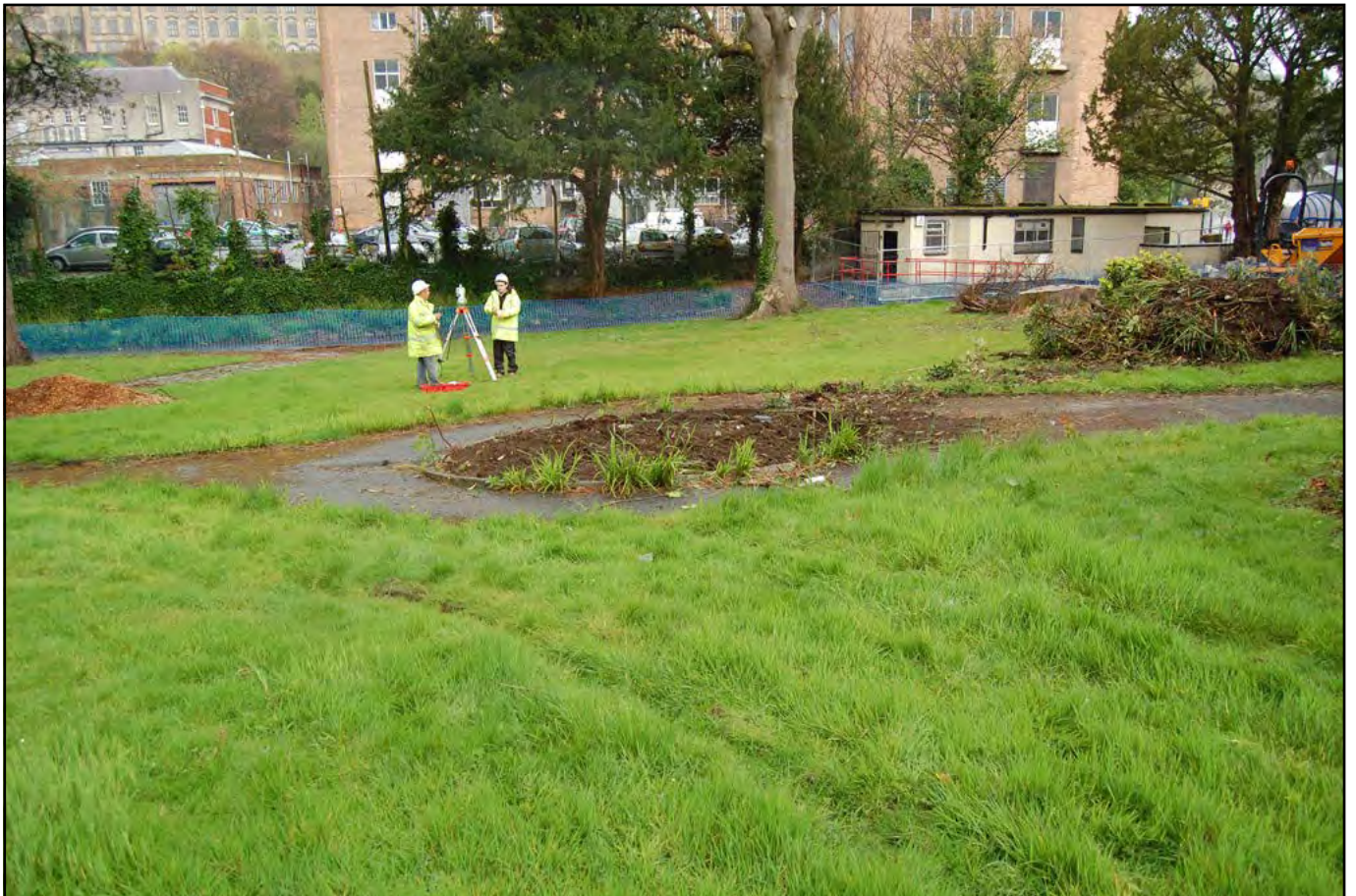
Plate 02 - View north of shrub plantation removal after stripping. This plantation area was located towards the centre of the publicpark area and was replaced both by the new concrete paving as well as a rectangular shaped plantation area. The grassed area in the foreground was also removed to accommodate the new concrete paving
