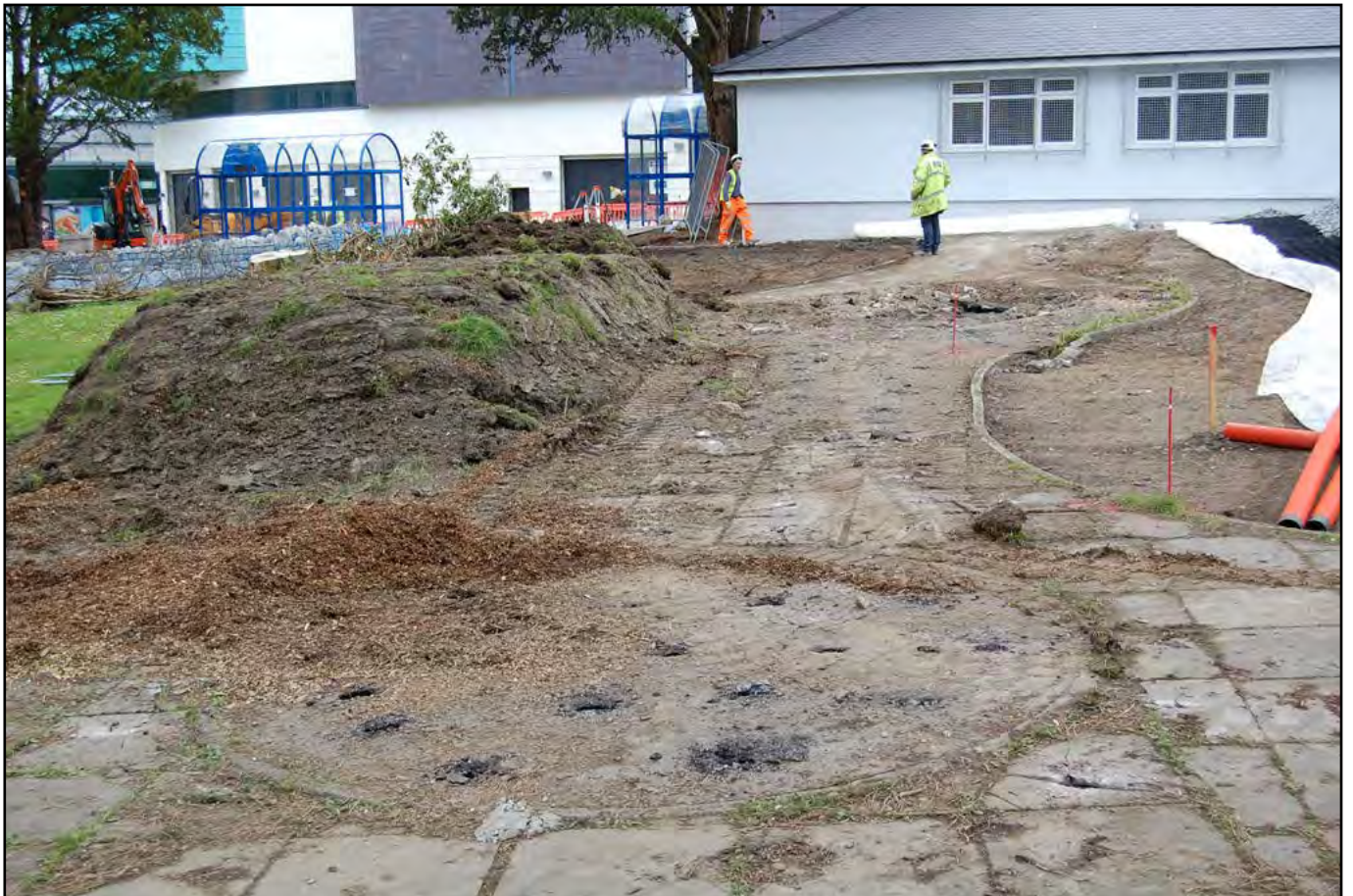
Plate 10 - Alternative view of stripped area detailed in Plate 09; the stripped area can be seen at the top of the image, whilst the original pathway can be seen in the foreground. Note the perforations in the pathway: the geotextile, geocell and sub-base were laid directly on top of the path at this location, rather than the path removed, due to the change in levels; the perforations allowed the original path to drain freely.
