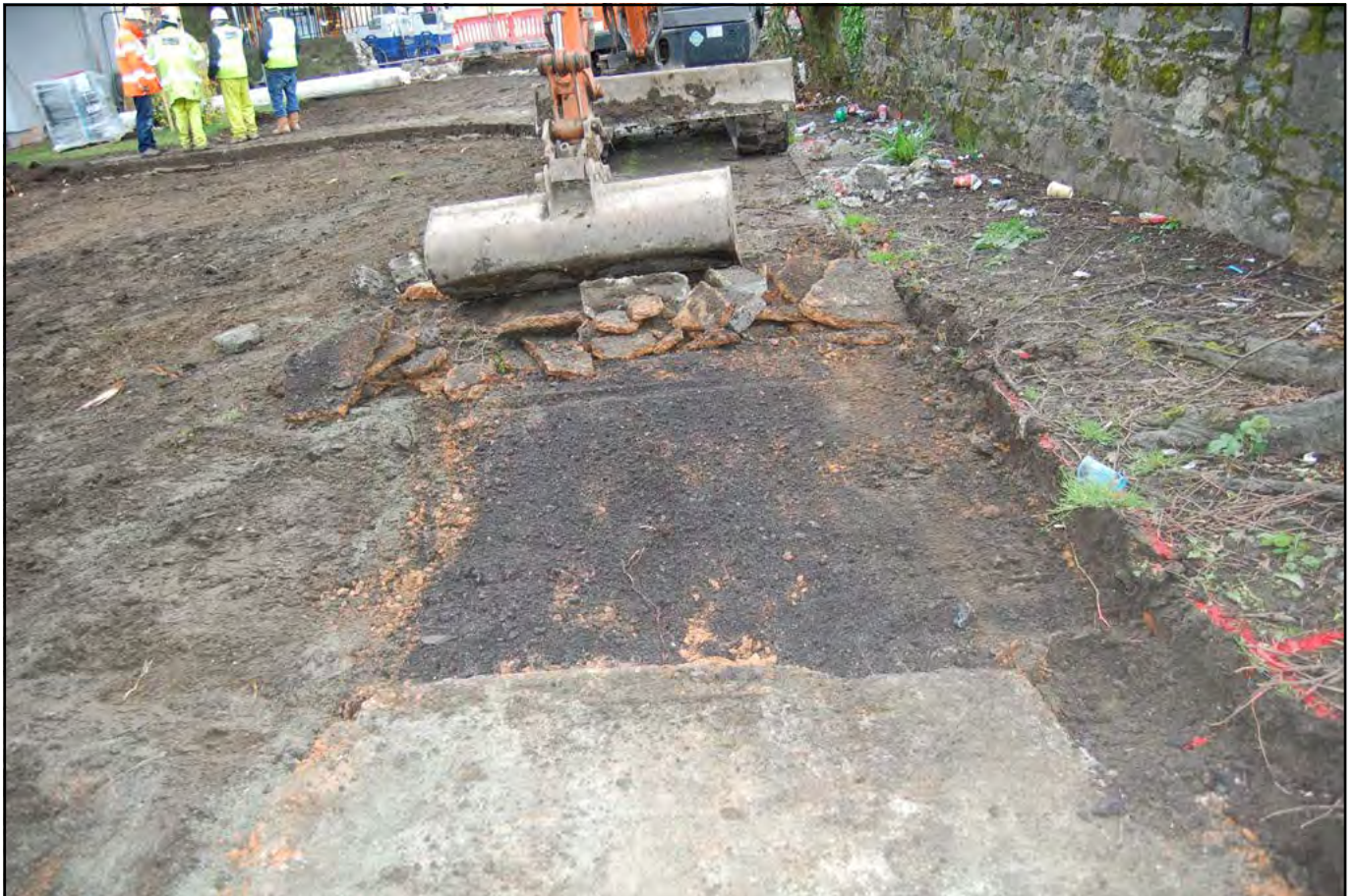
Plate 04 - General view of eastern corner of site during removal of existing pathway foundation material (visible in Plate 03). Beneath the pathway slabs were a concreted deposit followed by a thin clinker type deposit that was specifically laid as part of the foundation construction. This area was replaced by a new pathway. Limit of excavation was 100mm
