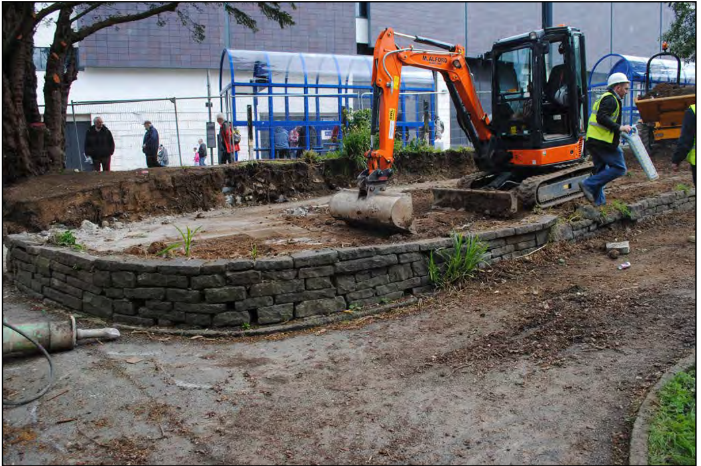
Plate 11 - View northeast of removal of an original planter. The planter had been built up from ground level and edged with unbonded stone (four courses high). The depth of the built up material forming the centre of the planter can be seen at the back of image close to the bus shelters. The exposed surface beneath the machine bucket was not breached: the area was subsequently built up and edged with re-dressed stone recovered from the boundary wall demolition zones.
