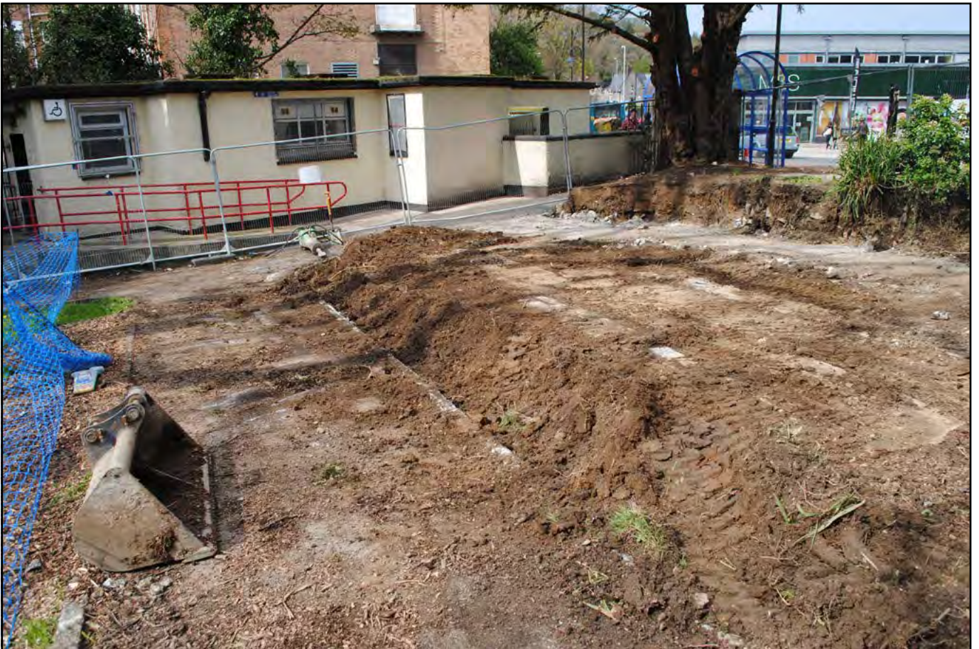
Plate 12 - View north-northwest of the planter area after the removal of the existing wall visible in Plate 11. There was no significant foundation cut or foundation course: the wall was set into a topsoil deposit. The area was subsequently built up and edged with re-dressed stone recovered from the boundary wall demolition zones.
