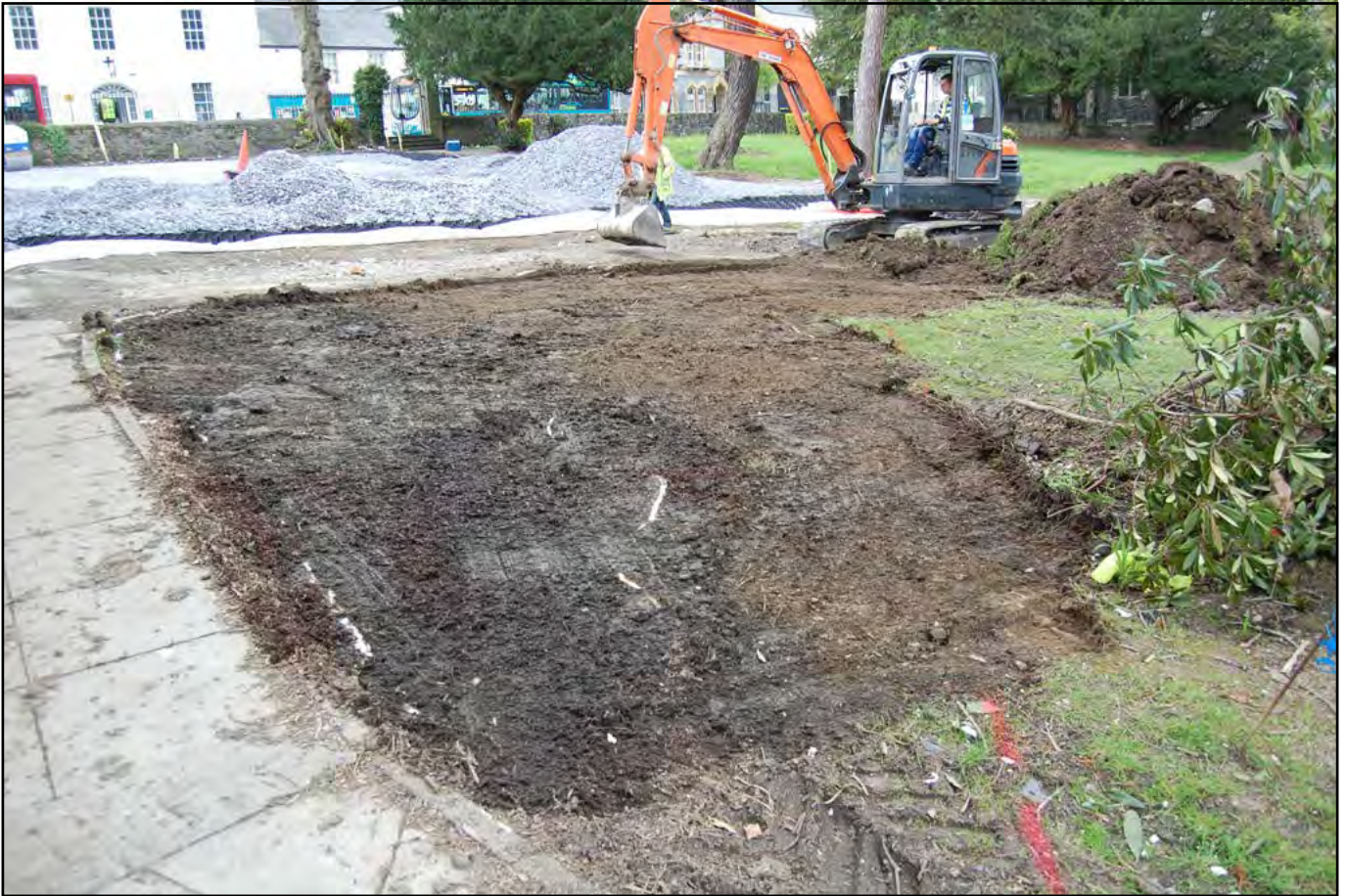
Plate 09 - View southeast of topsoil strip for the new pathway. The spray painted red line on the grass denotes the northern extent of the strip. Note the shallow depth, which is less than 100mm and deliberately kept higher to avoid damage to tree roots. As with the area visible to the top left of the image, the strip deposit was sealed with geotextile membrane, geocell and imported sub-base. The path was also removed.
