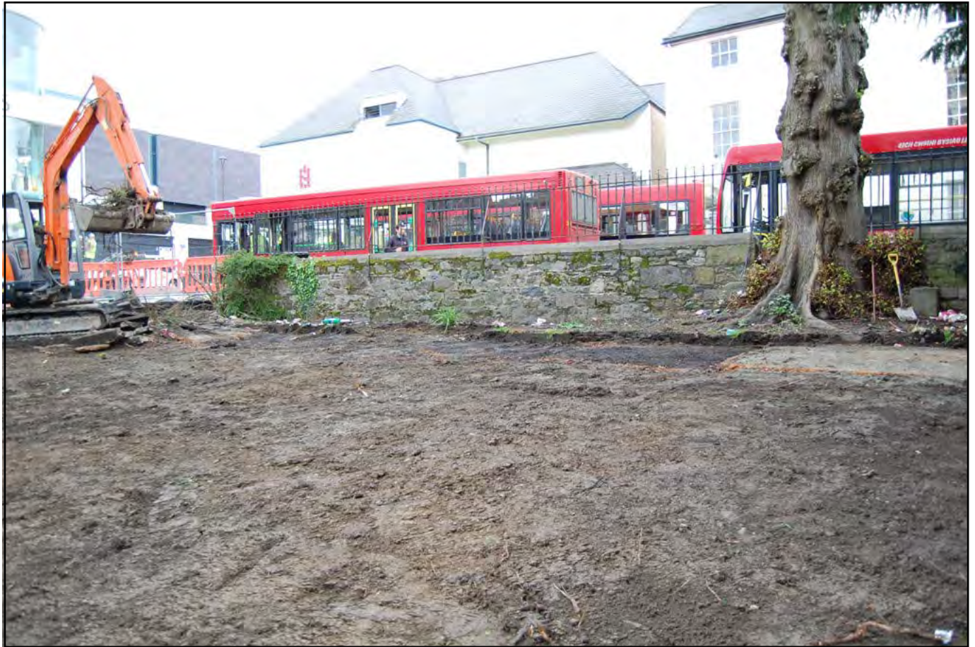
Plate 05 - General view of the eastern corner of site during removal of the pathway foundation material; this included a concreted deposit followed by a thin clinker type deposit that was specifically laid as part of the foundation construction. Note the portion of pathway foundation retained beneath the tree canopy. This area was used for the new pathway that encompassed the southeastern end of the site.
