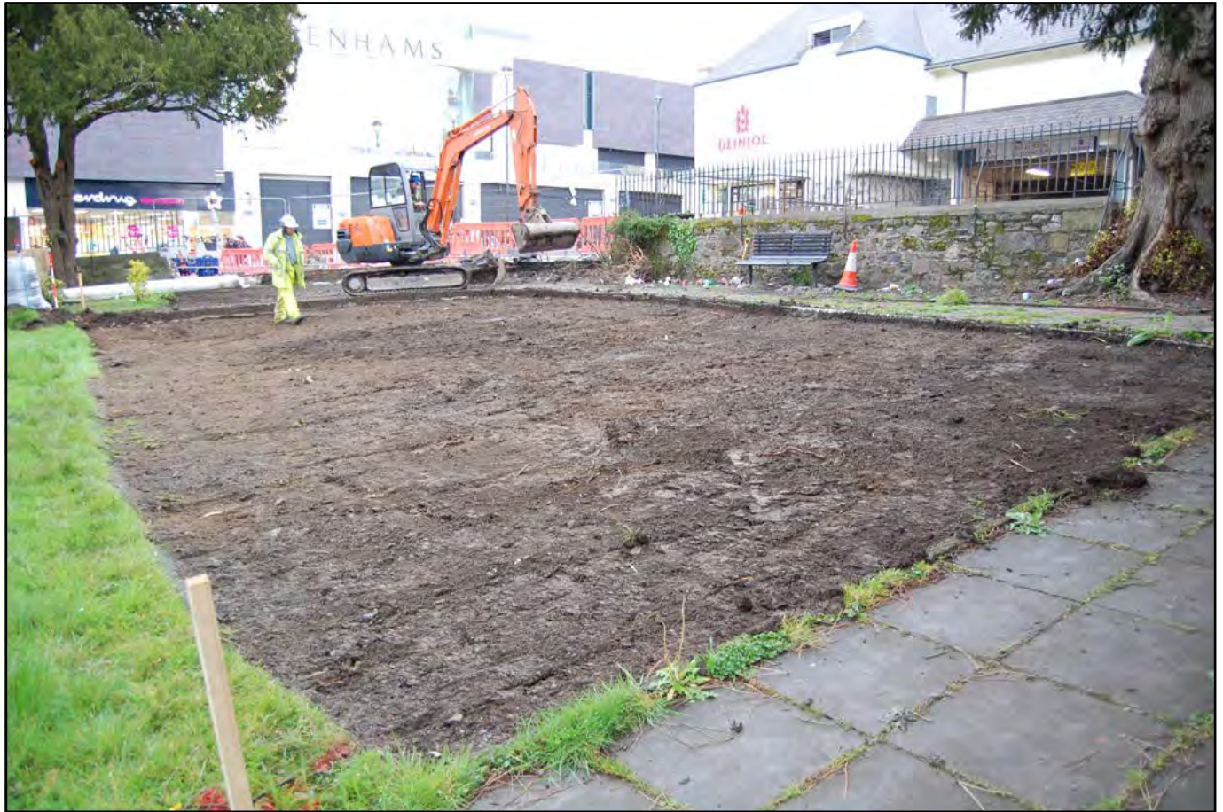
Plate 03 - General view of southeastern corner of site during stripping; excavation depth is less than 100mm; note that the strip has not exceeded the topsoil horizon; the former location of the plantation in Plates 01 and 02 is visible in the centre as a darkened area
