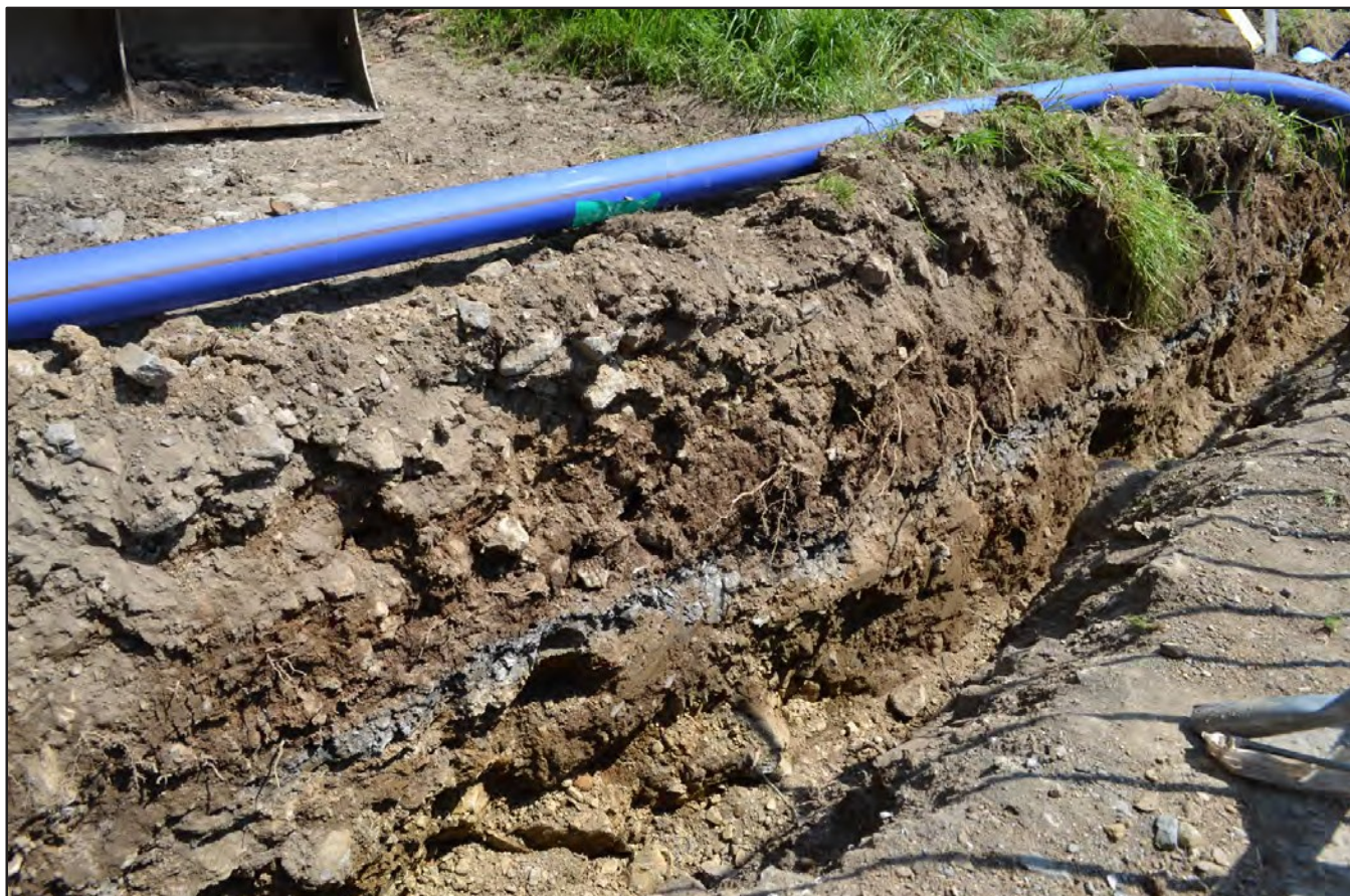
Plate 09: Section E with the old road surface of Tarmacadam and crushed slate sub-base layer running along section at a depth of 0.50m. View from the SW.
