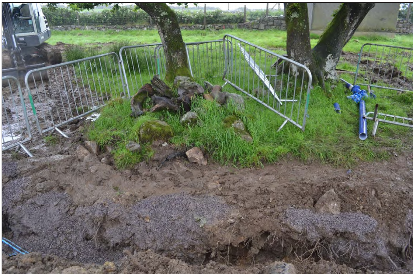
Plate 11: Earth and stone boundary truncated by pipe trench, no features , buried soil or cut below the surface boundary. Section L. View from the ESE.
