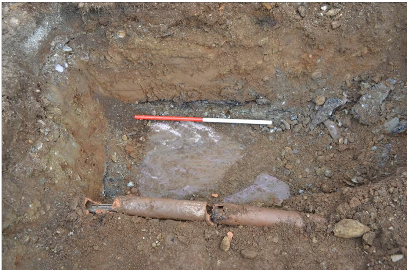
Plate 03: Trial hole 02. Shows purple slate capped culvert and band of Tarnacadam with a sub-base of crushed slate above it, in section, part of the old road.. View from the SW.
