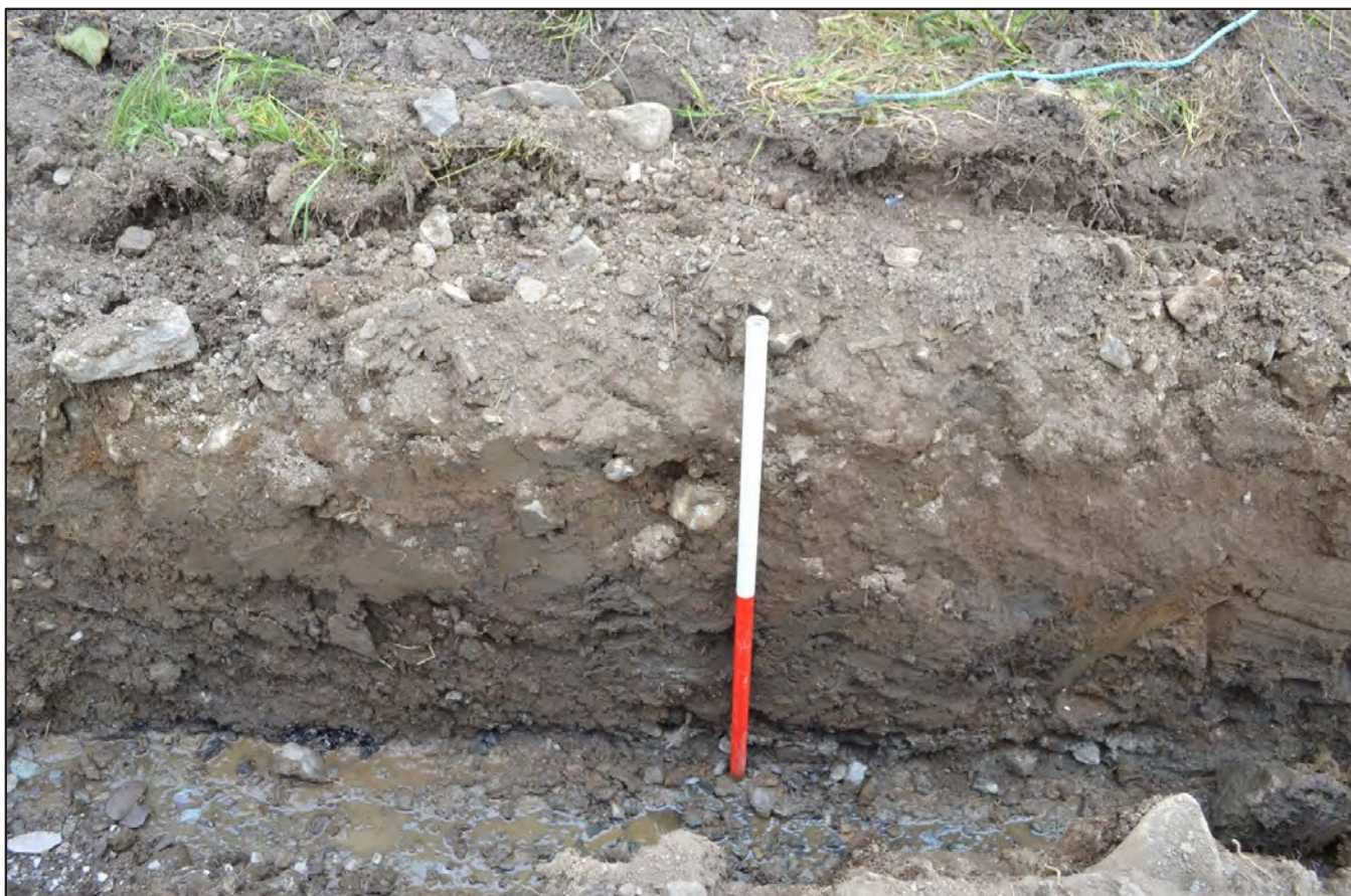
Plate 08: Northern end of section C, showing the pre-existing road indicated by a Tarmacadam layer with crushed slate sub-base layer. View from the W.
