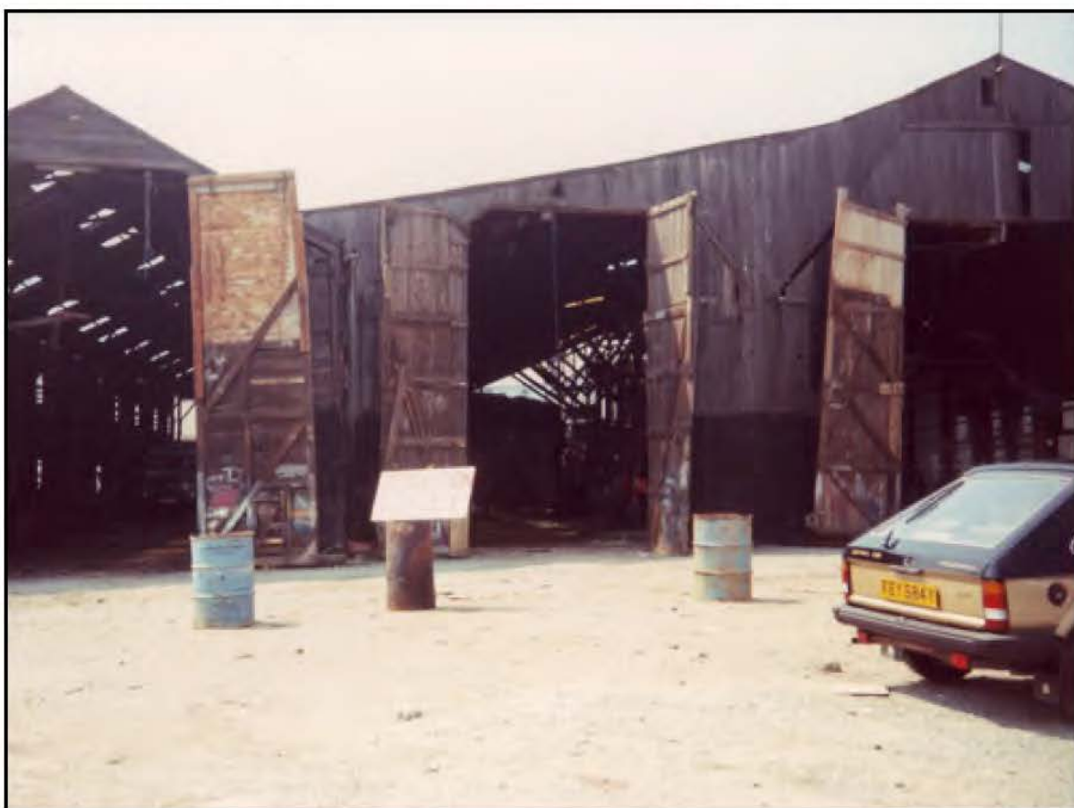
Plate 32 - A reproduction of a photograph taken in 1978 of Dickie's Boatyard prior to the demolition of a boatyard shed. The image is contemporary with Plate 31 and is a view from the south looking the entrance points. Some of the timber framing is visible within the middle entrance and it is also apparent that the shed was expanded in phases as the middle of part of the building appears to have been added to the structures on the left and the right of the image, conjoining them. The boatyard shed is not visible on the 1914 Ordnance Survey map of the area, but is visible in a photograph from the early 1930s (reproduced as Figure 09) and it is likely to have been constructed in the early twentieth century (Source: Bangor Civic Society; ref. BCS00039)
