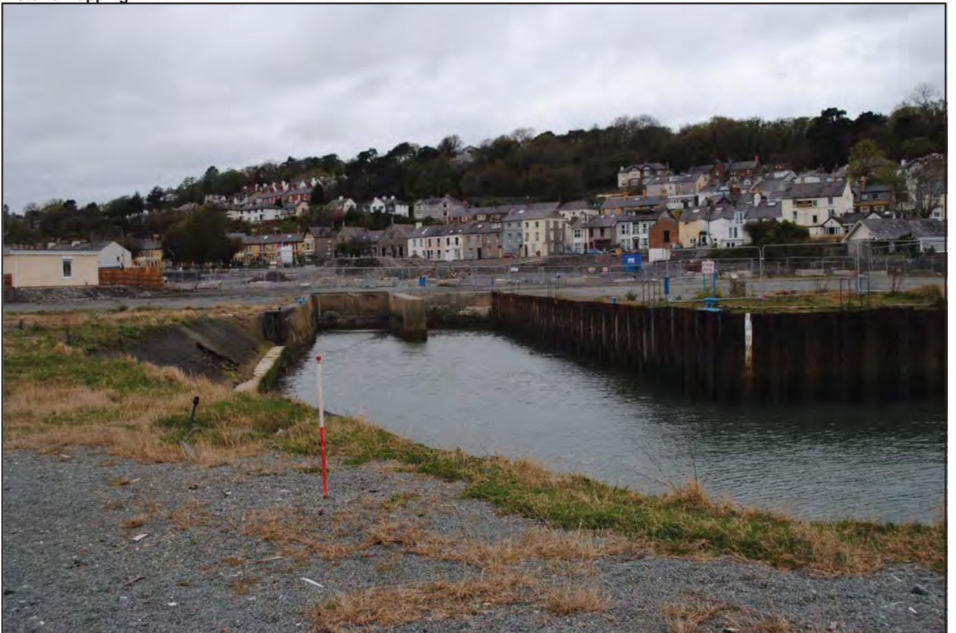
Plate 12 - View southwest detailing boatyard/dock area. Note the concrete built dock in the centre, the sheet piled boatyard to the right and the made ground forming the boatyard on the right. Note: this area is not being developed at this stage but the image indicates the extent of twentieth century development of Dickies' as the jetty/boatyard replaced the existing slipway and "Lewis' Pier" (via the dock and sheet piled yard) that were extant on late nineteenth/early twentieth century historic mapping
