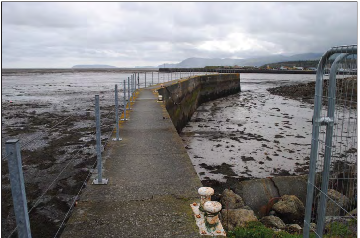
Plate 16 - View along the twentieth century jetty. The jetty is built from concrete; note the moorings in the foreground.
