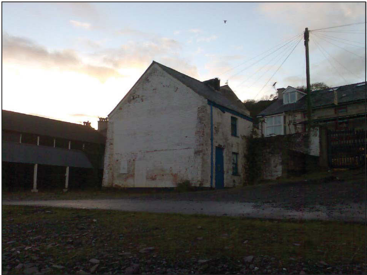
Plate 29 - Rear view of the Dickie's Boatyard structure/former shipbuilding yard structure fronting Garth Road. This structure was demolished in 2011. The historic mapping details a complex grouping of structures at this location (Figures 06 to 08) including the slipway. A buttress has been added to the building, probably after the demolition of an attached structure. A blocked door and window are evident at ground level. Gated access from Garth Road is also visible at the right side of the image. (Source: Watkin Jones Homes)
