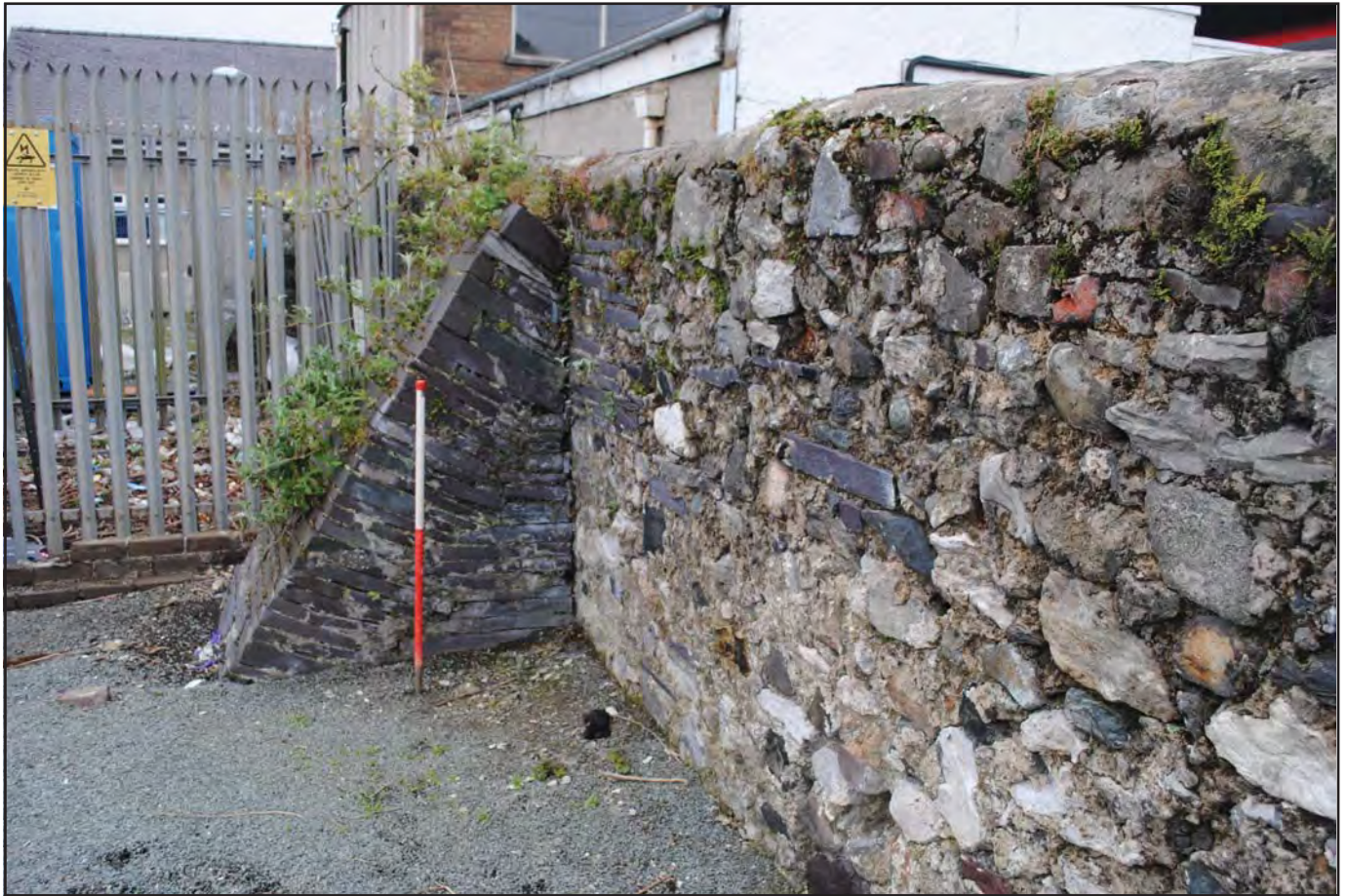
Plate 19 - Detailed view of boundary wall from Plate 18: note the slate buttress. Note: It is currently unclear from client drawing 3811-02 if this will be demolished or rendered.
