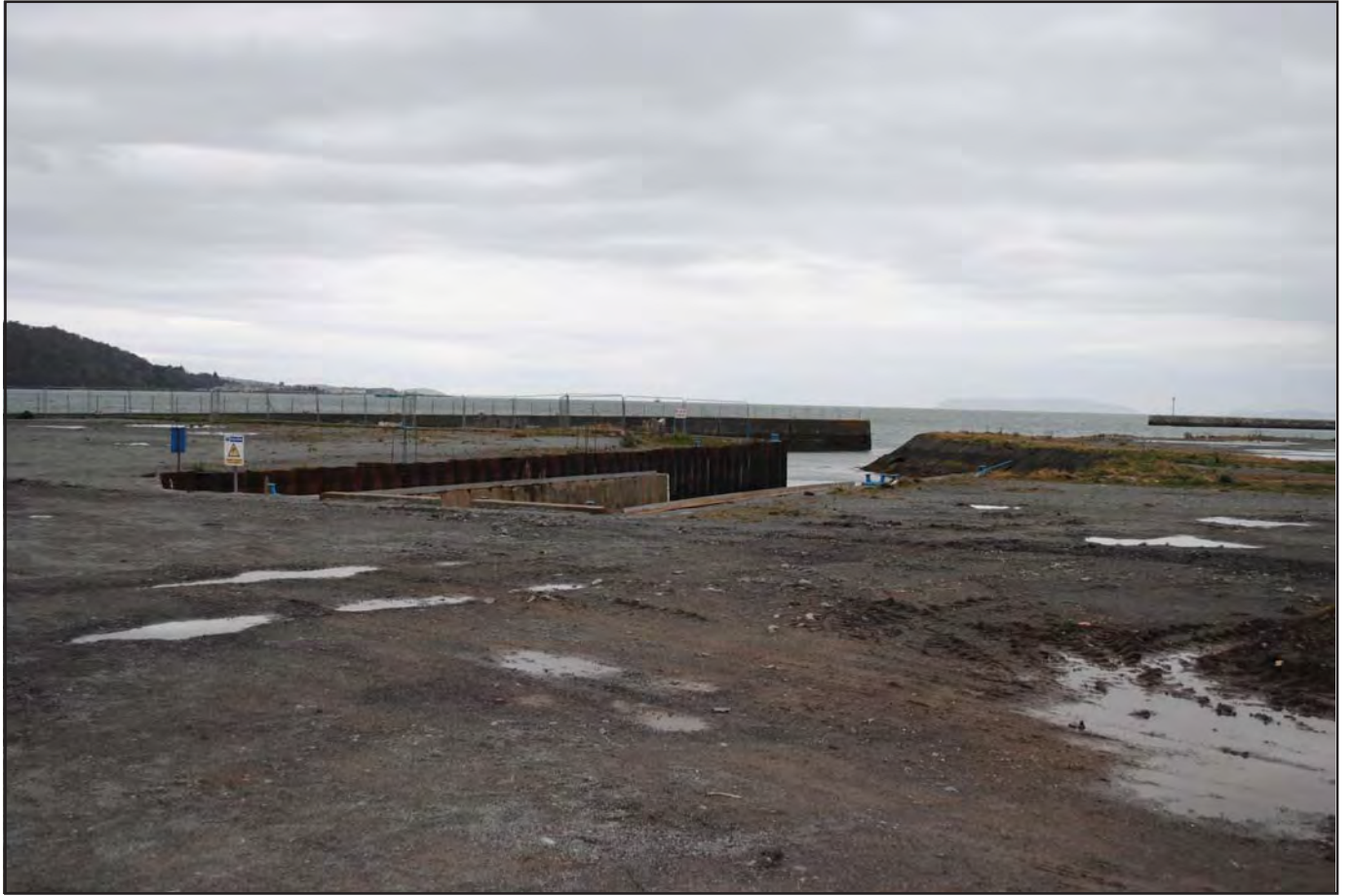
Plate 11 - View northwest detailing jetty/boatyard/dock area. Note the concrete built dock in the centre, the sheet piled boatyard to the left and the made ground forming the boatyard on the right. Note: this area is not being developed at this stage but the image indicates the extent of twentieth century development of Dickies' as the jetty/boatyard replaced the existing slipway and "Lewis' Pier" (via the dock and sheet piled yard) that were extant on late nineteenth/early twentieth century historic mapping
