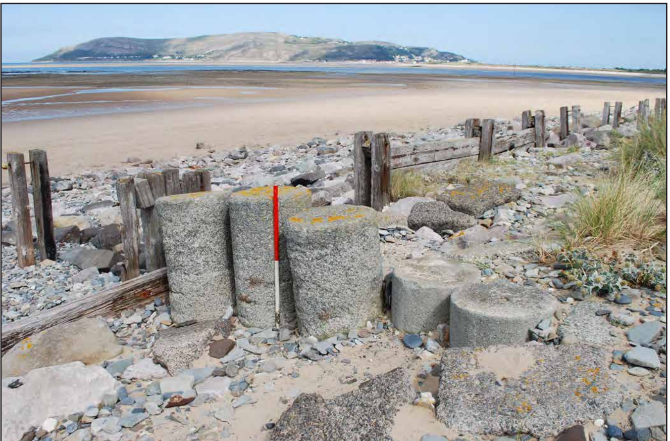
Plate 35: Possible anti-tank columns re-used for erosion control, Morfa Conwy.
