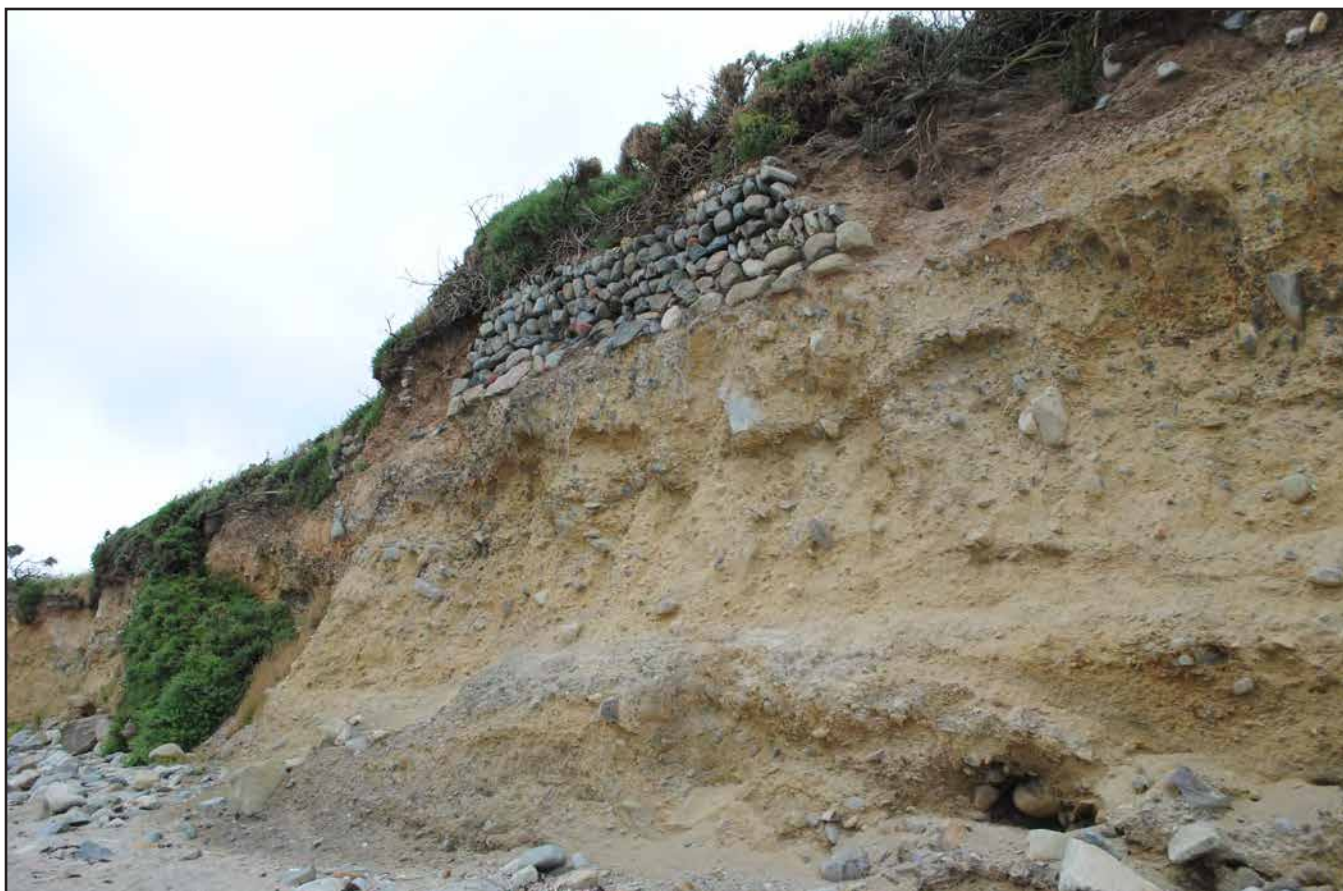
Plate 27: Clawdd boundary eroding from cliff at Criccieth
