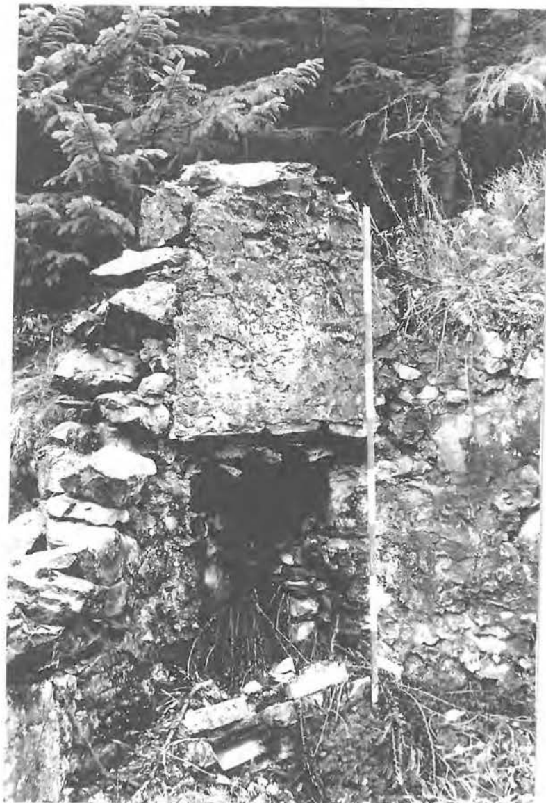
Plate 9. The hearth and flue in the cottage annexe
