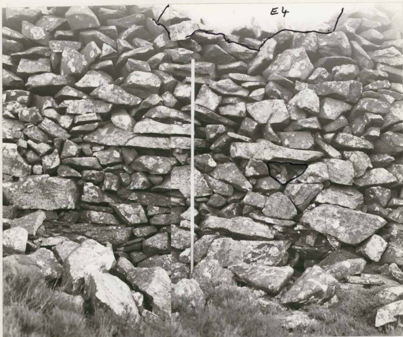
Plate 80. Collapse E4 before conservation, looking SE (G1022/014/12-13).
