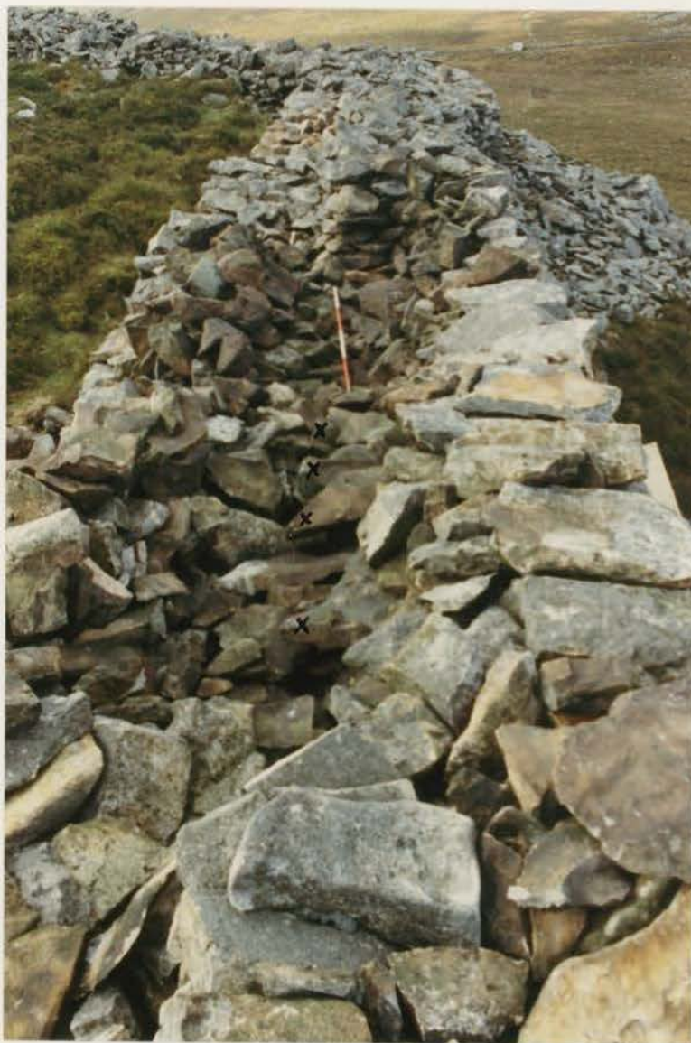
Plate 56. Collapse D10 after clearance of tumble/unstable masonry, looking SW (G1022/116/23).
