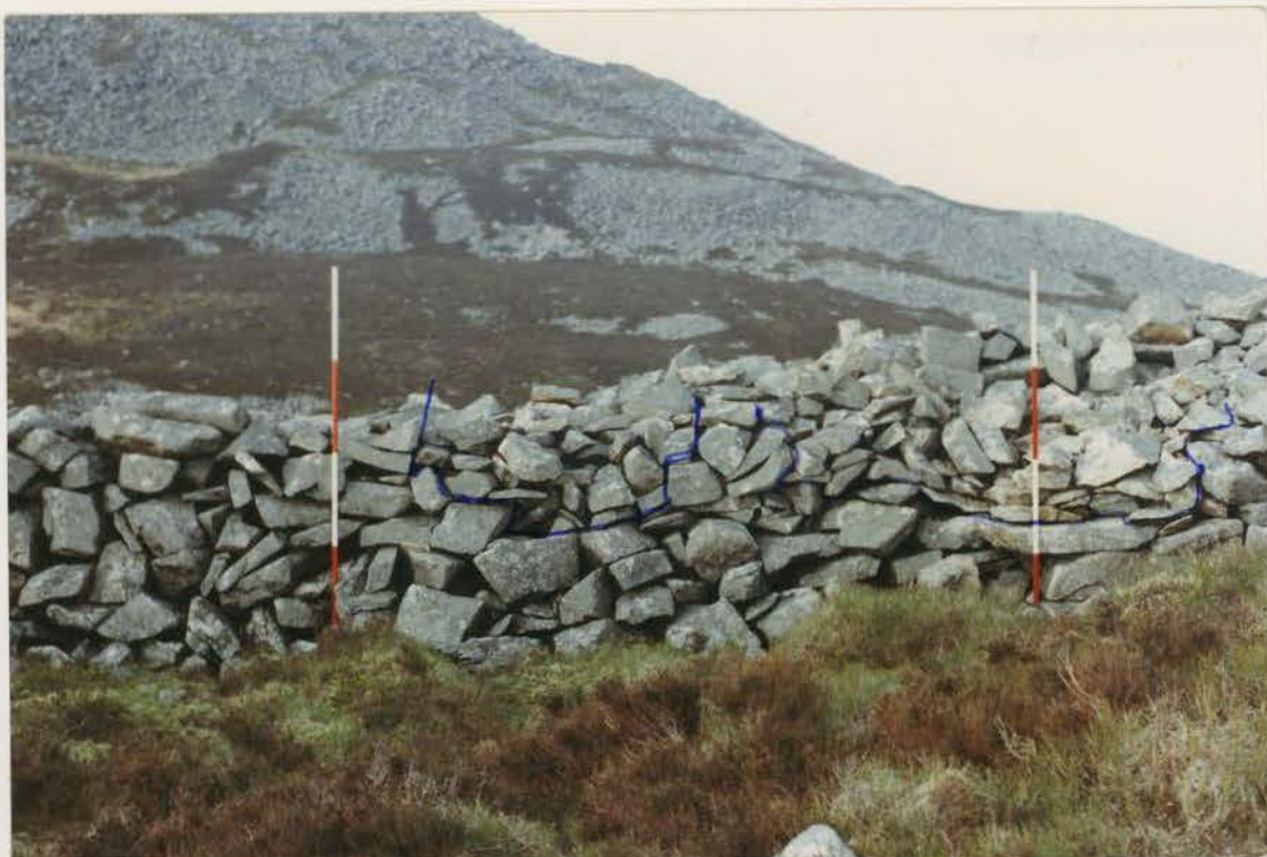
Plate 44. Collapses D4 & D5 before conservation, looking NW. The blocked entrance visible on the outer face would have entered the fort between the two scales. (G1022/104/20).
