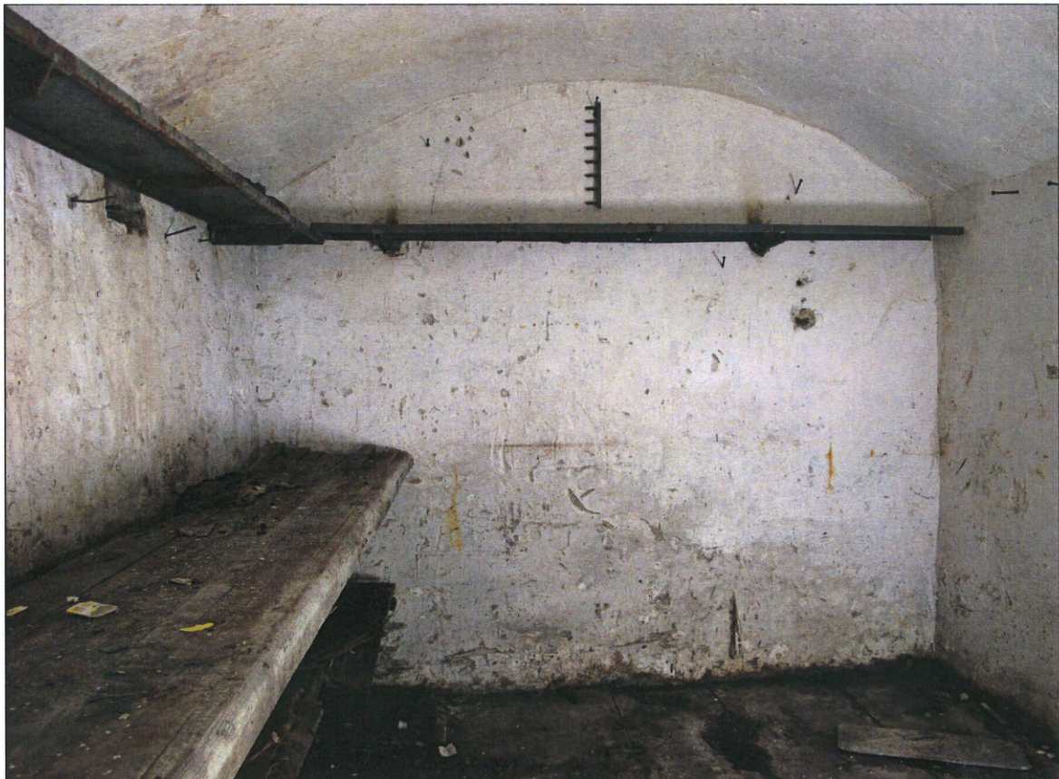
The smaller of the two vaulted cellars in the north-eastern rooms
