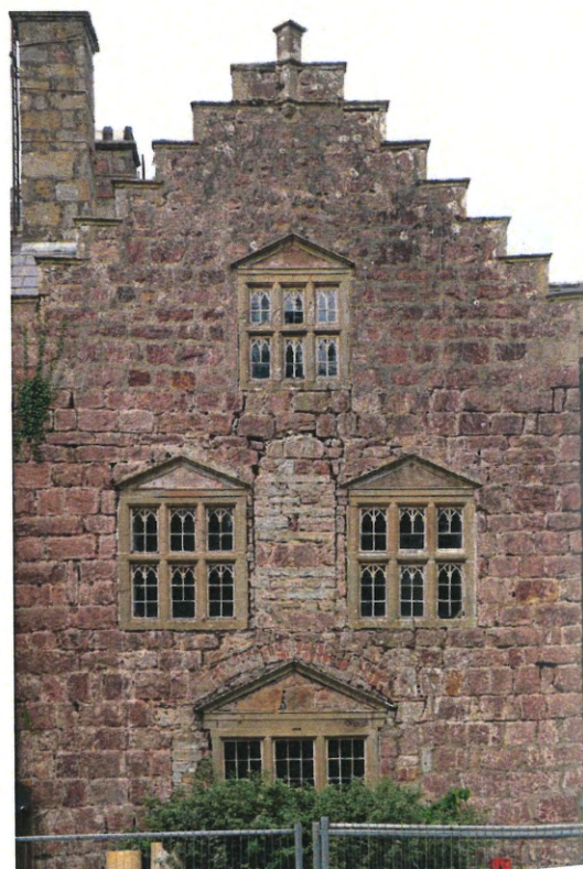
The southern gable of the main house
