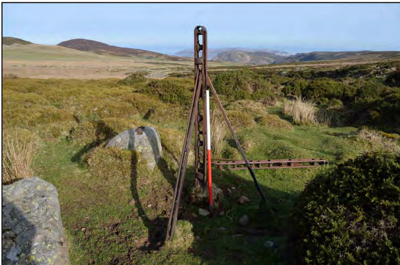
Plate 13: Mechanism for control of sluice gate; scale 1x1m (archive reference: G2594_041)
