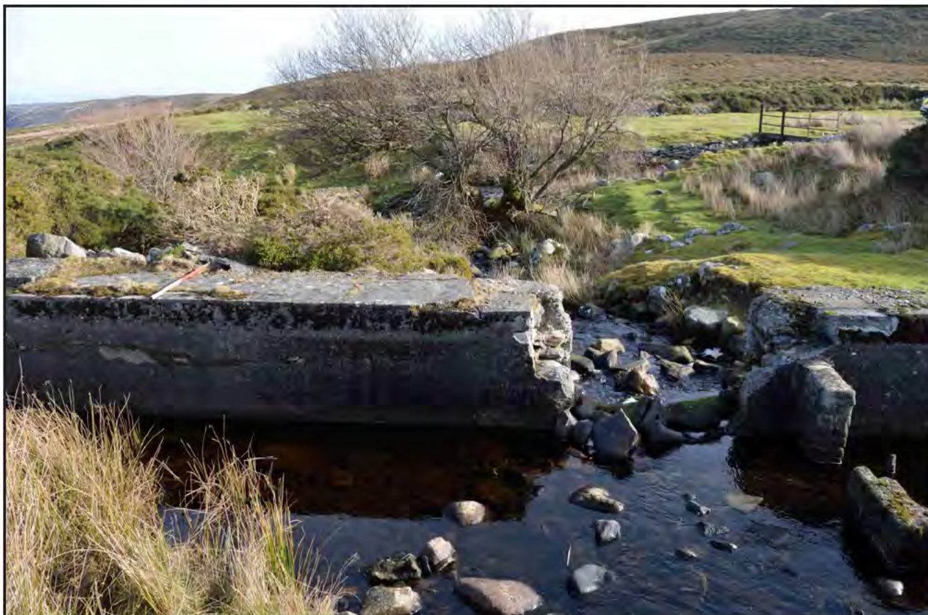
Plate 11: Gate missing in sluice; scale 1x1m (archive reference: G2594_043)
