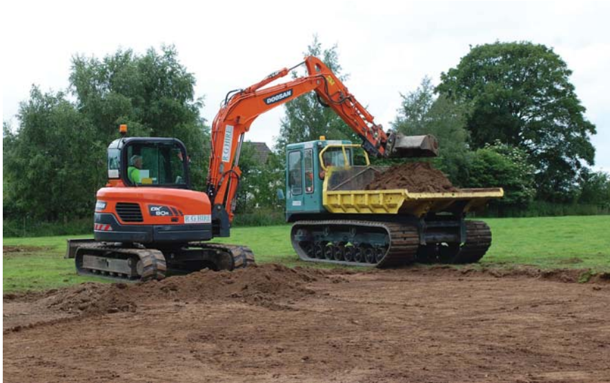
Plate 2. Use of a dumper to move spoil efficiently
