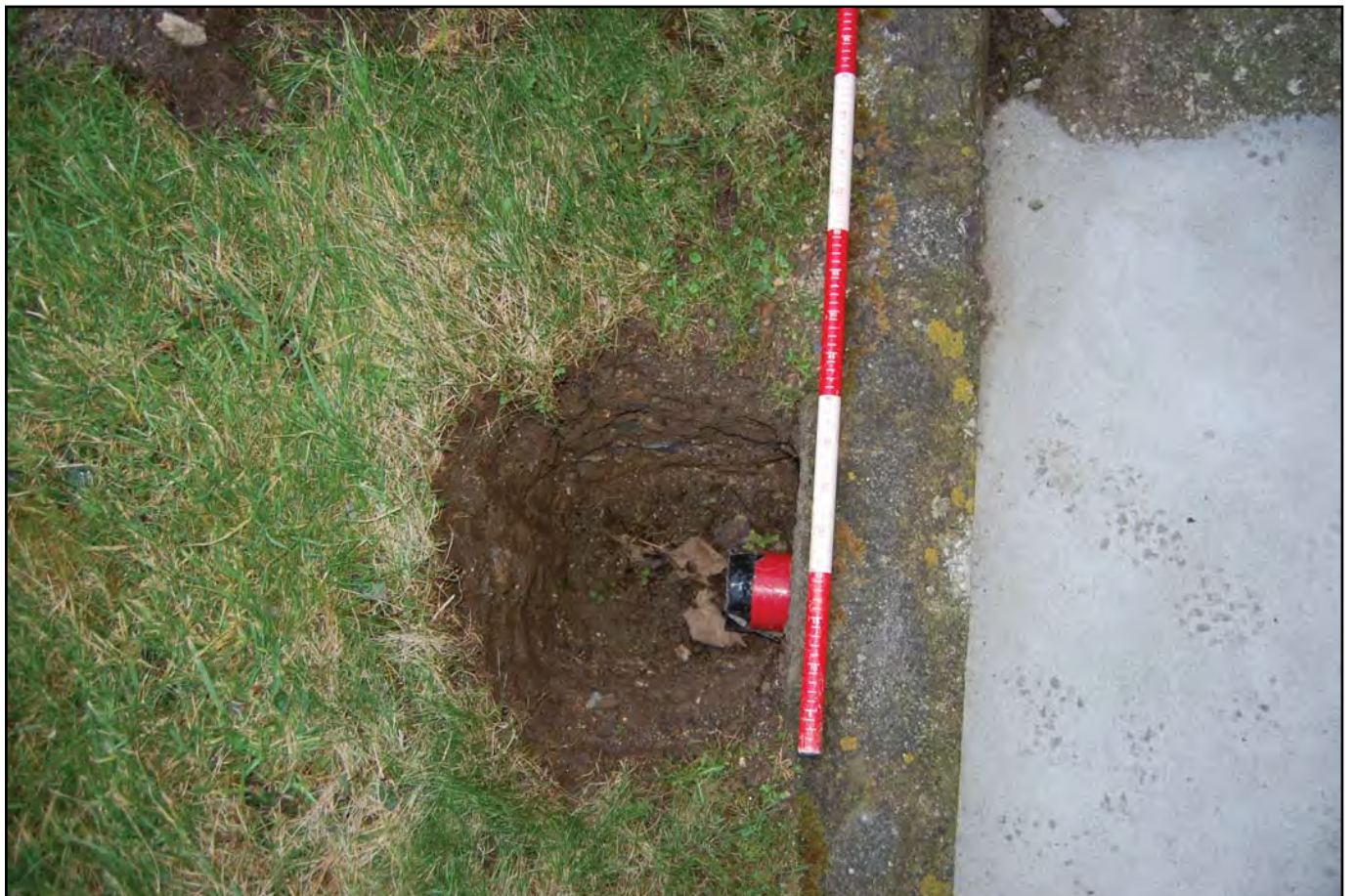
Plate 02 - TP01 as excavated by Derwen Llŷn Ltd. Electrical cable ducting visible in bottom of pit.
