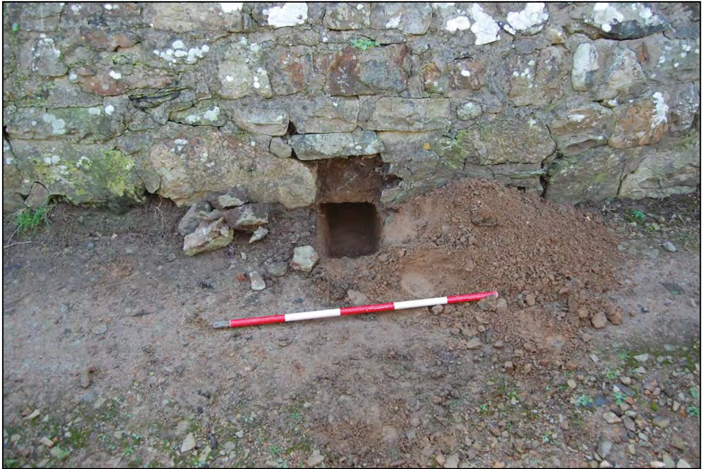
Plate 09 - View south of external face of north wall of the churchyard - the exit of the electrical cable ducting is visible as the slot in the centre of the image.
