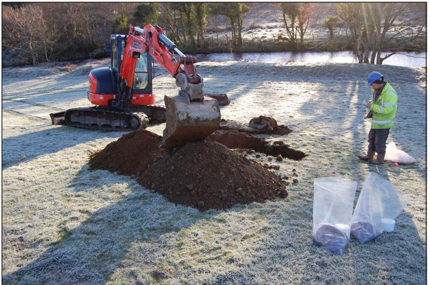
Plate 16 - Excavation of TPD 11 below natural as part of Ground Investigation
