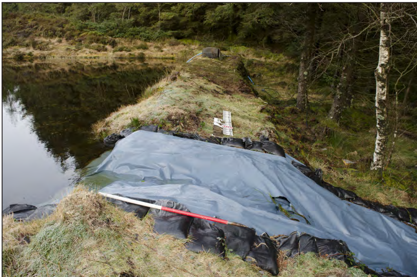
Plate 05: Old sluice through Embankment D - plastic sheeting and sandbags; scale: 1x1m (archive reference: G2674_005).
