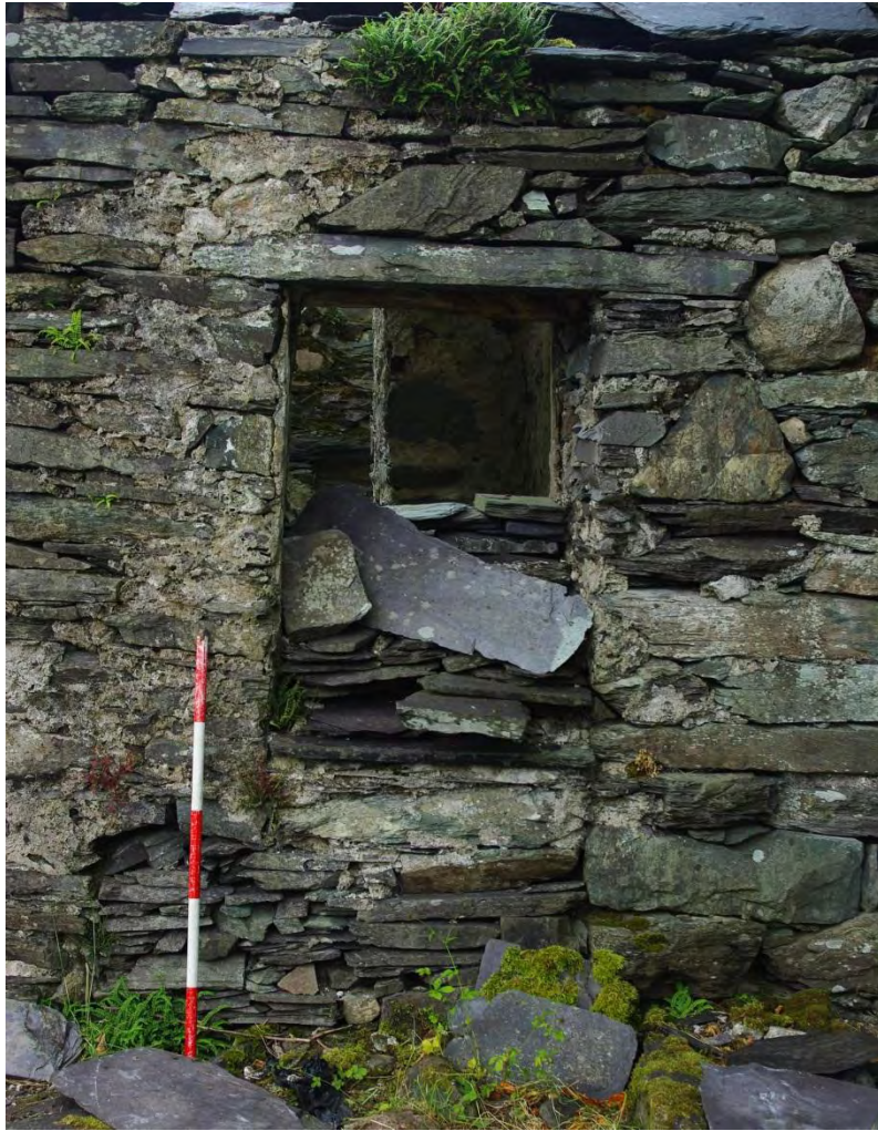
Figure 23. Remains of phase I doorway 2011 in ENE wall. Note straight joint below window
