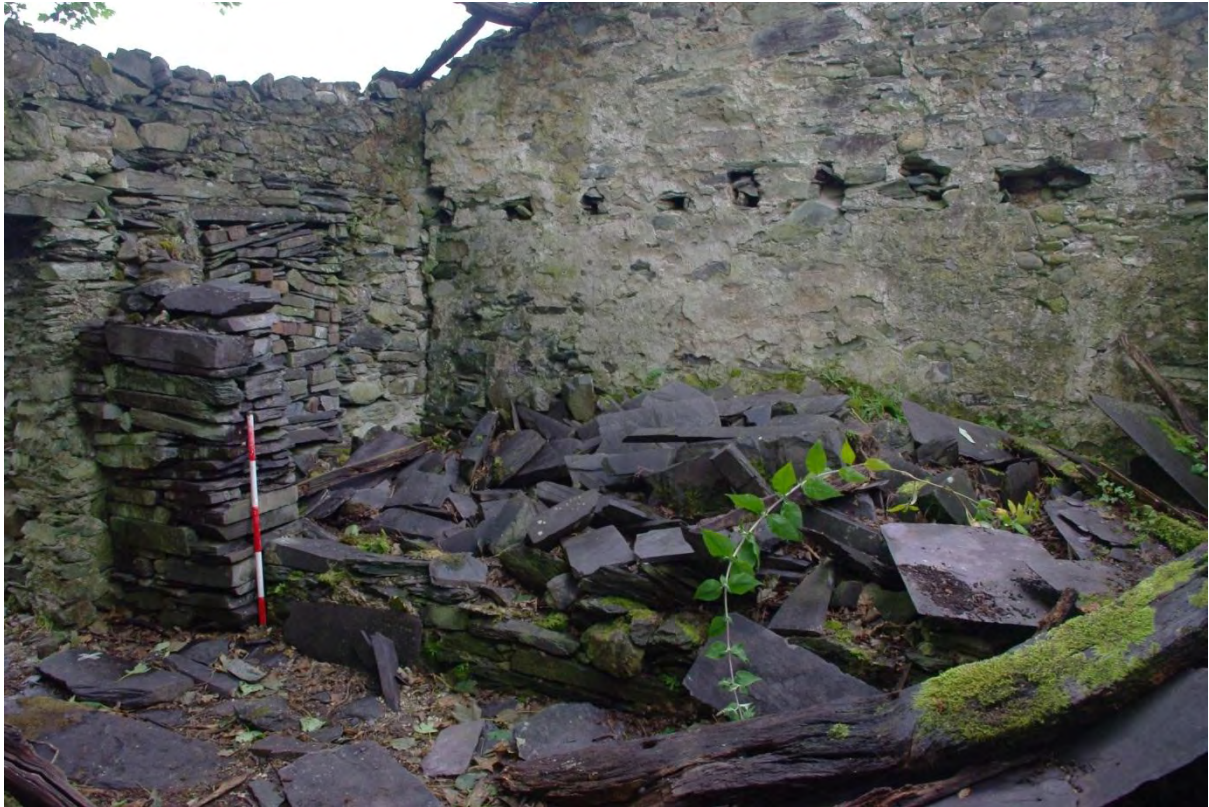
Figure 18. Collapsed dividing wall 1015. Note sockets for crog-loft joists
