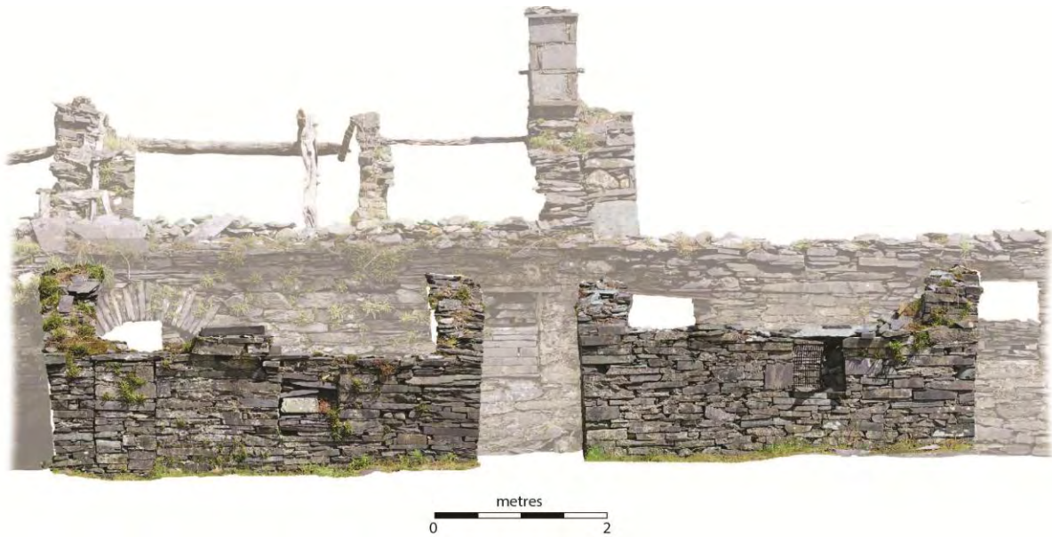
Figure 11. Orthographic projection from 3d model – WSW facing elevation of extensions
