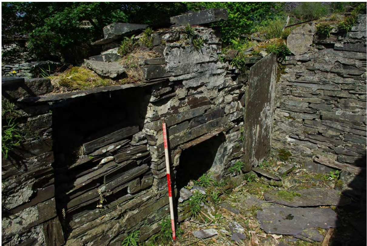
Figure 27. WSW wall of extension 2006 showing fireplace 2006 window 2002 and blocked door 2001
