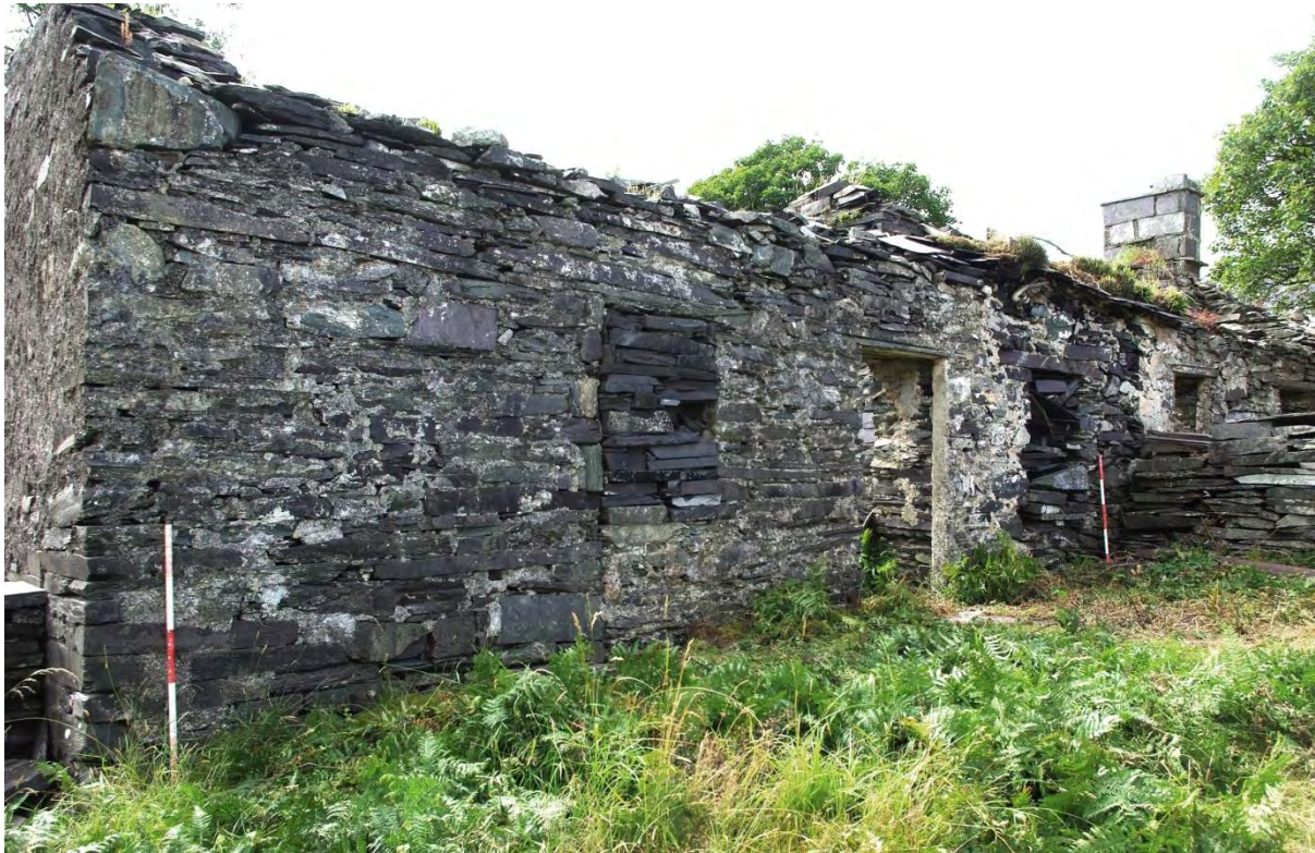
Figure 40. ENE wall of cottage (4009) showing straight joint beneath window 4008
