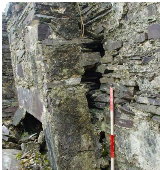
Figure 43. Fireplace 4018 showing collapse
