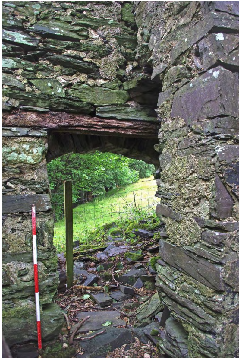
Figure 15. Blocked doorway 1005 showing oak lintel and corner of fireplace
