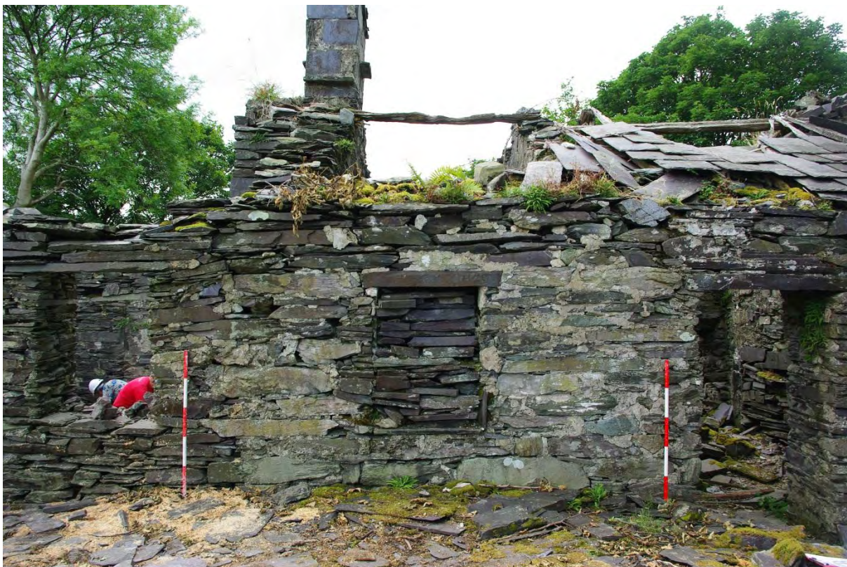
Figure 30. ENE wall of cottages 2 and 3 showing change from field-stone masonry to slate (at L scale)
