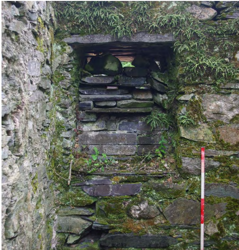
Figure 20. Partly blocked window 2003
