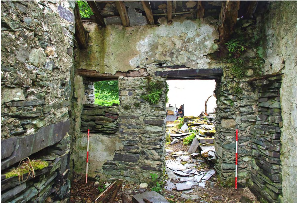
Figure 24. Interior of ENE wall of cottage showing blocked phase I doorway and oak lintel
