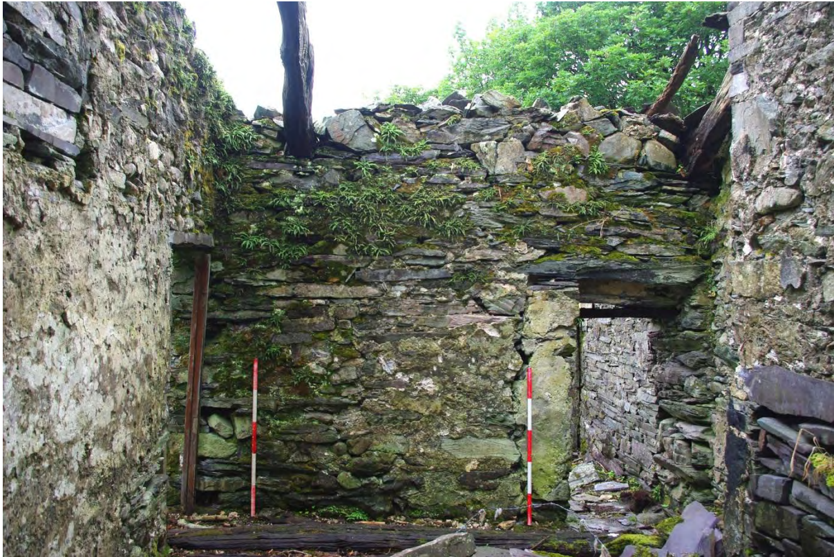
Figure 22. Inside of arched doorway 2007 showing blocking 2008 and slate lintel
