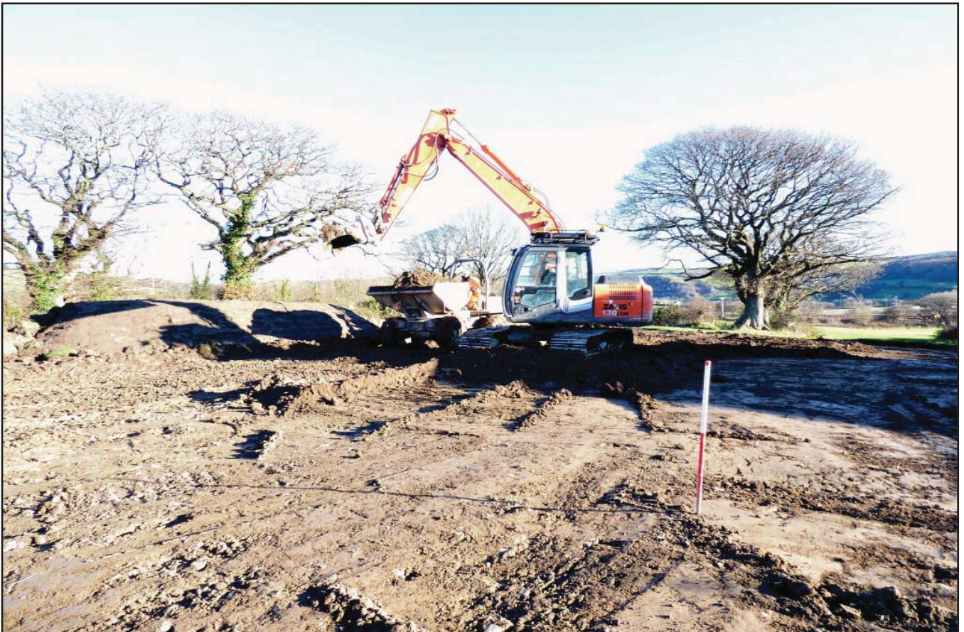
Plate 02: Topsoil strip in Build Phase A, with 360° excavator and dumper. View from the north. 1 x 1m scale.
