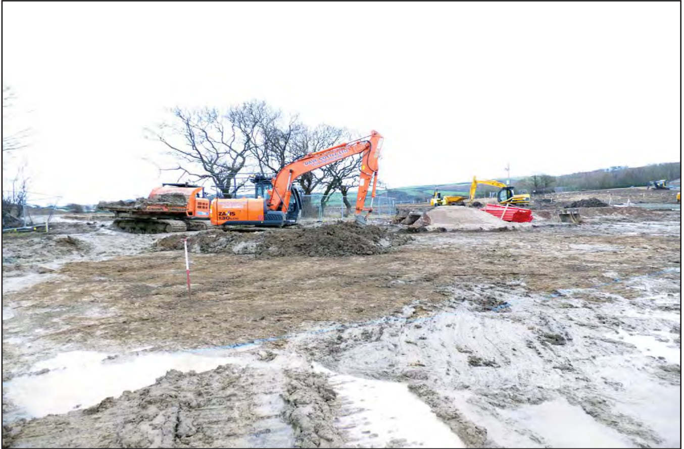
Plate 05: Tracked dumper being used for the saturated ground conditions. 1m x 1m scale. View from the north west (Photographic archive ref. G2374_Esgyryn_0158.jpg).
