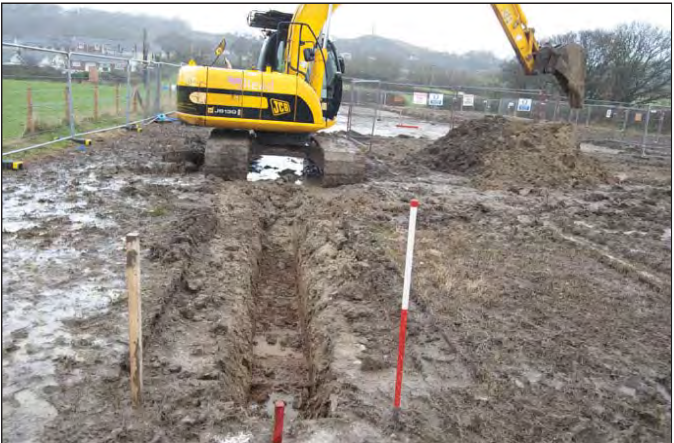
Plate 16: Excavation of duct trench adjacent to main car park. 1m x 1m scale. View from the south (Photographic archive ref. G2374_Esgyryn_0144.jpg).
