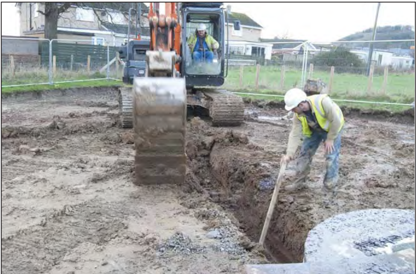
Plate 14: Excavation of drainage pipe trench at hammerhead. View from the south east (Photographic archive ref. G2374_Esgyryn_0140.jpg).
