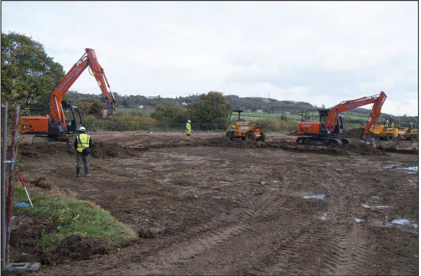
Plate 02: Topsoil strip of sports pitch with 360° excavators & 3 wheeled dumpers. View from the west (Photographic archive ref. G2374_Esgyryn_0116.jpg).
