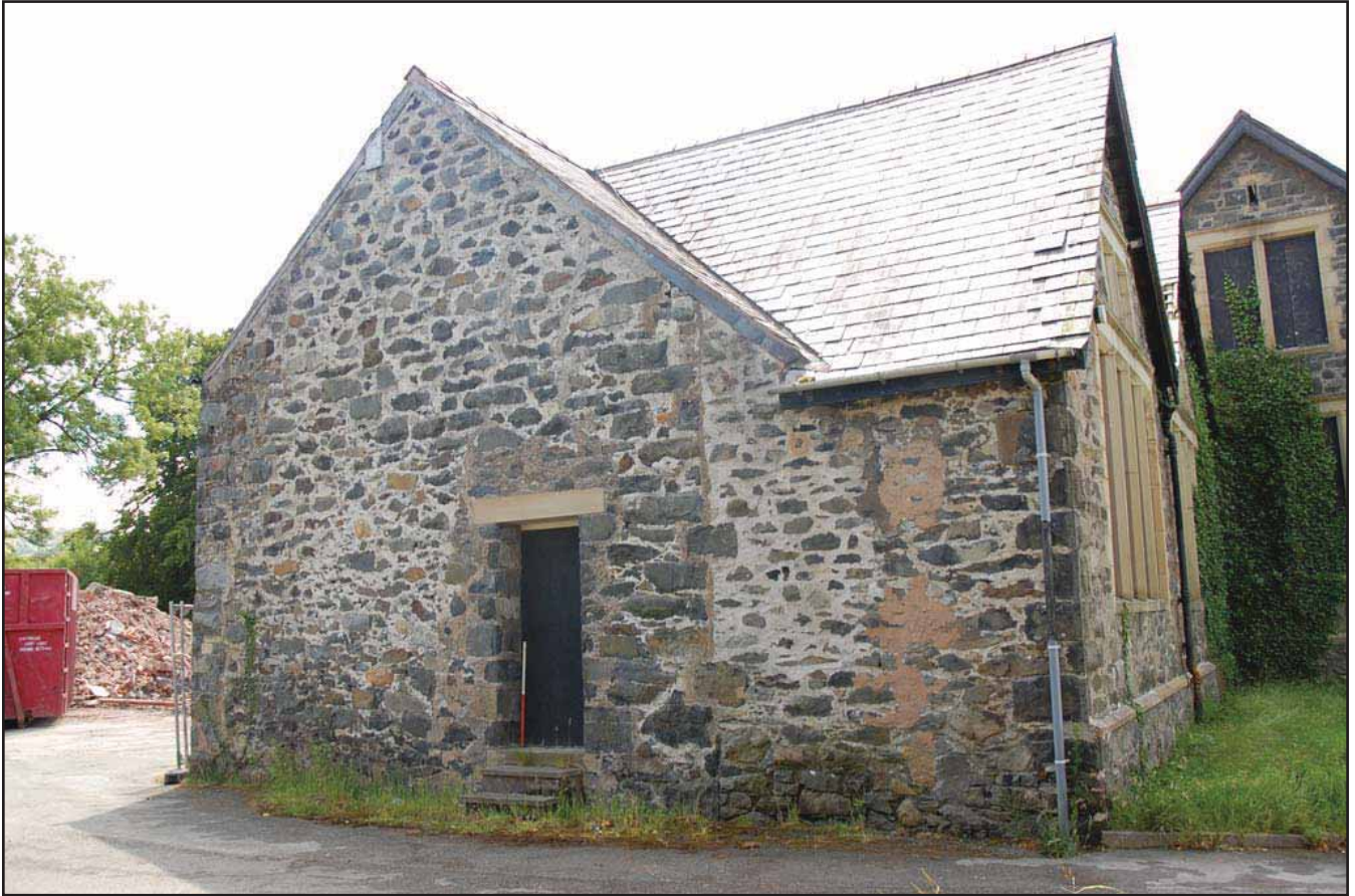
Plate 79 - Extension B (Old Grammar School Block) - north facing elevation; note structural phasing to the left of the door. Scale: 1.0m
