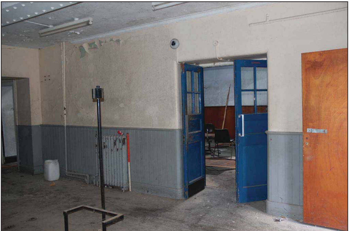
Plate 83 - Extension A (Old Grammar School Block) - Room G01 view east; note cloakroom furniture and ceiling support joist. The double door entrance provides access to the Old Grammar School Hall. Scale: 1.0m
