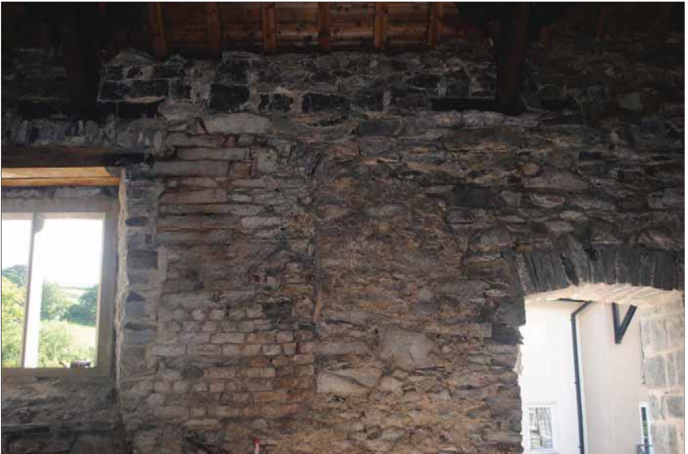
Plate 140 - Old Grammar School internal - Blocked Window on on the West Facing Internal Elevation with Brick Infill
