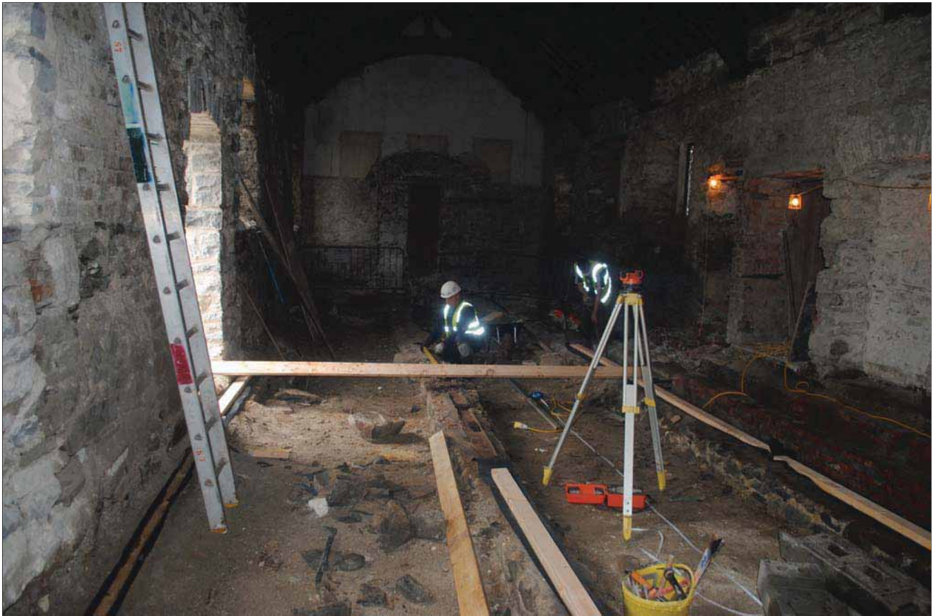
Plate 148 - Old Grammar School internal - View of the School Hall looking north during renovations, showing the sleeper walls beneath the hall floor
