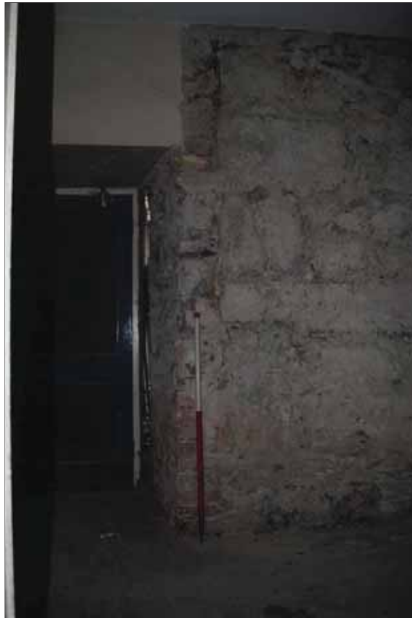
Plate 146 - Old Grammar School internalView of the Formerly External Quoin Stones at the South West Corner of the School Hall, with adjacent Modern Brickwork. Scale 1m
