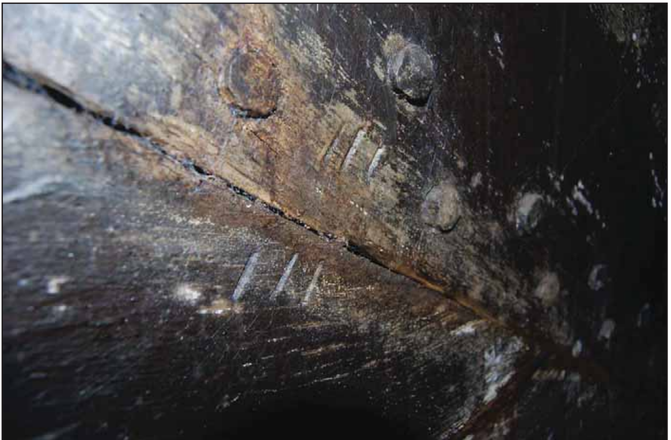
Plate 131 - Old Grammar School internal - detail of carpenter's markings on roof truss 02
