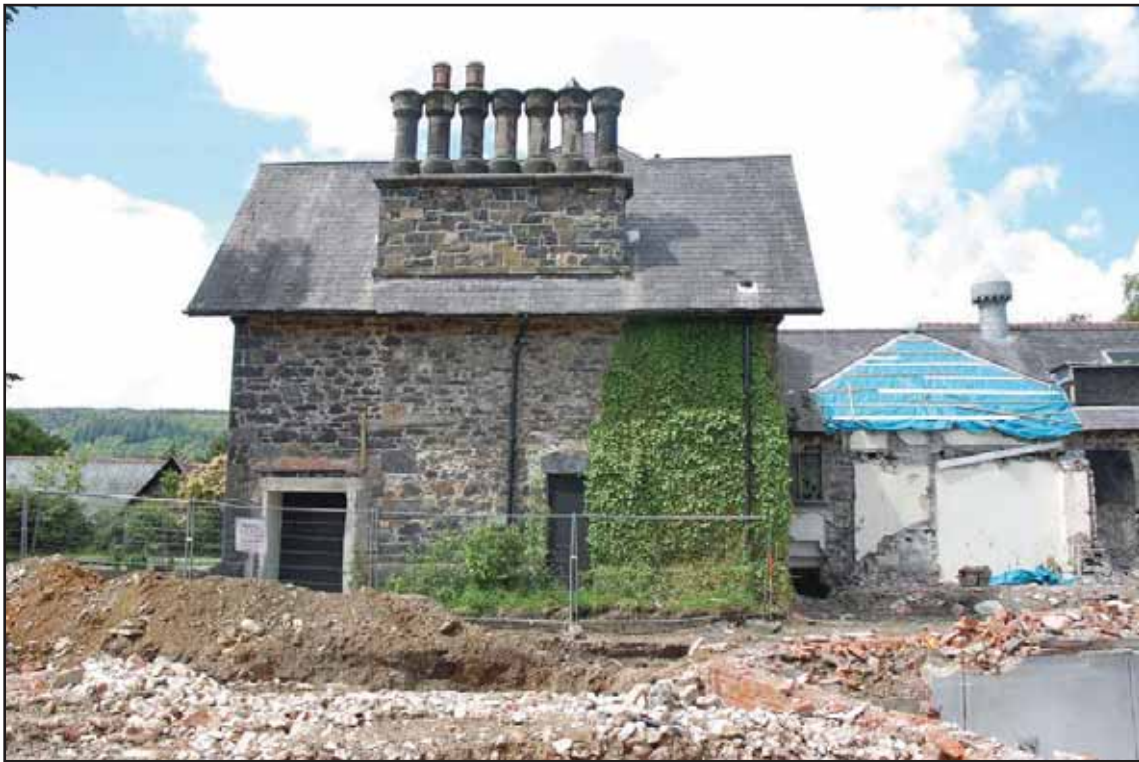
Plate 98 - Headmaster's Building - east elevation. The former link corridor entrance is at the left of image. Note the former building exterior next to the link corridor entrance that was replaced by the projecting gable. Scale: 1.0m
