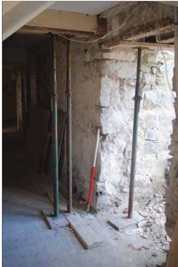
Plate 144 - Old Grammar School internal- View of the Formerly External Quoin Stones at the South East Corner of the School Hall. Scale 1m
