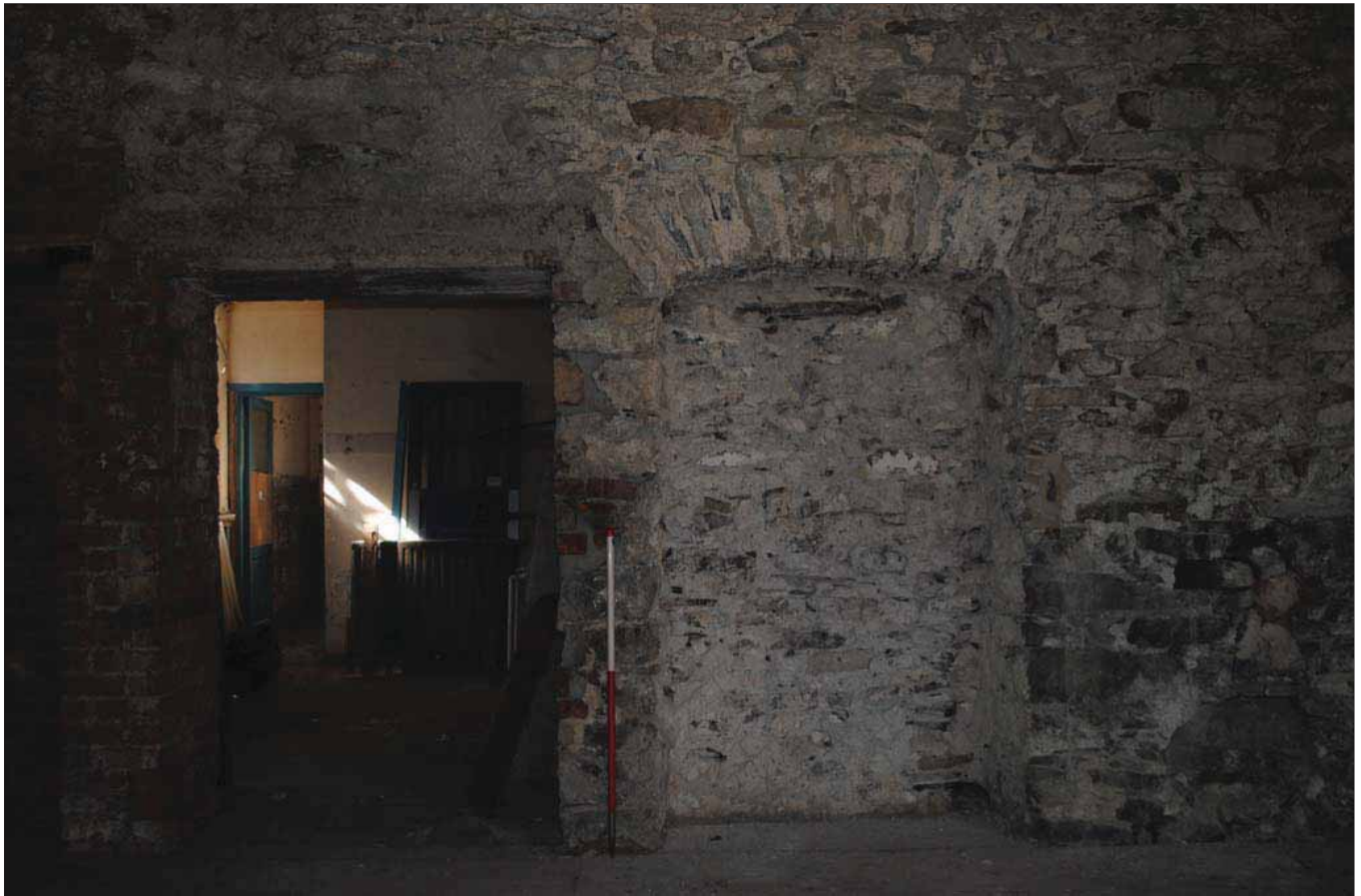
Plate 138 - Old Grammar School internal - Blocked Cross-Passage Door on the East Facing Internal Elevation. Scale 1m
