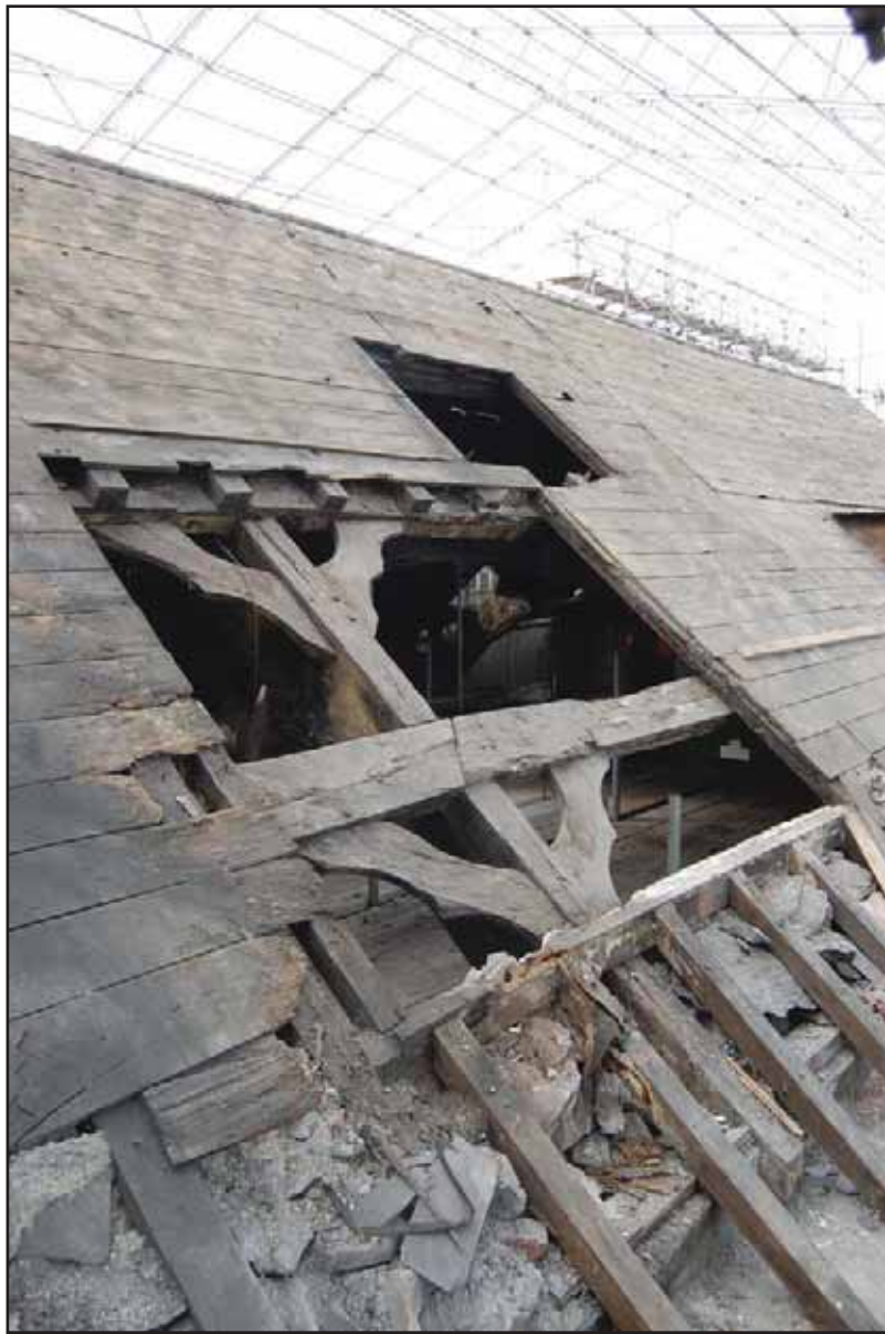
Plate 122 - Old Grammar School External - view east of roof during renovation: wind brace and purlin detail
