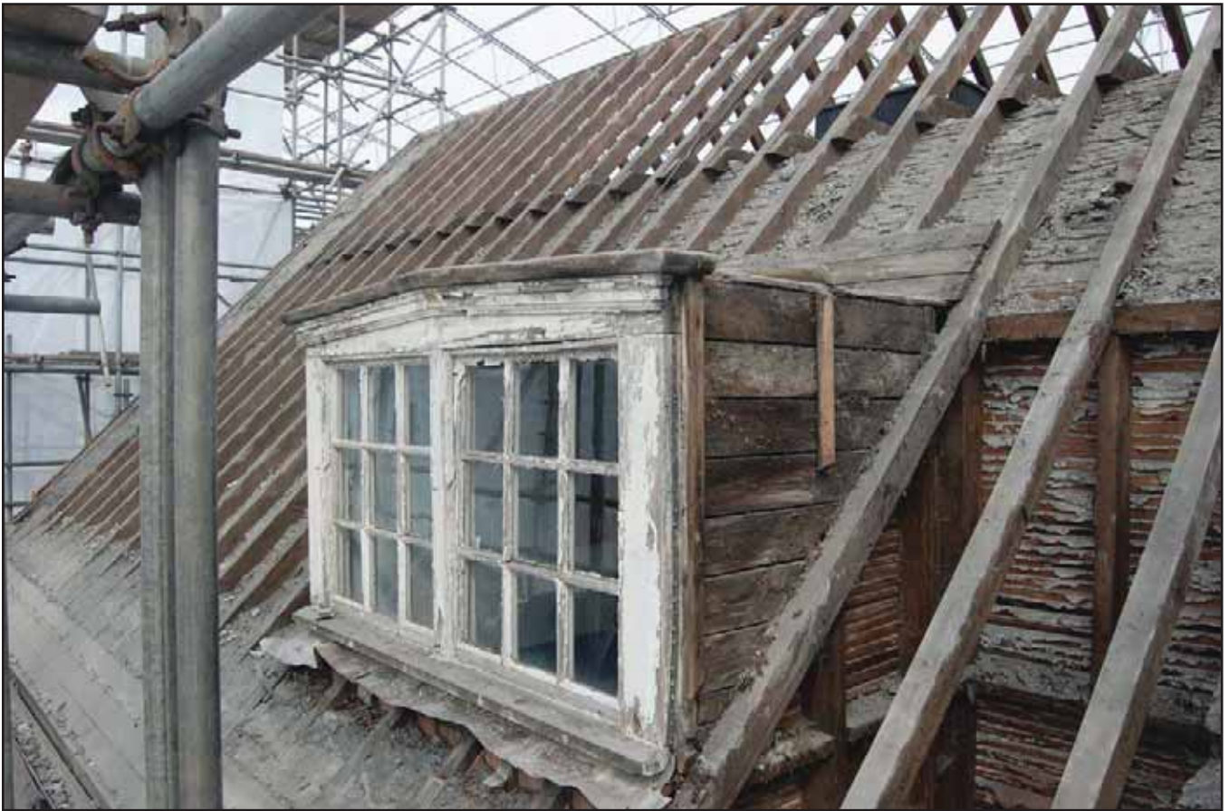
Plate 120 - Old Grammar School External- view west of roof during renovation: dormer light detail
