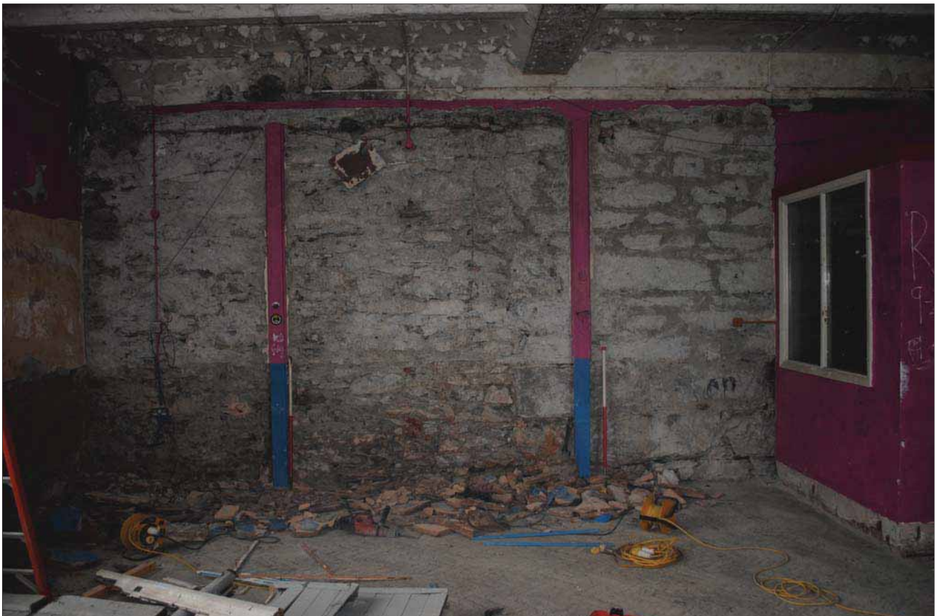
Plate 147 - External View of North West Corner of the School Hall, taken from Extension A room G02 showing interface between the corner quoins and the later school passage constructed of smaller rubble masonry. Scales 1m
