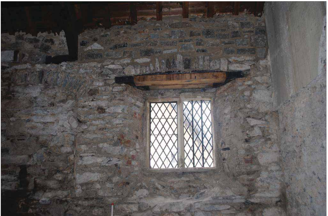
Plate 139 - Old Grammar School internal - Detail of blocked window and renewed window with modern lintel at the Southern End of the West Facing Internal Elevation
