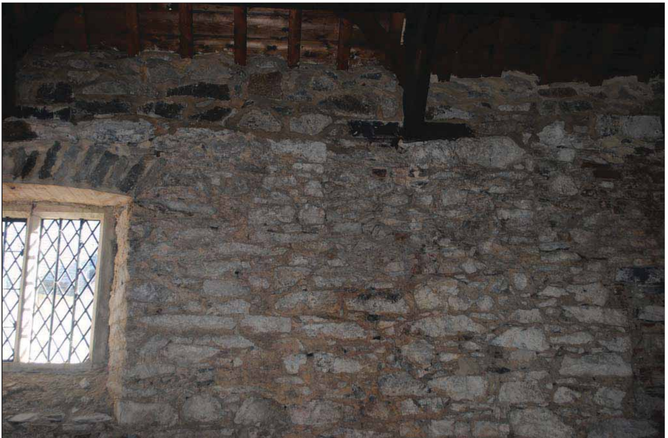
Plate 143 - Old Grammar School internal - Detail showing modern work on the West Facing Internal Elevation at wall plate level
