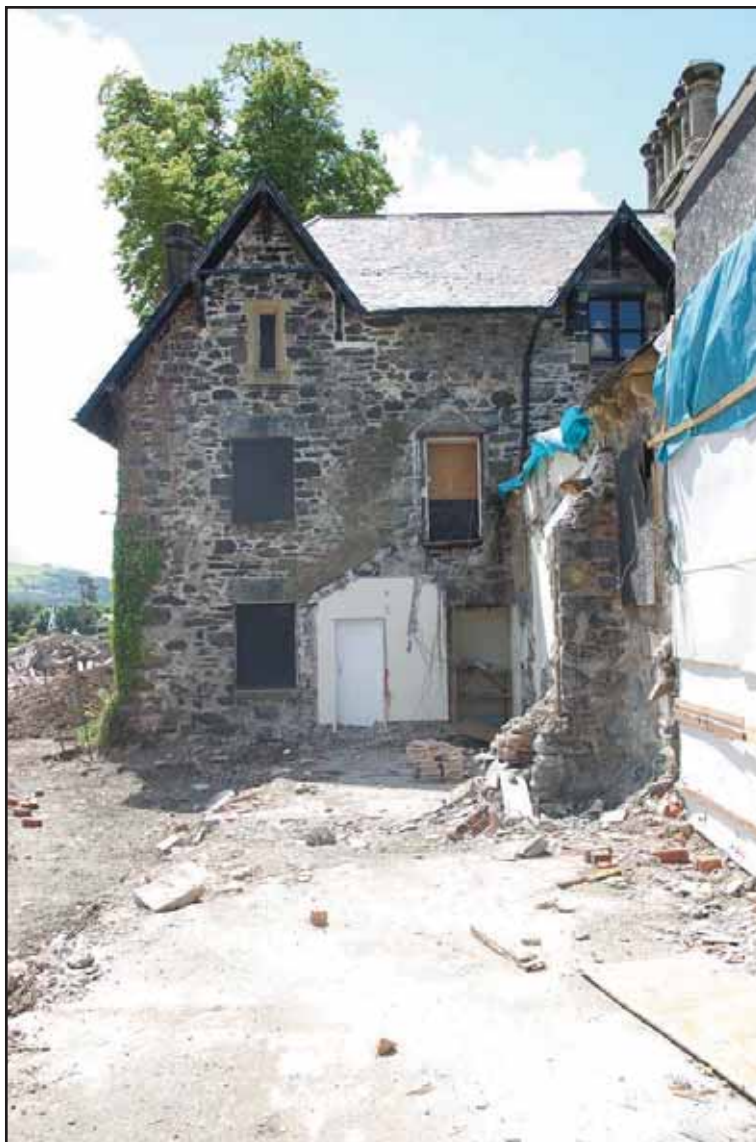
Plate 99 - Headmaster's Building - north elevation east side. Note the former building extension which was demolished in 2008 and the first floor window converted into a door. Scale: 1.0m
