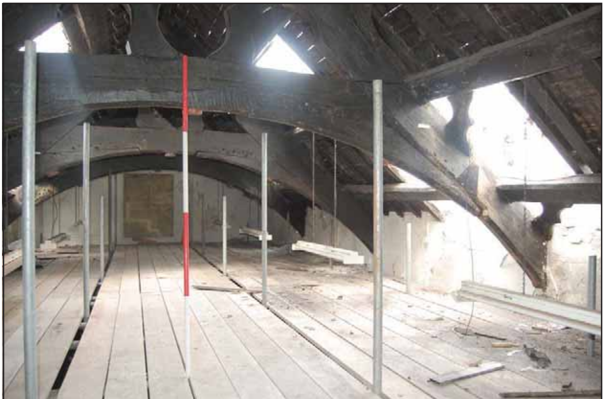
Plate 123 - Old Grammar School internal- view north of roof trusses during renovation. Scale: 2.0m
