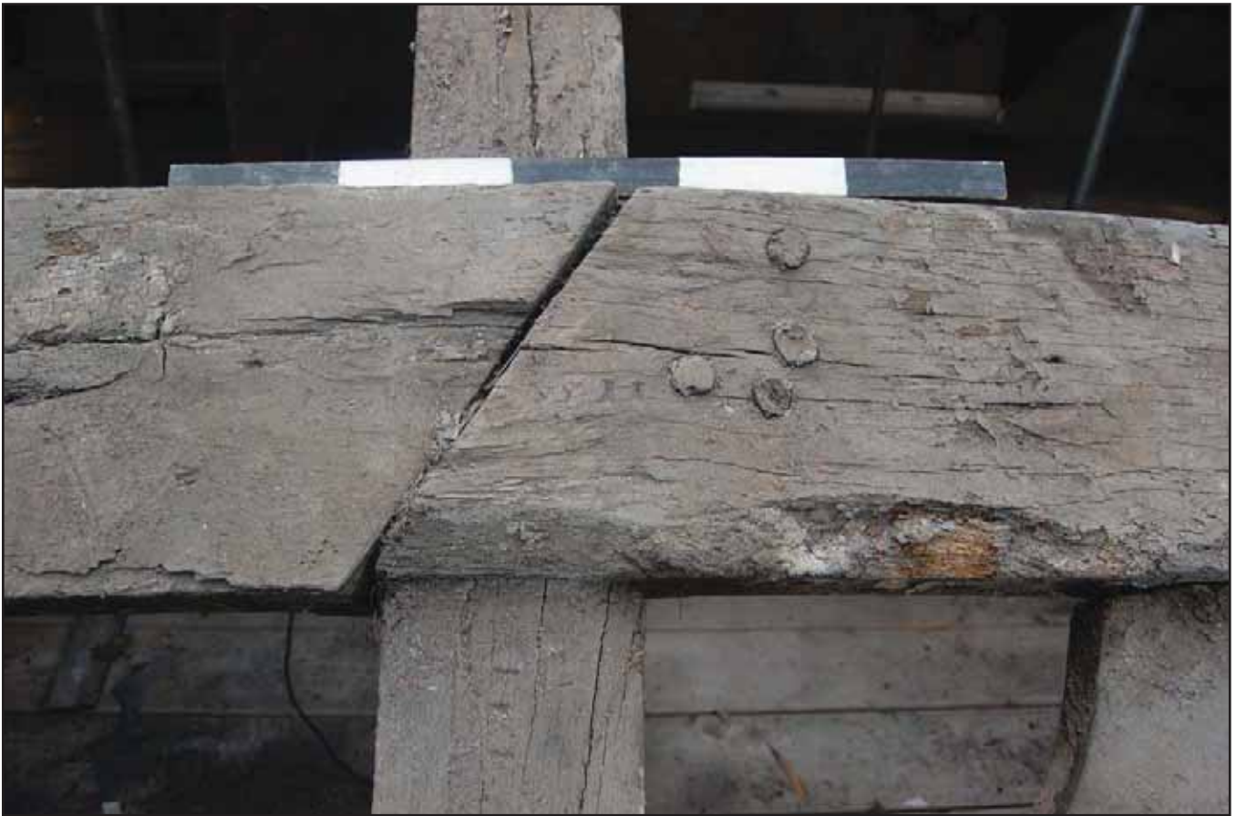
Plate 128 - Old Grammar School internal - detail of join between purlins and associated fixings. Scale: 0.3m
