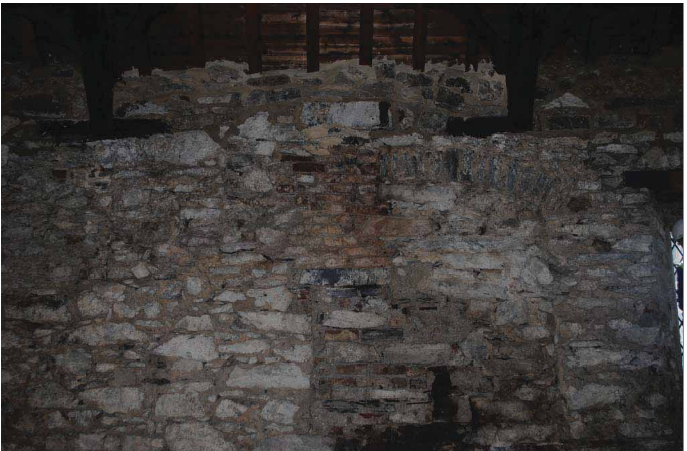
Plate 141 - Old Grammar School internal - Detail of blocked window on the West Facing Internal Elevation, with later brick infill
