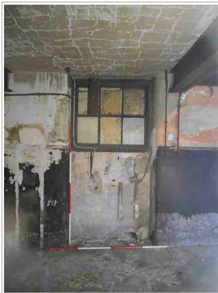
Plate 133. Remains of early door, subsequently transformed into a window which is currently blocked. Eastern facing interior wall.
