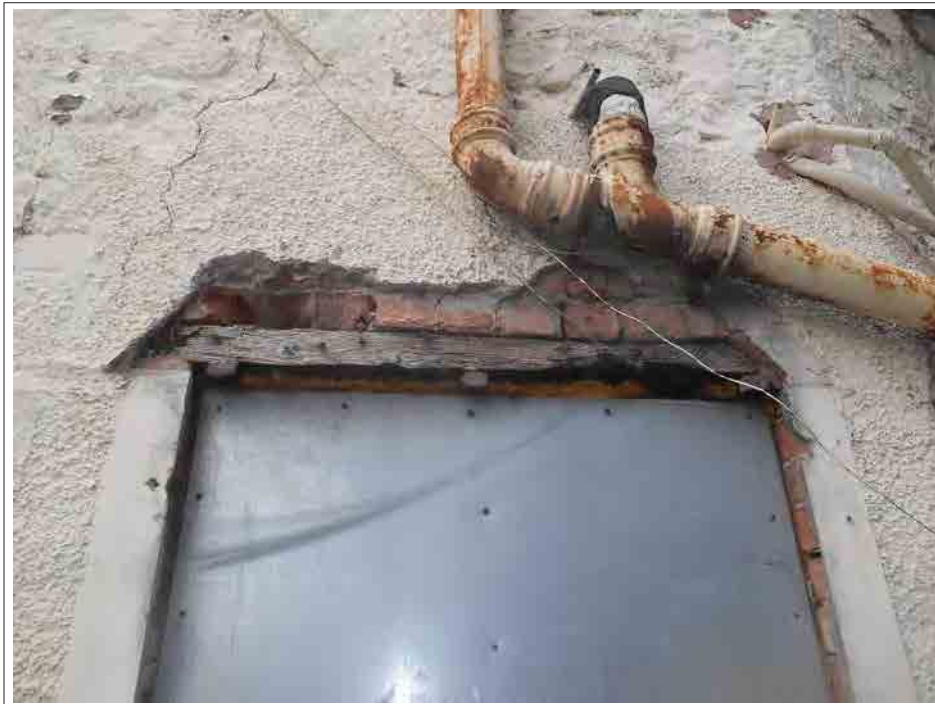
Plate 158. Detail of wooden lintel.
