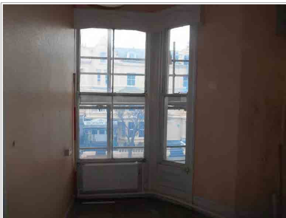
Plate 68. View of Room 8. Storeyed canted three-light window blocked by wall addition, looking N.
