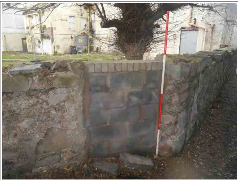
Plate 172. Modern alteration of circuit wall. Scale 2m
