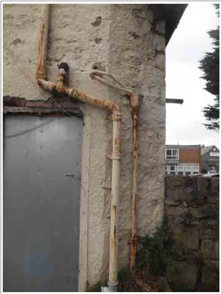
Plate 156. View of cast iron guttering.
