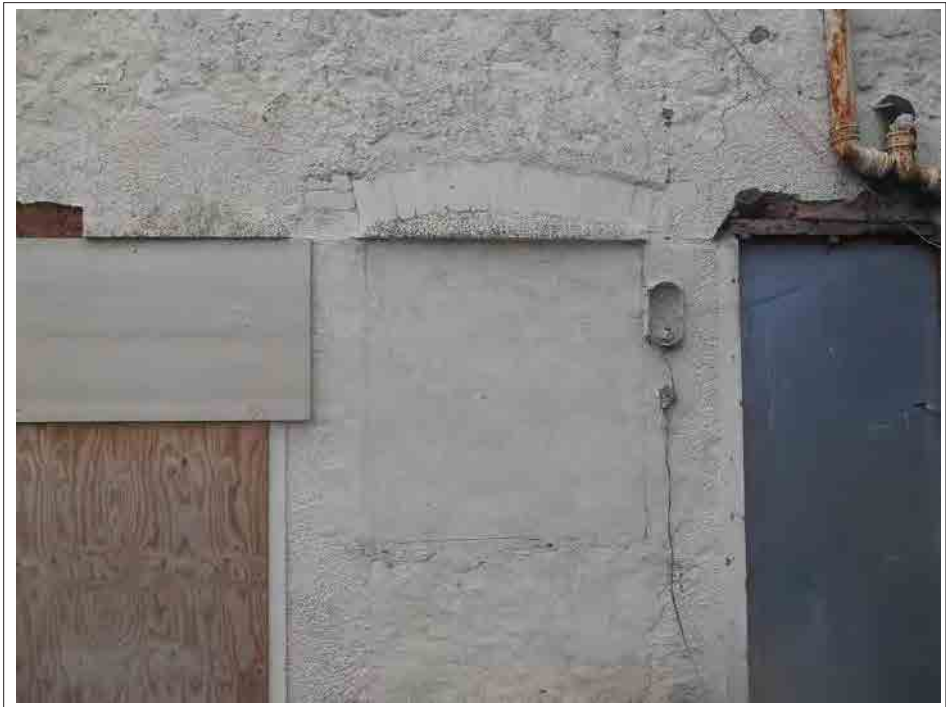
Plate 153. Detail of window hood.
