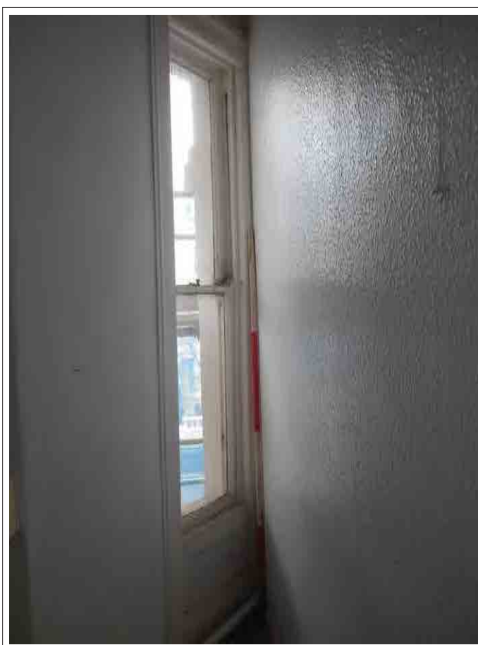
Plate 72. View of Room 7. Storeyed canted three-light window blocked by wall addition, looking N.
