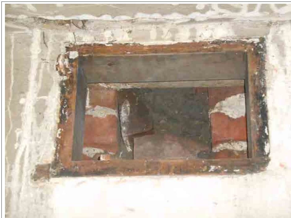
Plate 143. Blocked vent, west facing wall.
