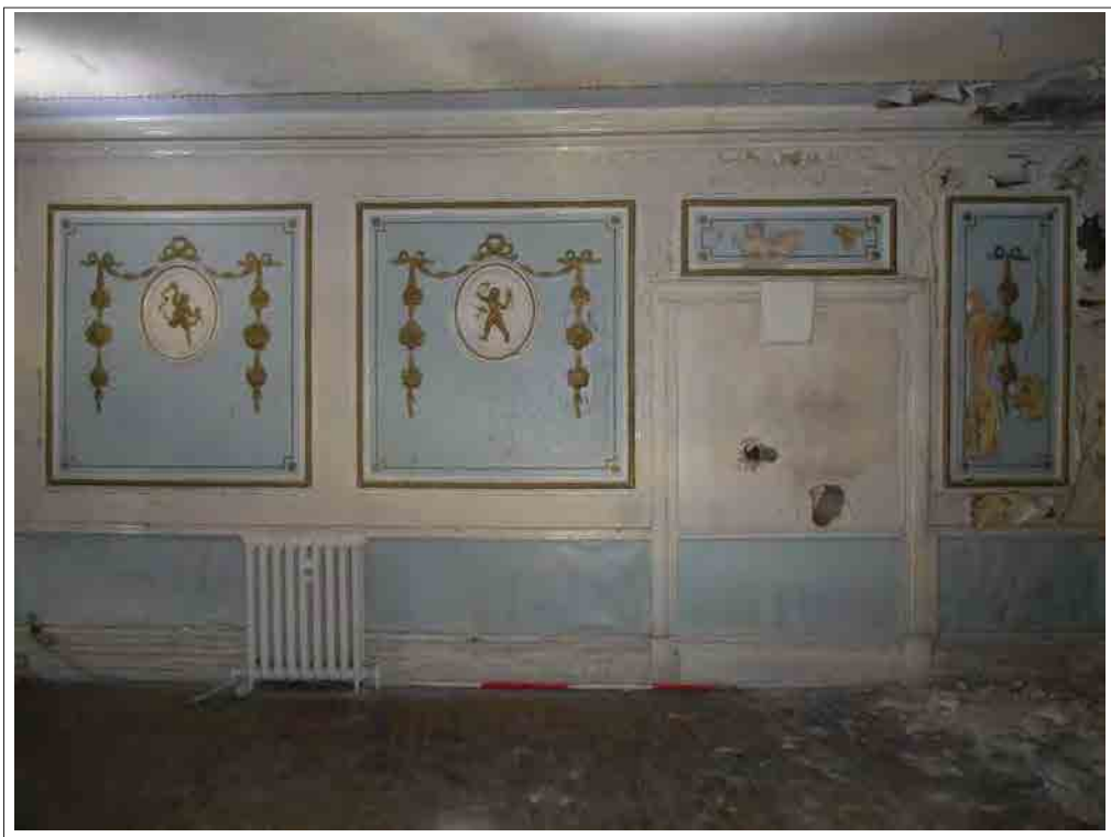
Plate 19. Blocked door, subsequently decorated, looking N.
