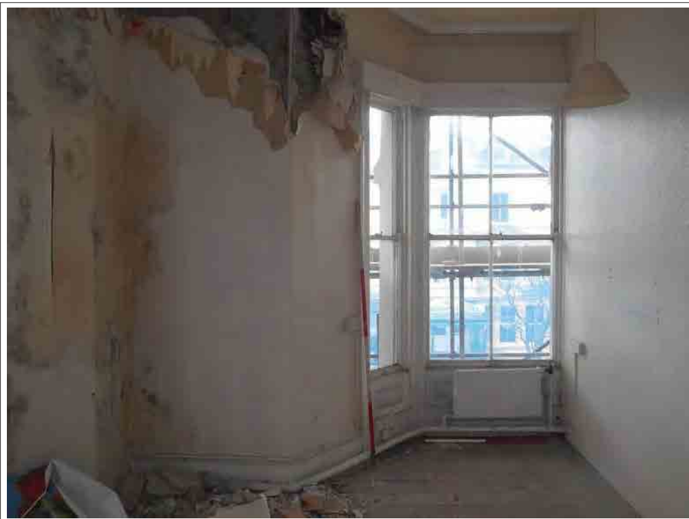
Plate 73. View of Room 7. Canted three-light window blocked by wall addition looking N.
