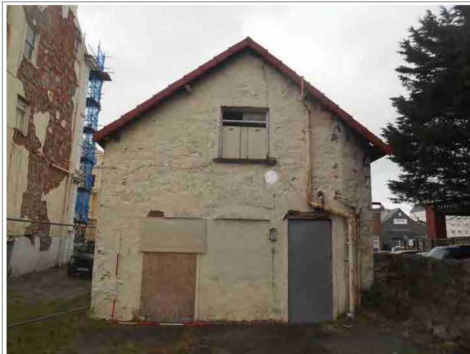
Plate 151. View of back entrance. Windows and doors are not original and demonstrate a number of alterations over time. 1960's hoods. First floor window with reveal toothed brick effect. Scales 2 x 2m
