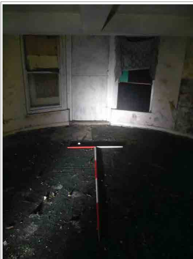
Plate 110. Canted five-light window currently blocked, looking NE.
