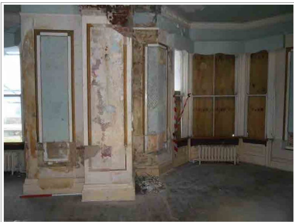
Plate 31. Projected wall evidencing different layers of decoration. Looking NW.
