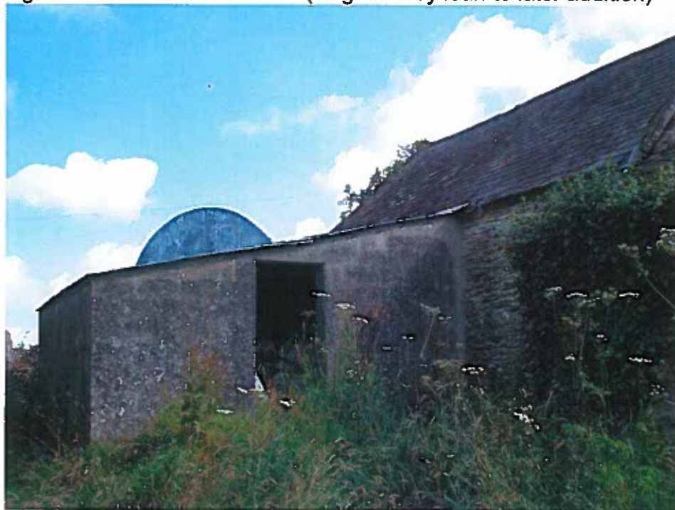
Fig. 2 BARN 01: Exterior View (single storey lean-to later addition) - south west
