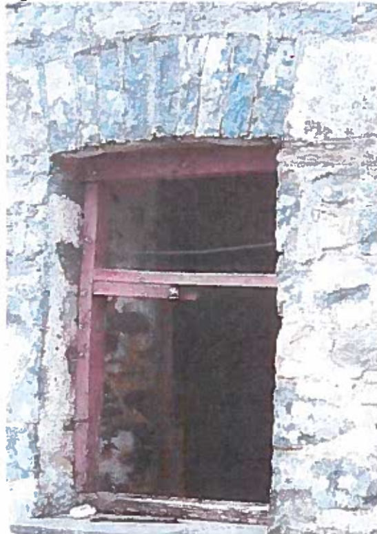
Fig. 14 BARN 01: Exterior View, two storey – window & slate cill
