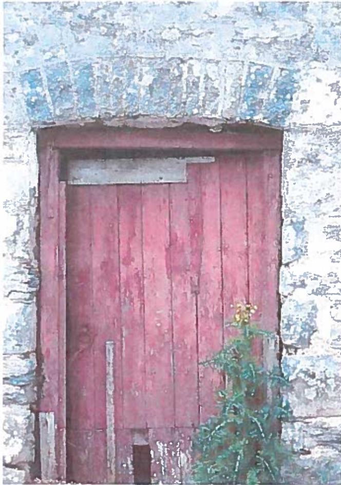
Fig. 13 BARN 01: Exterior View, two storey – door, stone arch & quoins
