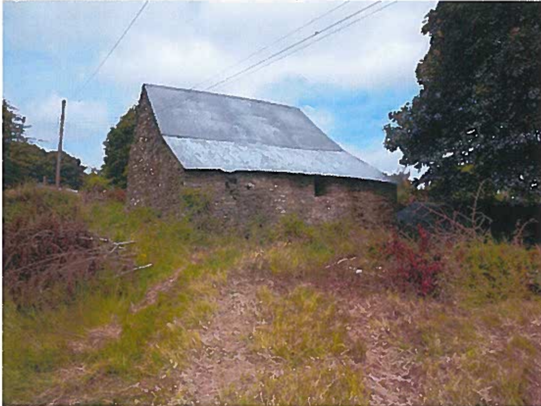
Fig. 11 BARN 02: Exterior View, two storey – walls
