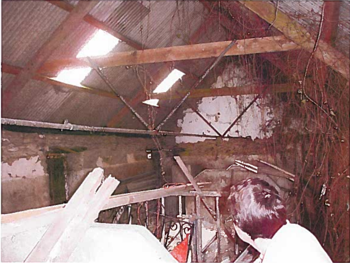
Fig. 8 BARN 01: Interior View, single storey (lower section) – truss and purlins
