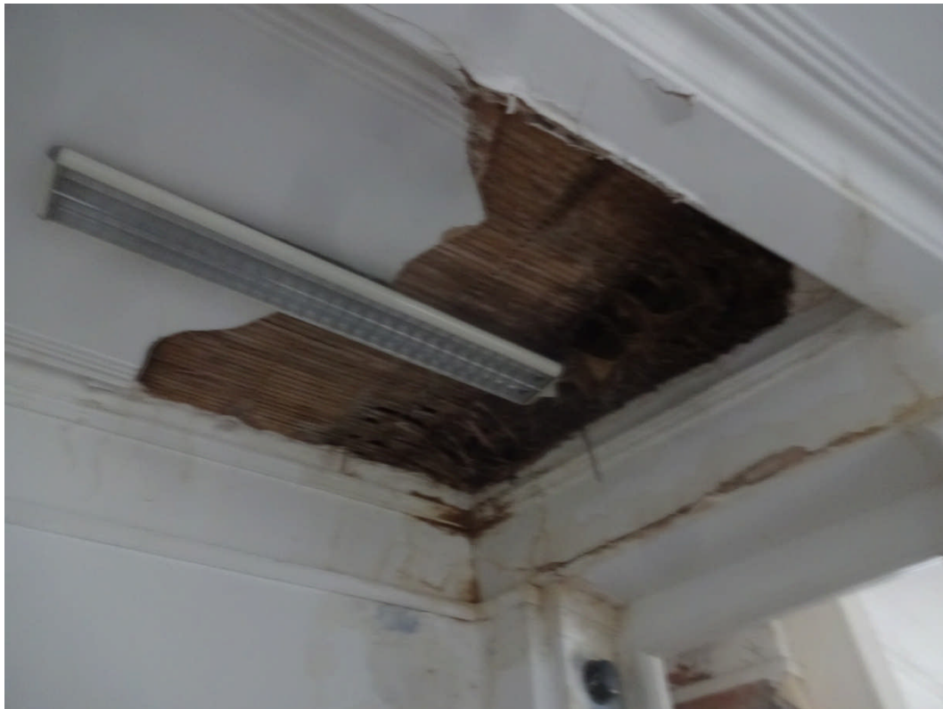
Figure 6 - damage to ground floor ceiling through dry rot
