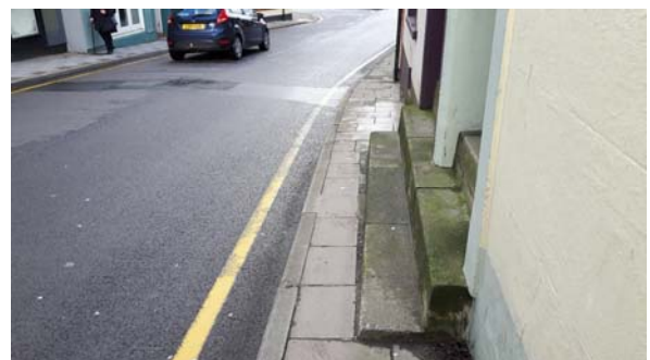
Figure 3-6 Narrow Footway and trip hazard along High Street view west
