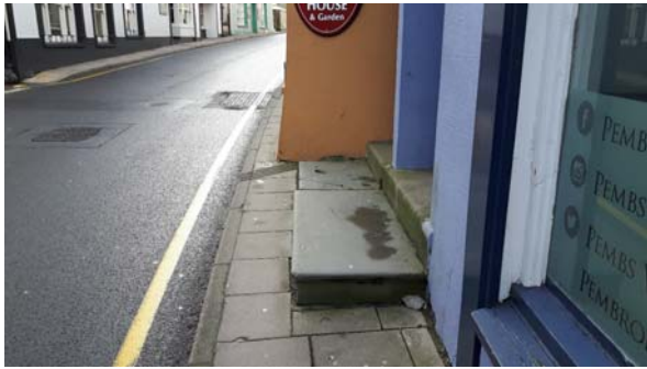
Figure 3-7 Narrow Footway and trip hazard along High Street view west
