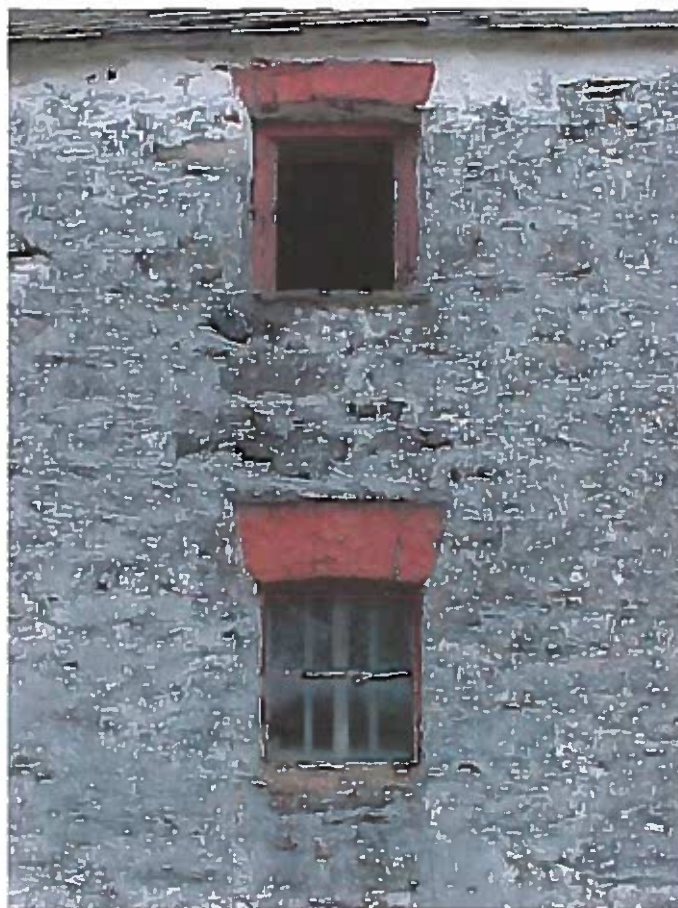
PHOTOGRAPH NO. 6 – TYPICAL GROUND & FIRST FLOOR WINDOWS (SOUTH VIEW)
