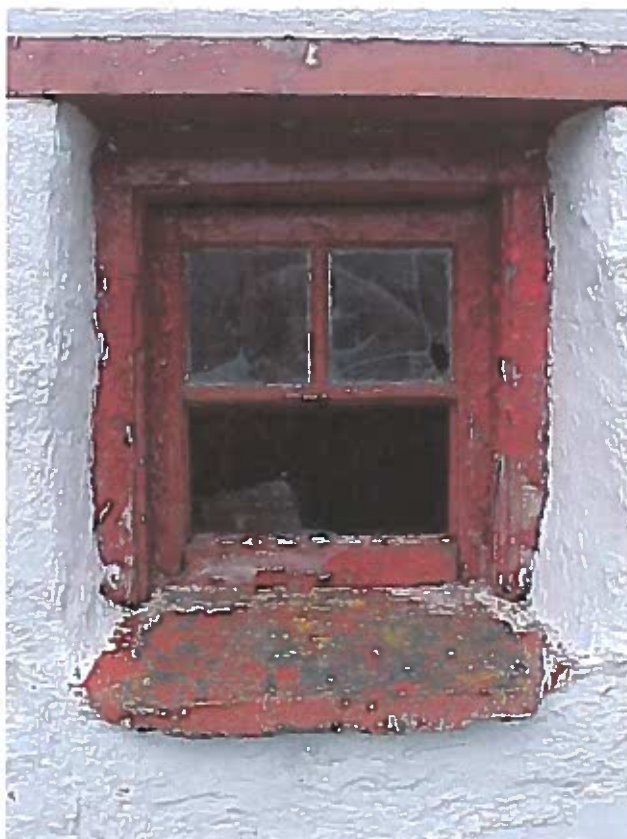
PHOTOGRAPH NO. 3 – WINDOW (SOUTH VIEW)
