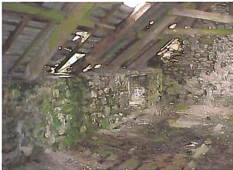
PHOTOGRAPH NO. 12 – FIRST FLOOR PART INTERNAL SOUTH VIEW
