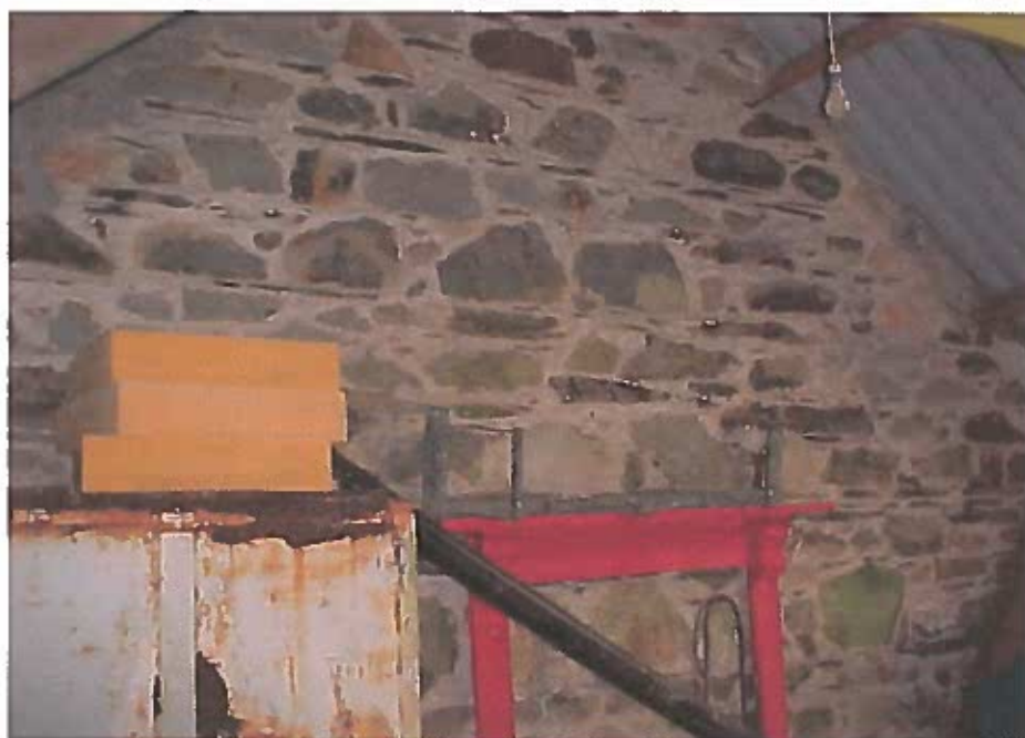
PHOTOGRAPH NO. 12 – INTERNAL WEST VIEW (1)
