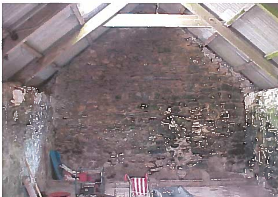
PHOTOGRAPH NO. 7 – INTERNAL WEST VIEW
