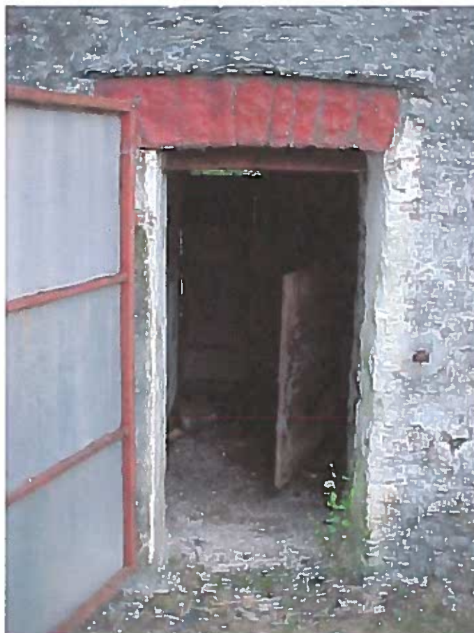
PHOTOGRAPH NO. 7 – DOOR (SOUTH VIEW)
