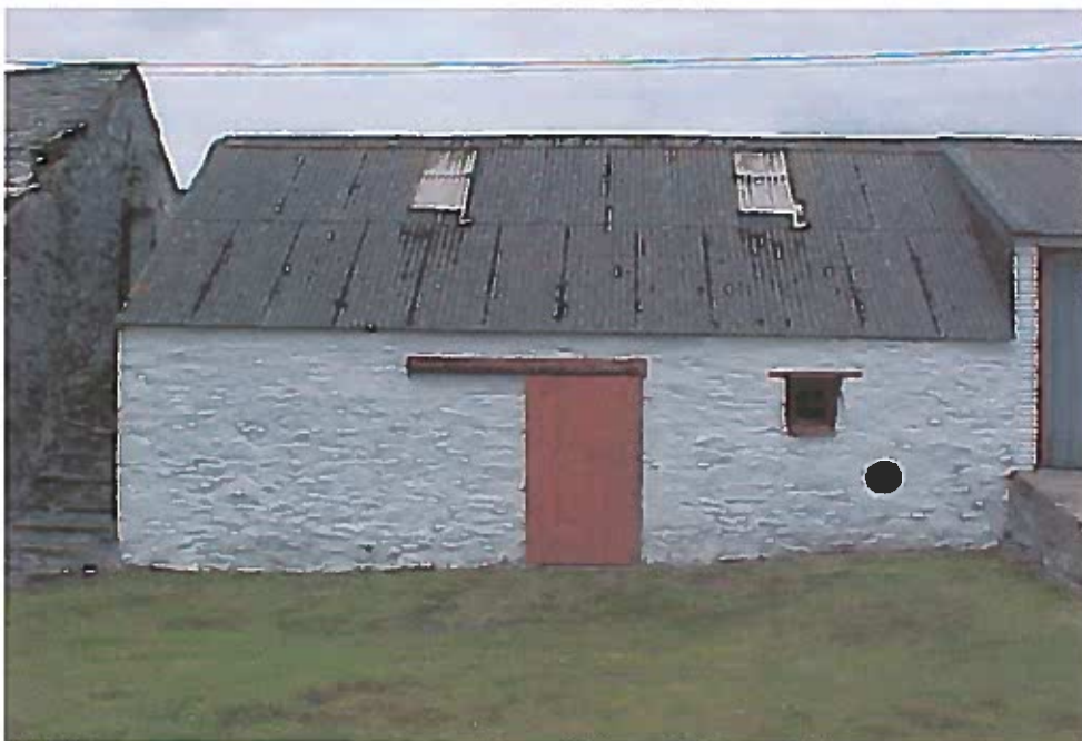
PHOTOGRAPH NO. 2 – SOUTH VIEW
