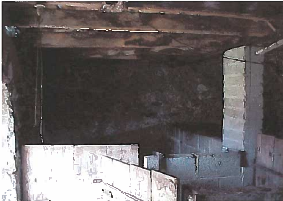
PHOTOGRAPH NO. 10 – GROUND FLOOR PART INTERNAL WEST VIEW (1)
