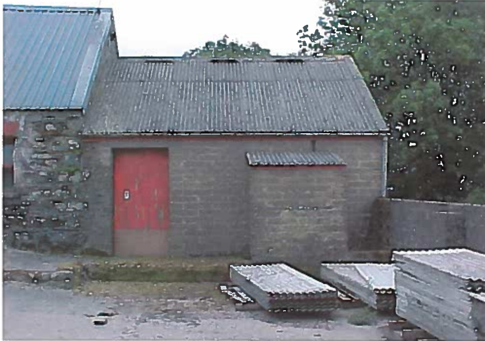
PHOTOGRAPH NO. 1 – NORTH VIEW
