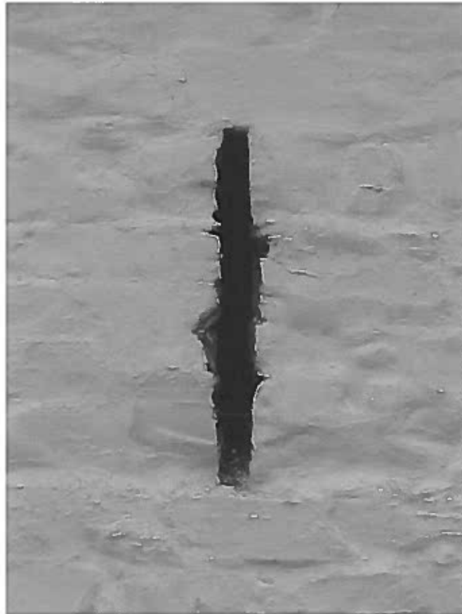
PHOTOGRAPH NO. 5 – TYPICAL RECTANGULAR SLIT (NORTH VIEW)
