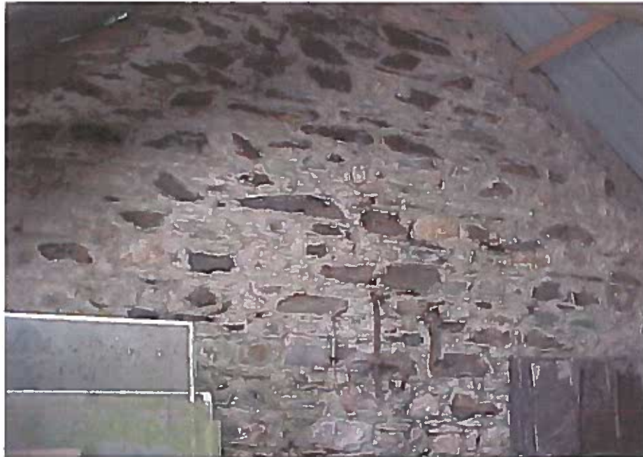
PHOTOGRAPH NO. 13 – INTERNAL EAST VIEW (1)
