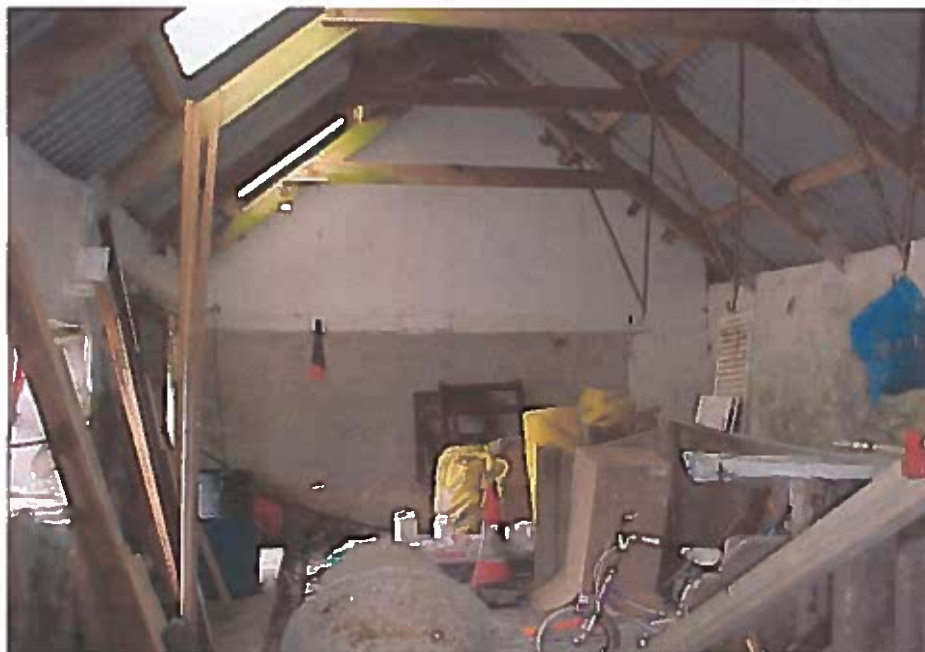
PHOTOGRAPH NO. 14 – INTERNAL EAST VIEW (2)
