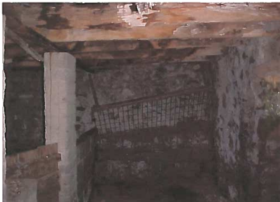
PHOTOGRAPH NO. 11 – GROUND FLOOR PART INTERNAL WEST VIEW (2)
