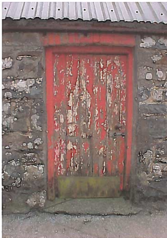
PHOTOGRAPH NO. 9 – TYPICAL DOOR (NORTH VIEW)
