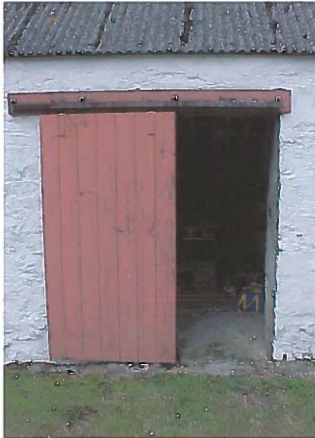
PHOTOGRAPH NO. 4 – DOOR (SOUTH VIEW)
