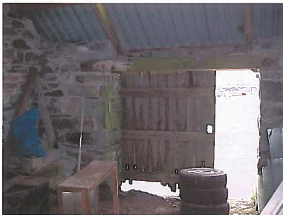
PHOTOGRAPH NO. 11 – PART INTERNAL NORTH VIEW
