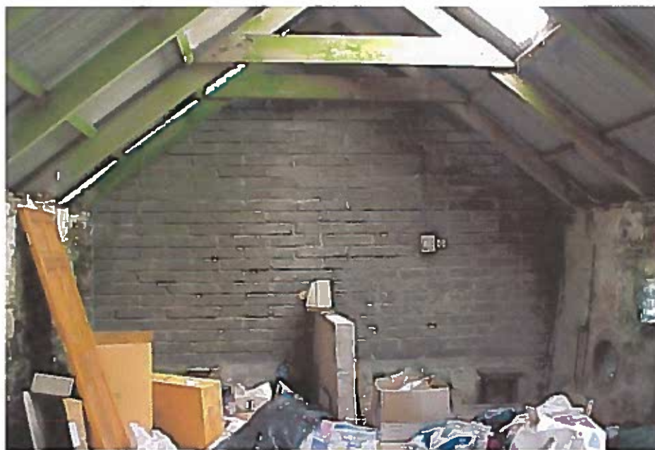
PHOTOGRAPH NO. 6 – INTERNAL EAST VIEW
