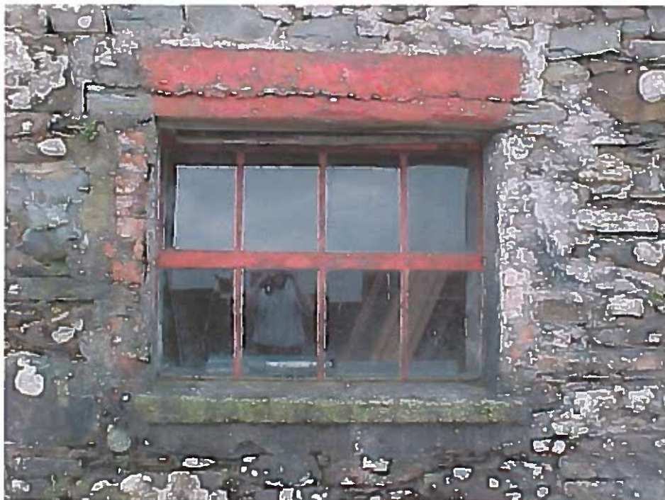
PHOTOGRAPH NO. 8 – TYPICAL WINDOW (NORTH VIEW)
