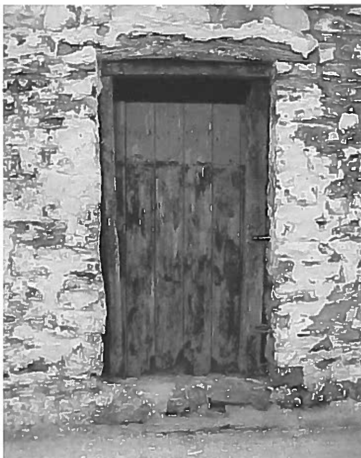
PHOTOGRAPH NO. 4 – DOOR (NORTH VIEW)
