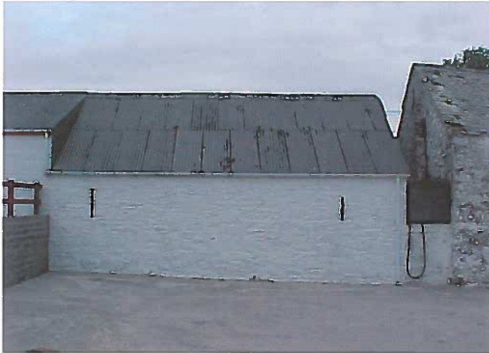
PHOTOGRAPH NO. 1 – NORTH VIEW
