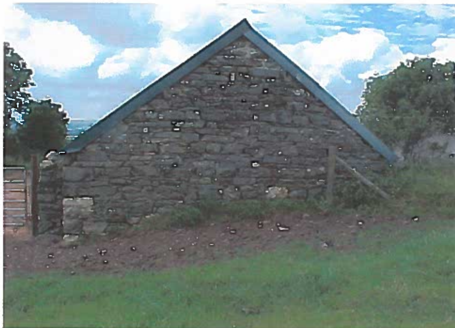
PHOTOGRAPH NO. 4 – EAST VIEW
