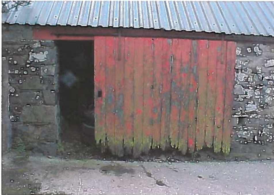
PHOTOGRAPH NO. 7 – SLIDING DOUBLE DOOR (NORTH VIEW)
