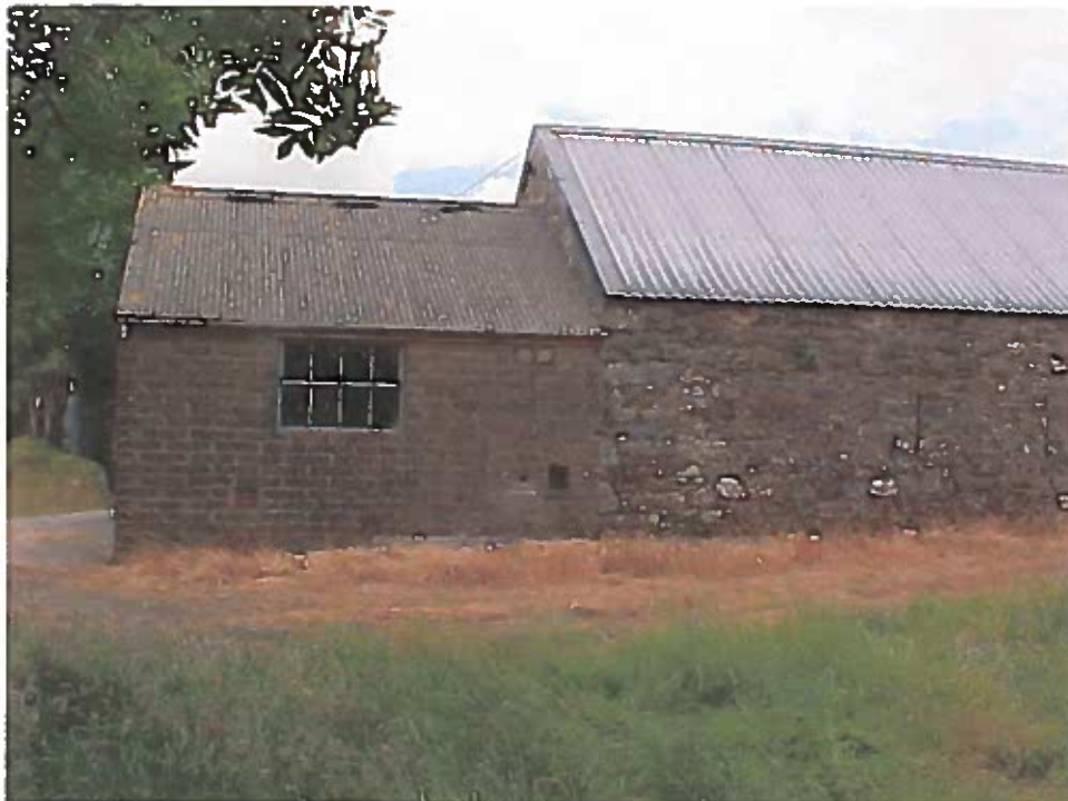
PHOTOGRAPH NO. 2 – SOUTH VIEW
