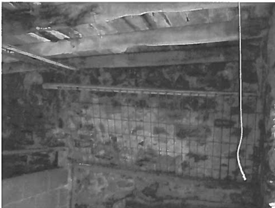
PHOTOGRAPH NO. 9 – GROUND FLOOR PART INTERNAL EAST VIEW (2)
