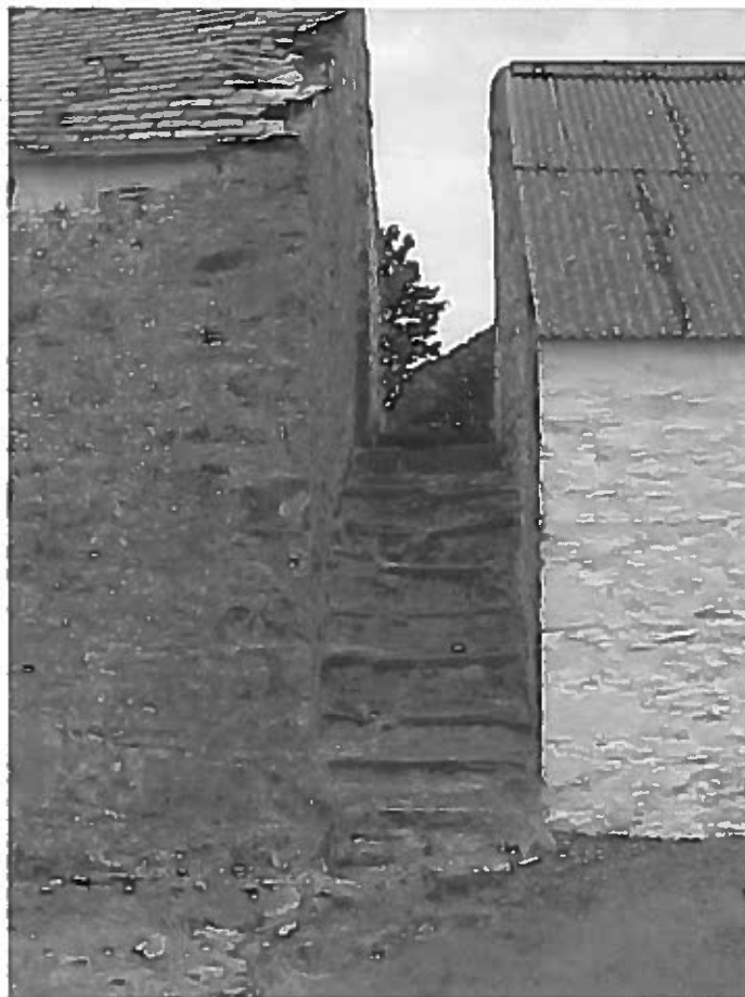
PHOTOGRAPH NO. 5 – EXTERNAL STEPS (SOUTH VIEW)
