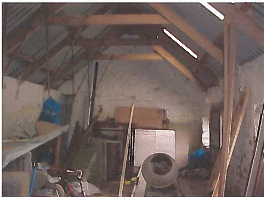
PHOTOGRAPH NO. 15 – INTERNAL WEST VIEW (2)
