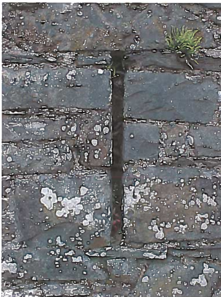
PHOTOGRAPH NO. 10 – TYPICAL RECTANGULAR SLIT (SOUTH VIEW)
