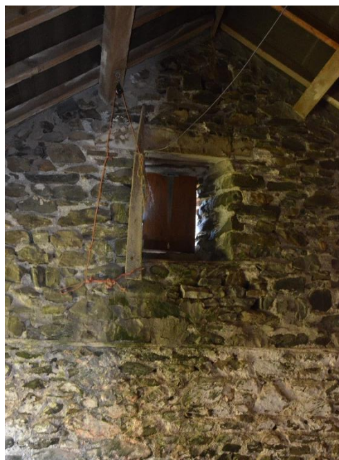
Plate 46: Building c West Section -Ventilation opening Western Elevation
