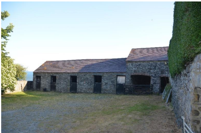
Plate 35: Building C South Elevation
