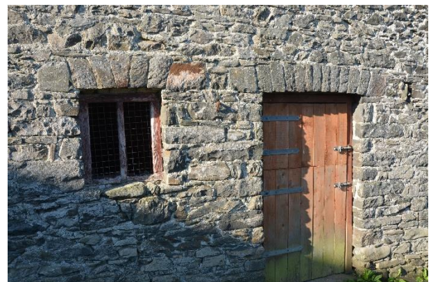
Plate 19: Building B North Elevation -Central Section Access
