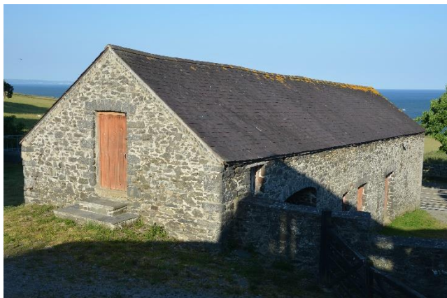
Plate 7: Building B East and North Elevations
