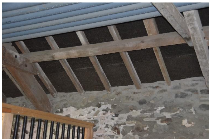
Plate 42: Building C West Section -Roof Construction
