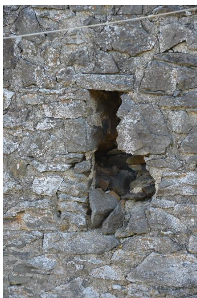
Plate 11: Building B Ventilation Slit Central Section South Elevation
