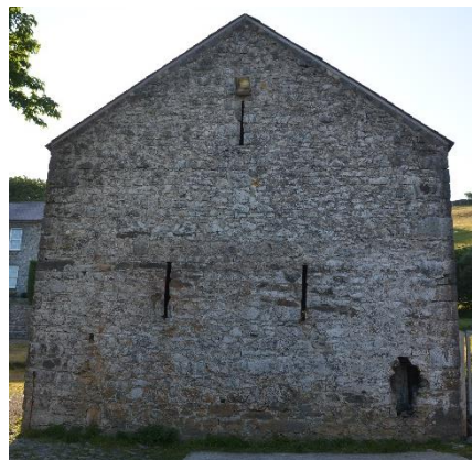
Plate 10: Building B West Elevation
