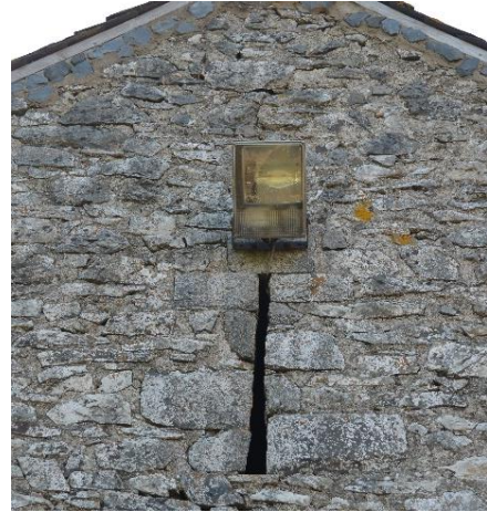
Plate 15: Building B West Elevation -Top Ventilation Slits
