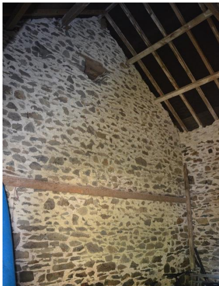
Plate 26: Building B West Section -Internal Wall with Central Section
