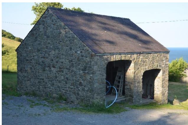
Plate 4: Building A East and North Elevation
