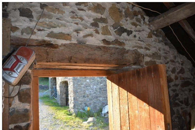
Plate 31: Building B Eastern Section Entrance Door
