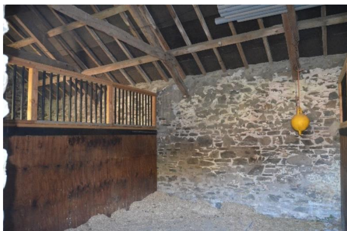
Plate 43: Building C West Section -Internal Stonework
