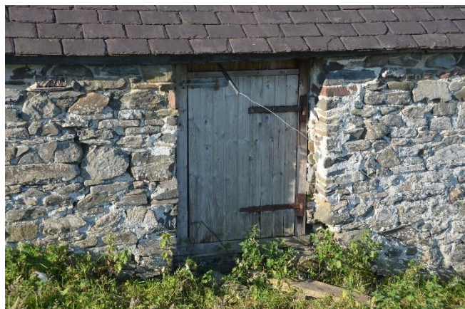
Plate 50: Building C Ventilation Opening North Elevation
