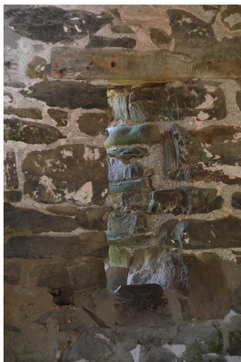
Plate 45: Building C West Section -Ventilation Slit to North
