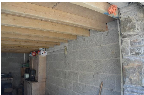
Plate 6: Building A Internal Construction
