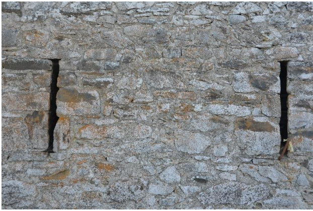
Plate 14: Building B West Elevation -Ground Floor Ventilation Slits
