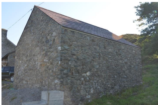
Plate 5: Building A West and South Elevation
