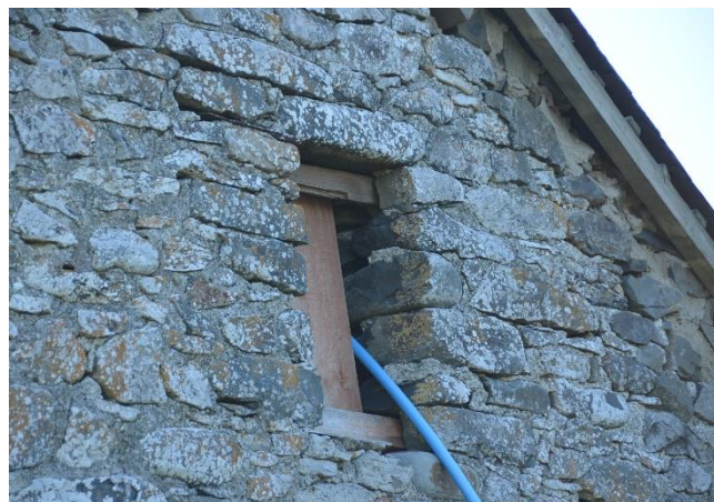
Plate 53: Building C Ventilation Opening West Elevation
