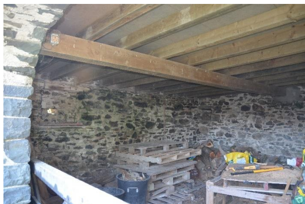
Plate 18: Building B East Section Ground Floor Internal Stone Work
