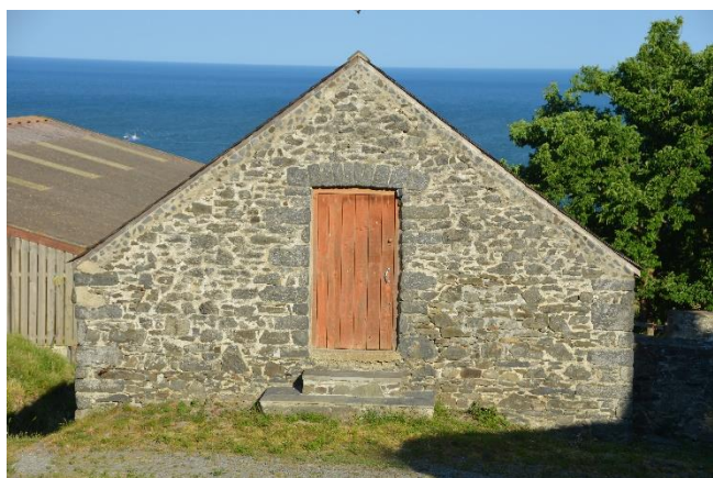
Plate 30: Building B Eastern Elevation
