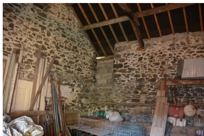
Plate 23: Building B Central Section -First Floor Access from South
