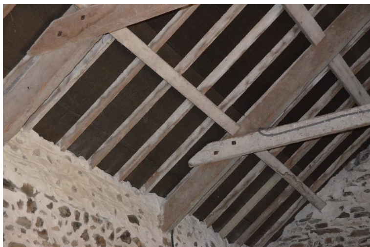
Plate 27: Building B West Section -Roof Construction
