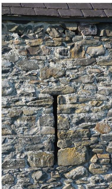
Plate 51: Building C Ventilation Slit on North Elevation
