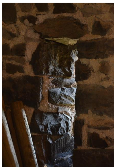
Plate 29: Building B West Section -Ground Floor Ventilation Slit to North
