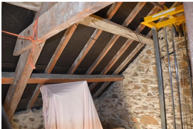
Plate 32: Building B Eastern Section Roof Construction
