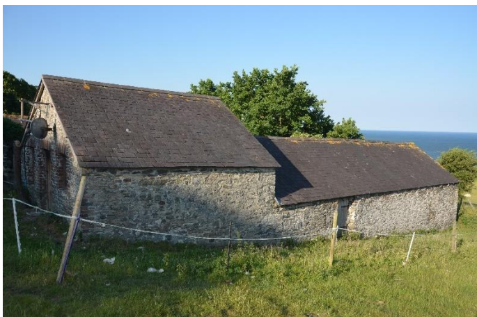
Plate 49: Building C East and North Elevations
