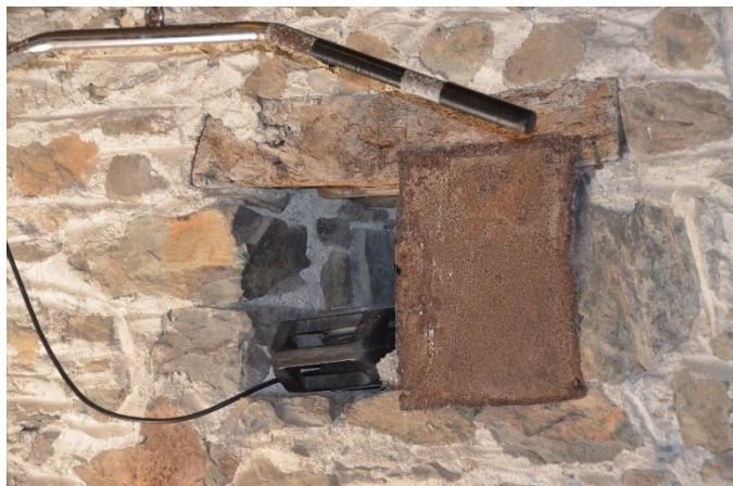
Plate 34: Building B Ventilation Opening into Central Section
