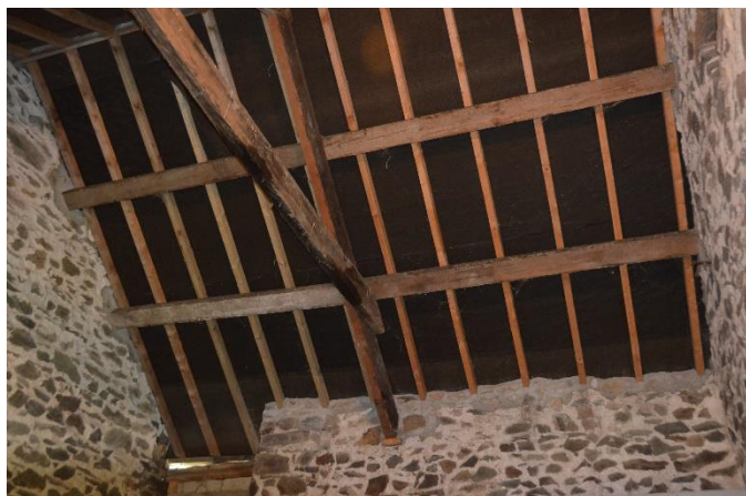
Plate 22: Building B Central Section -Roof Construction
