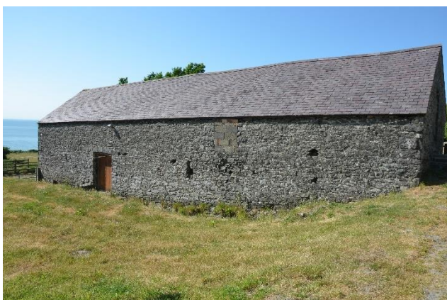
Plate 9: Building B South Elevation
