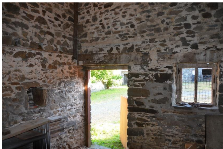
Plate 21: Building B Central Section -Internal Access from North
