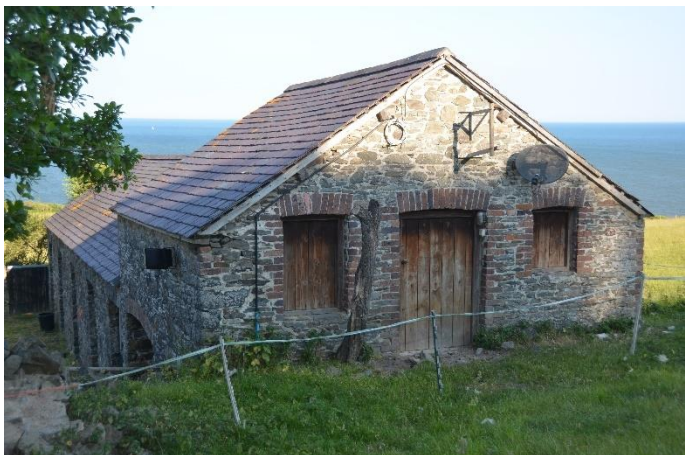
Plate 47: Building C East Elevation
