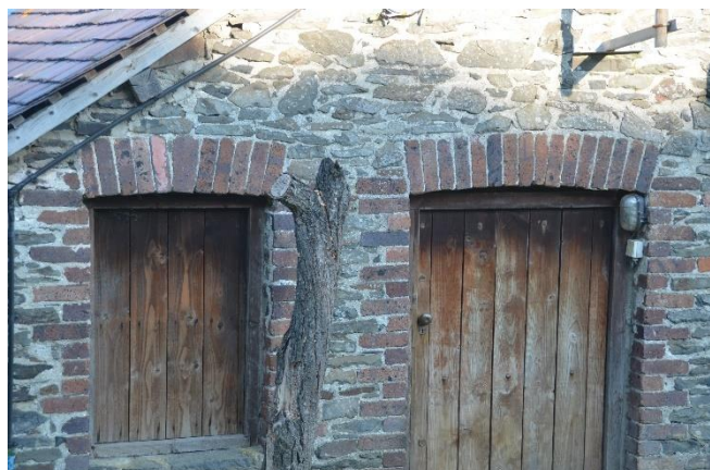
Plate 48: Building C East Elevation Brickwork
