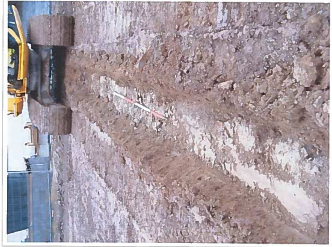
Plate 4: Southern foundation trench, showing subsoil removed to the top of the natural, looking east. Scale 2m
