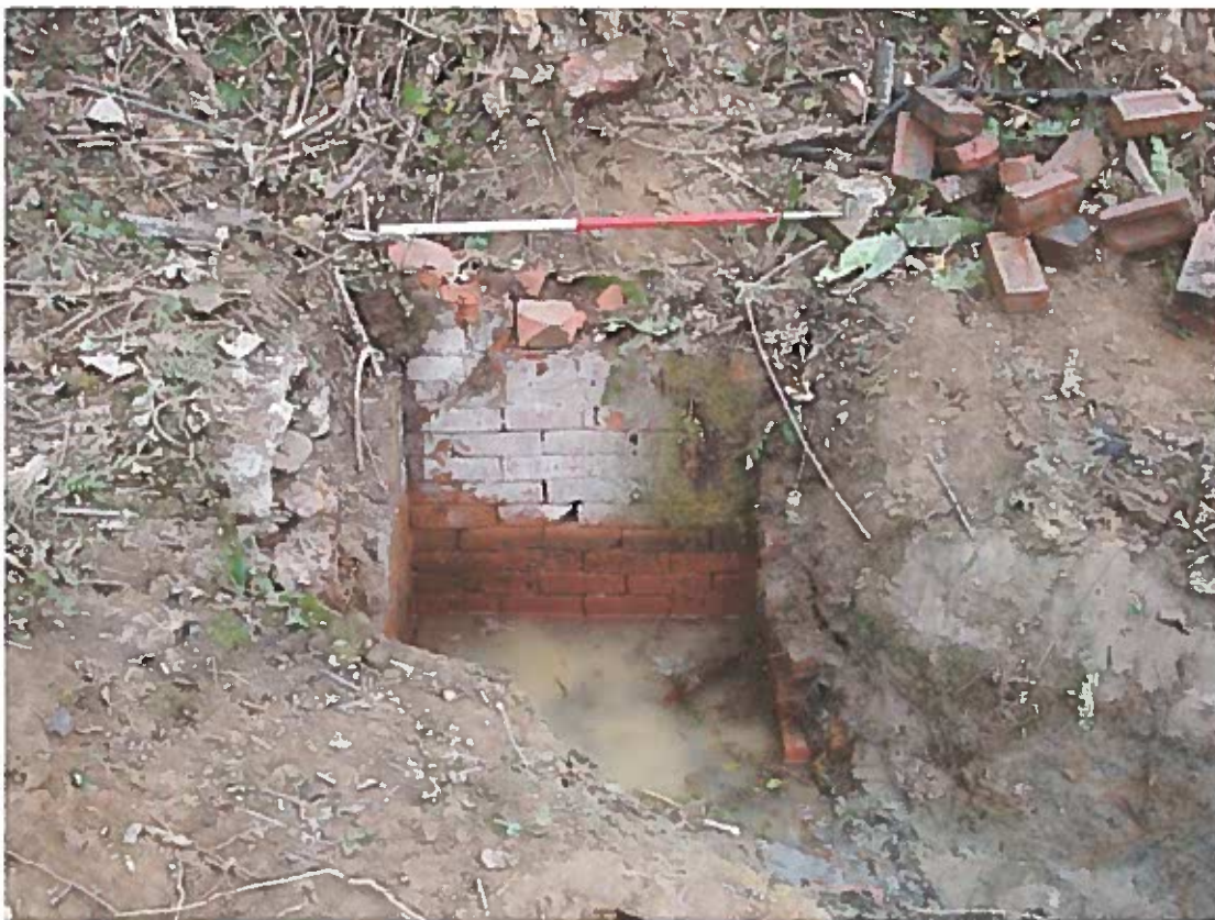
Plate 4: The brick-lined spring chamber (Feature No. 020)
