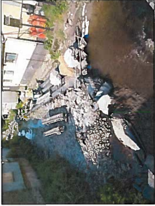
Plate 2 Damming and diverting of river by bridge in preparation for dredging. Looking south from bridge.
