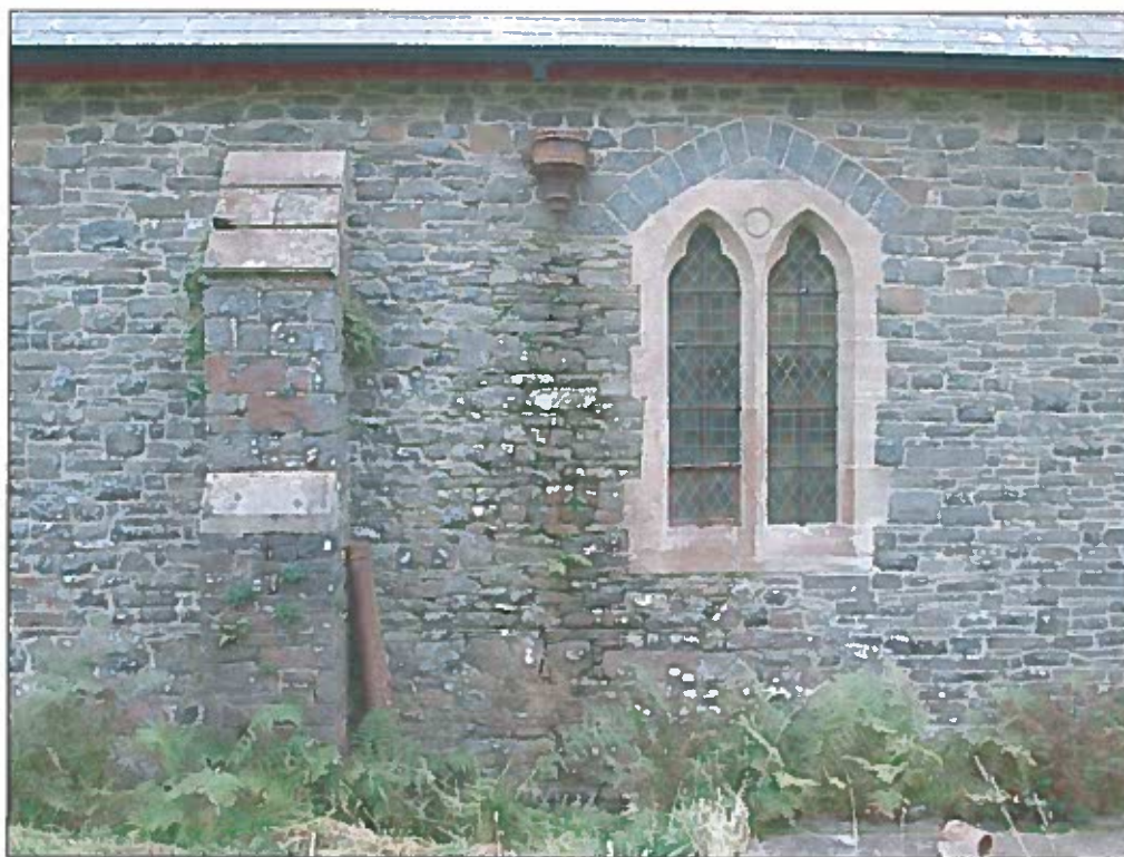
Plate 11. Nant Cwnlle Church. North facing elevation, west end showing area of 19th century extension. Note different mortar types. Looking south.
