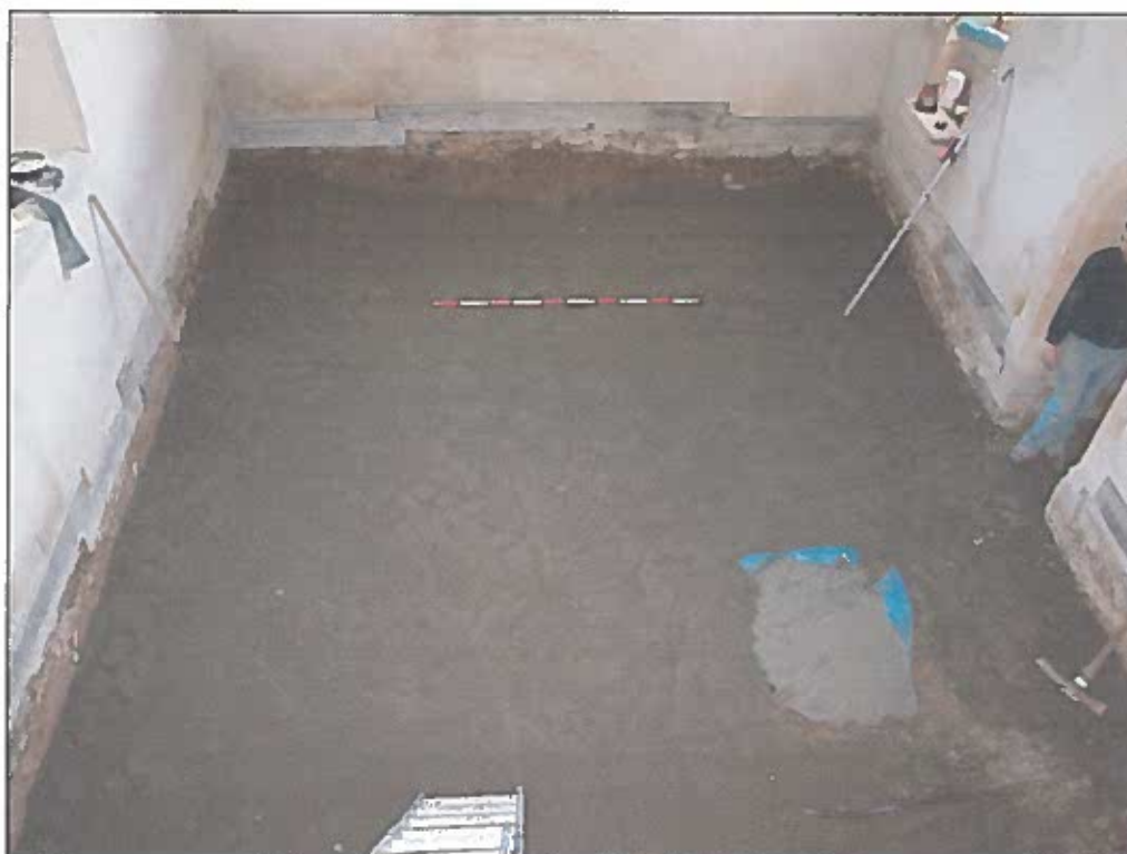
Plate 47. View of Chancel floor following floor reduction and terram sheeting laid down with archaeological deposits preserved beneath in situ. Looking northeast.
