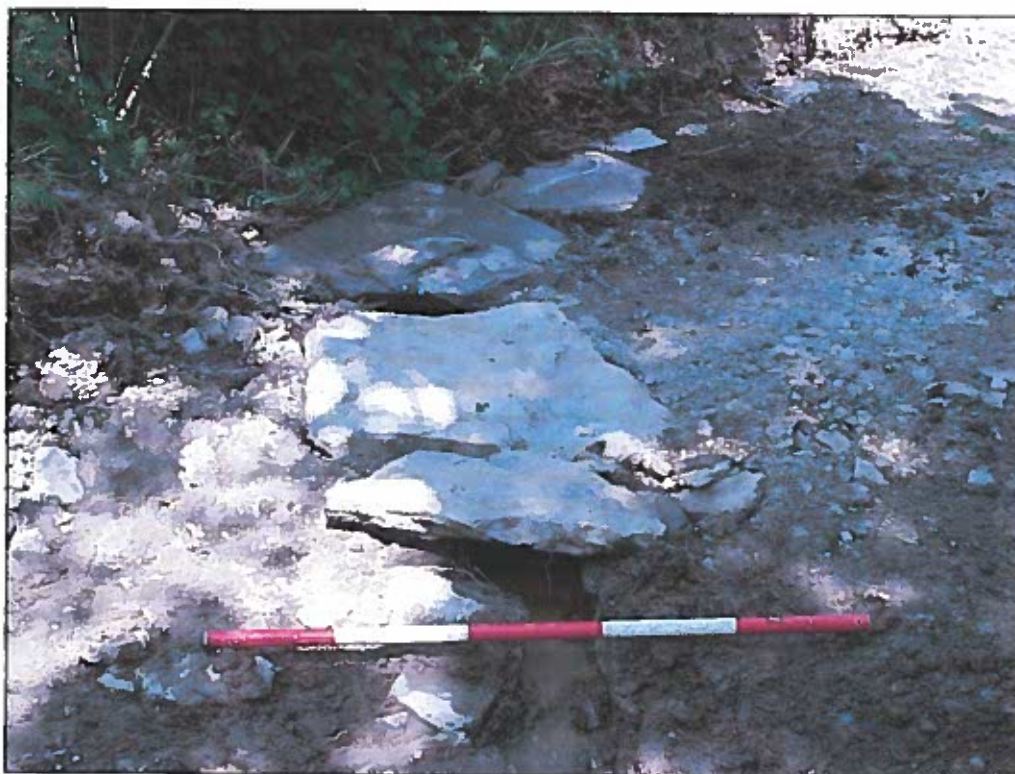
Plate 20. Exposed stone culvert running across church access track from natural spring by old school house. Looking northeast toward school house, source of spring.
