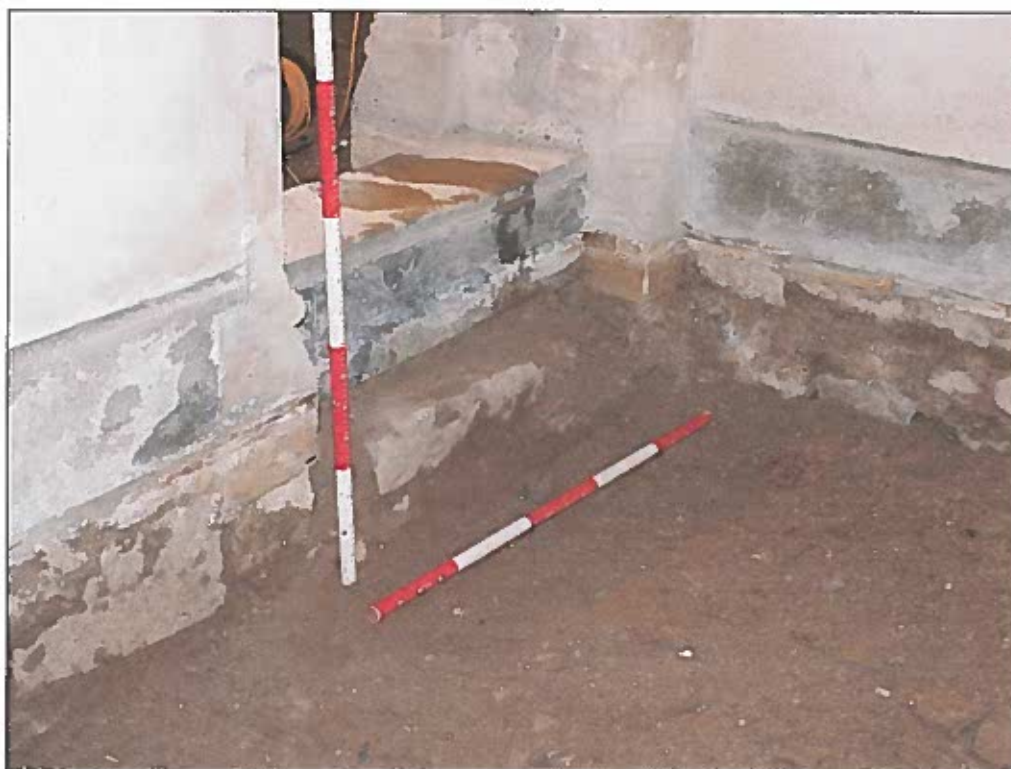
Plate 45. Exposed threshold into Chancel from Vestry following floor reduction. Looking northeast.
