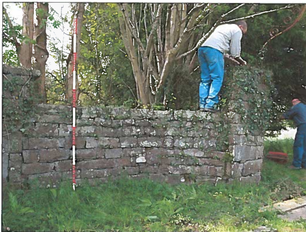
Plate 14. Working shot showing dismantling of entrance gate in order to allow access to church for proposed ground works. Looking west.
