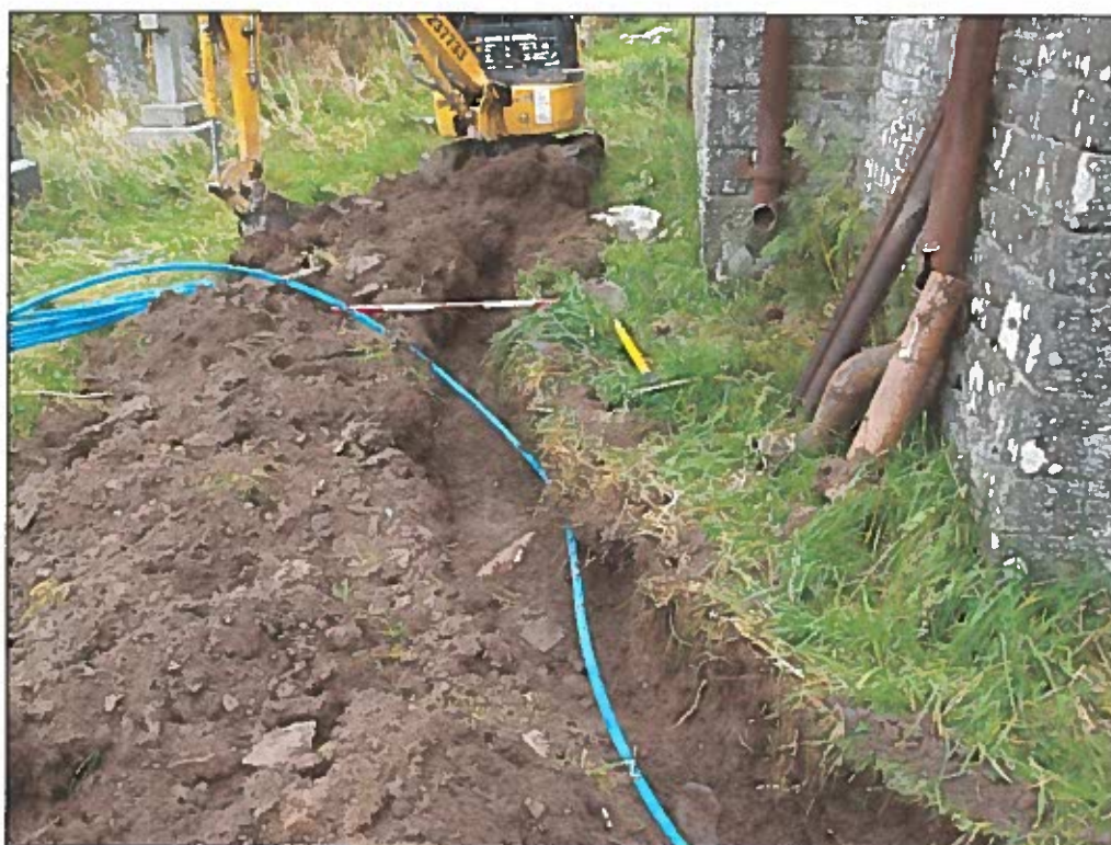
Plate 51. Service trench for foul drain alongside water service trench. Looking west.
