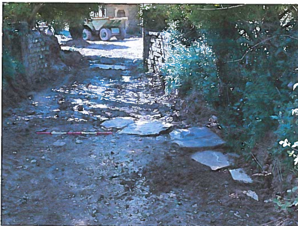
Plate 19. Exposed stone culvert running across church access track from natural spring by old school house. Looking west toward graveyard.
