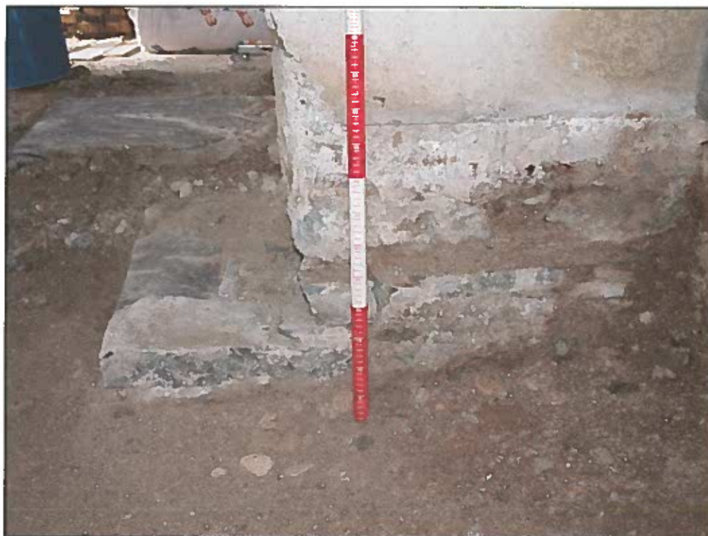
Plate 44. Base of support arch pillar between Chancel and Nave following floor reduction. Looking west.
