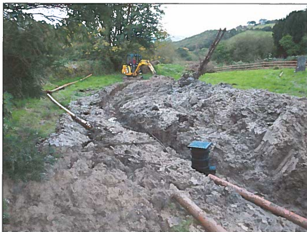
Plate 52. Trench for septic tank soakaway. Looking south.
