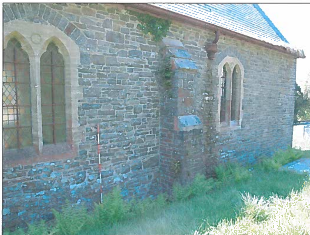
Plate 10. Oblique View of Nant Cwnlle Church north facing elevation showing buttress marking 1886/7 extension..
