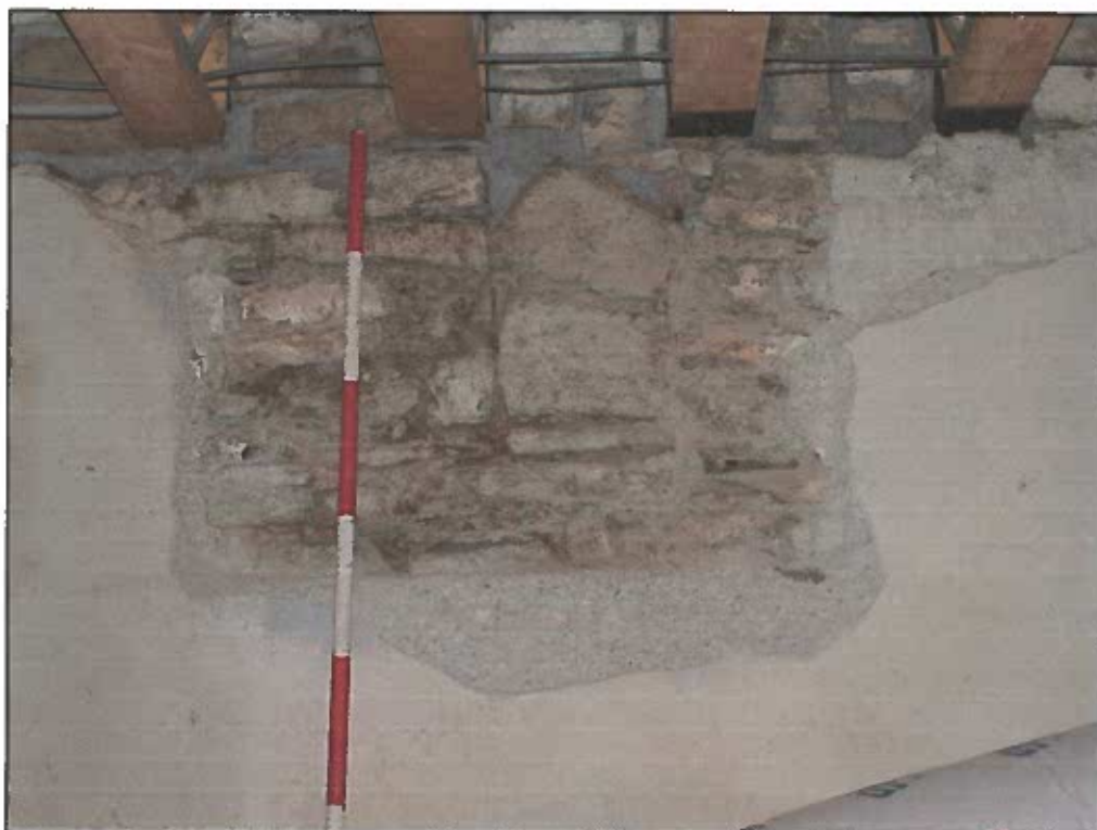
Plate 48. Exposed spring of blocked in arched window in north wall of Nave behind plasterwork following removal of memorial plaque. Looking north.
