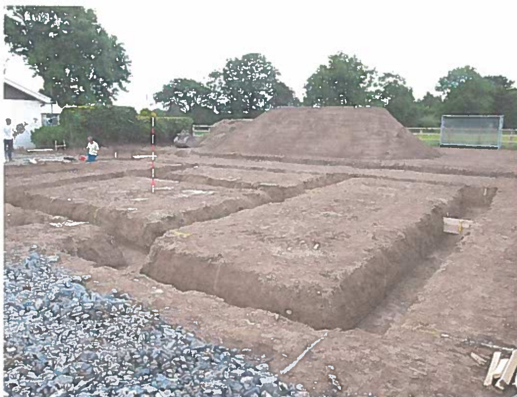
Plate 6. View of cut foundation trenches looking southeast
