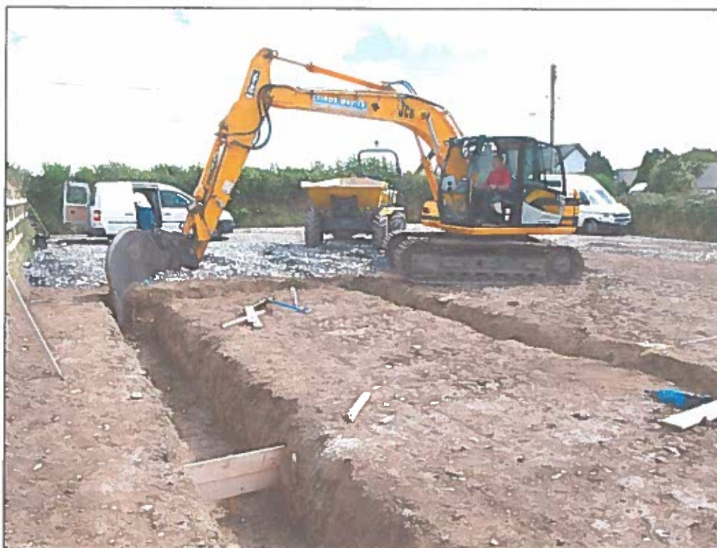
Plate 3. Working shot during cutting of foundation trenches.
