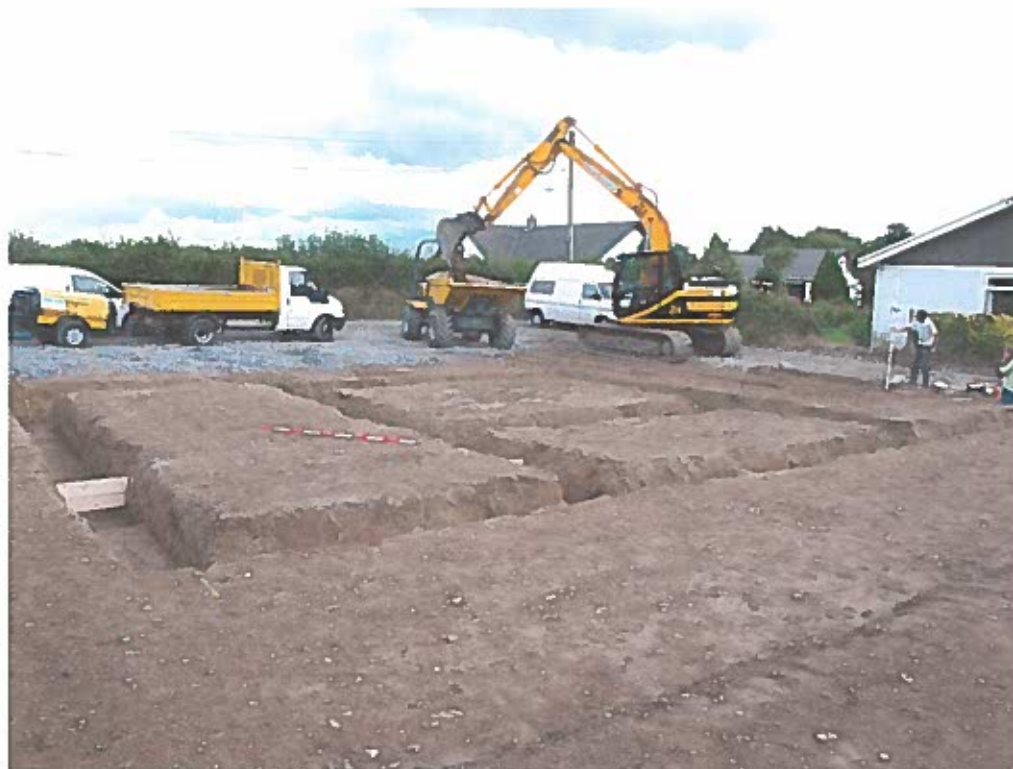
Plate 5. View of cut foundation trenches looking northeast.
