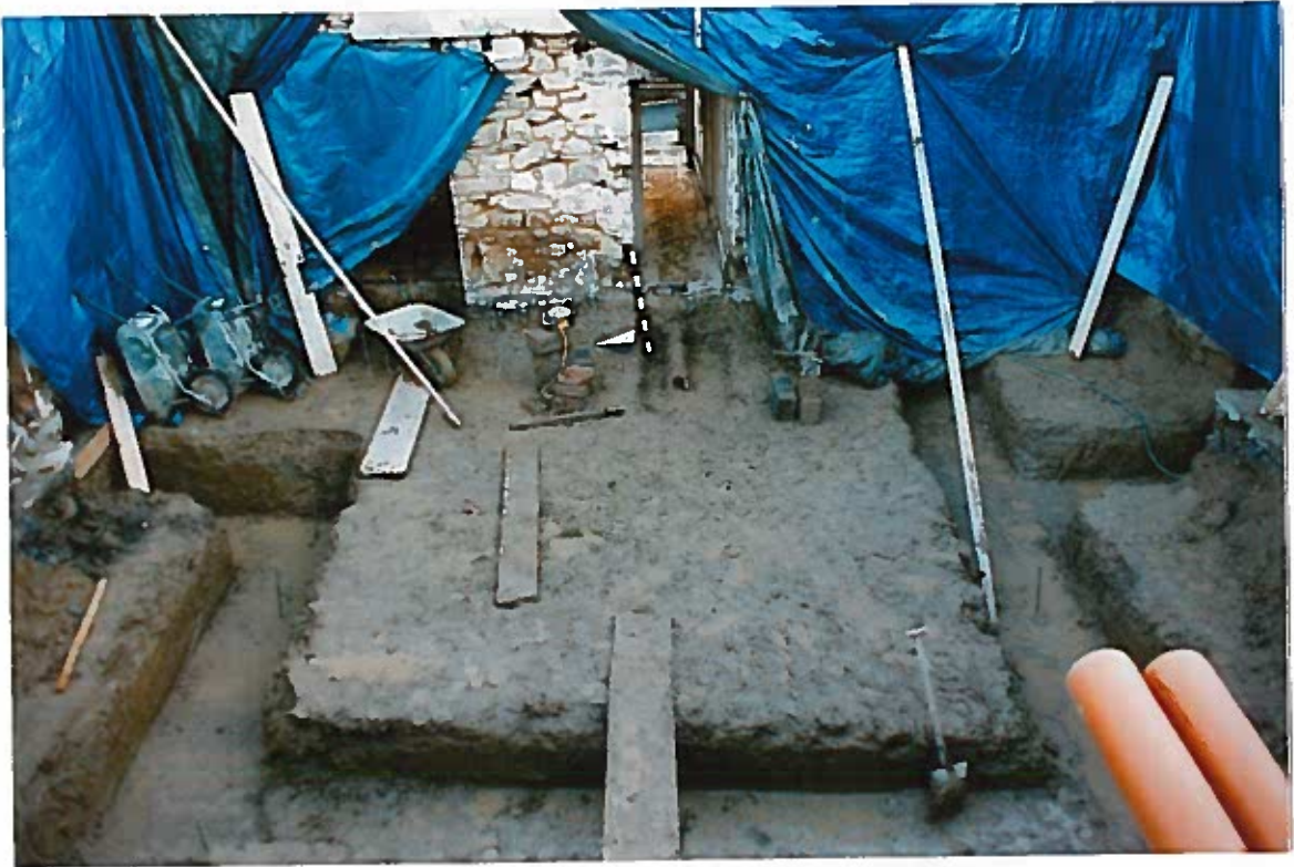
Foundation trenches for the extension from the west
