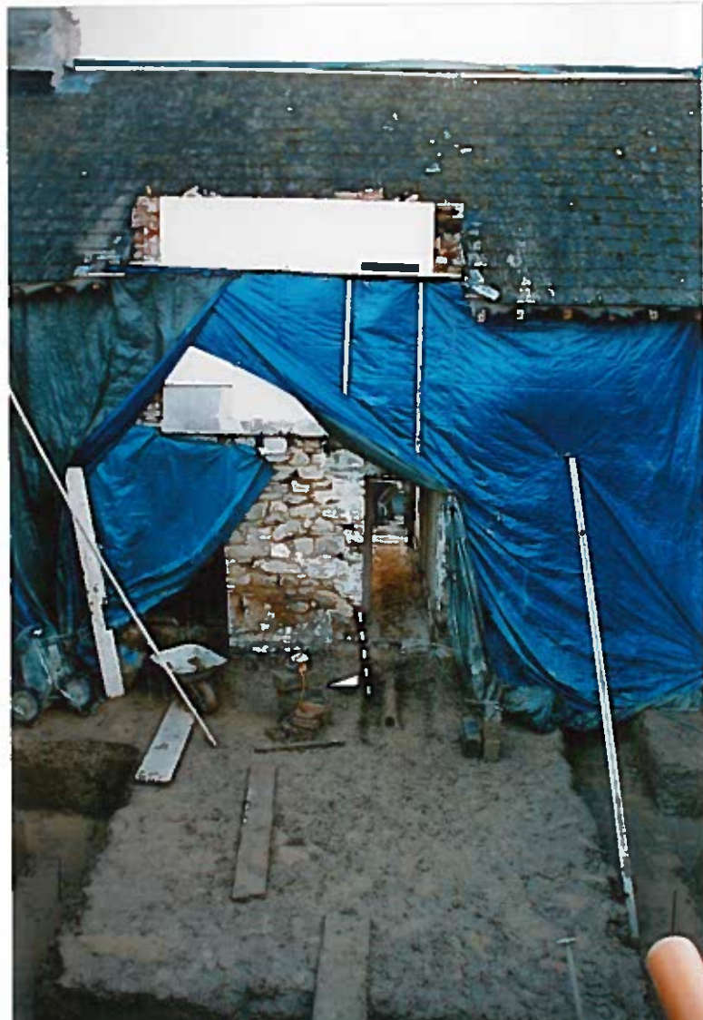
Foundation trenches for the extension from the west
