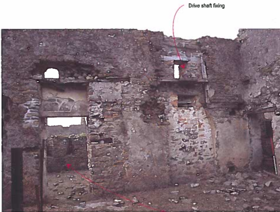
Plate 11. Drive shaft fixing
