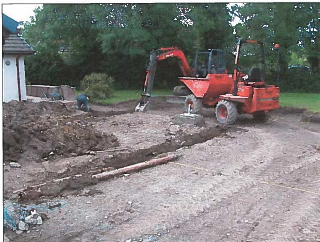
Plate 2. Top soil strip completed and former service trenches re-exposed. Looking southward.
