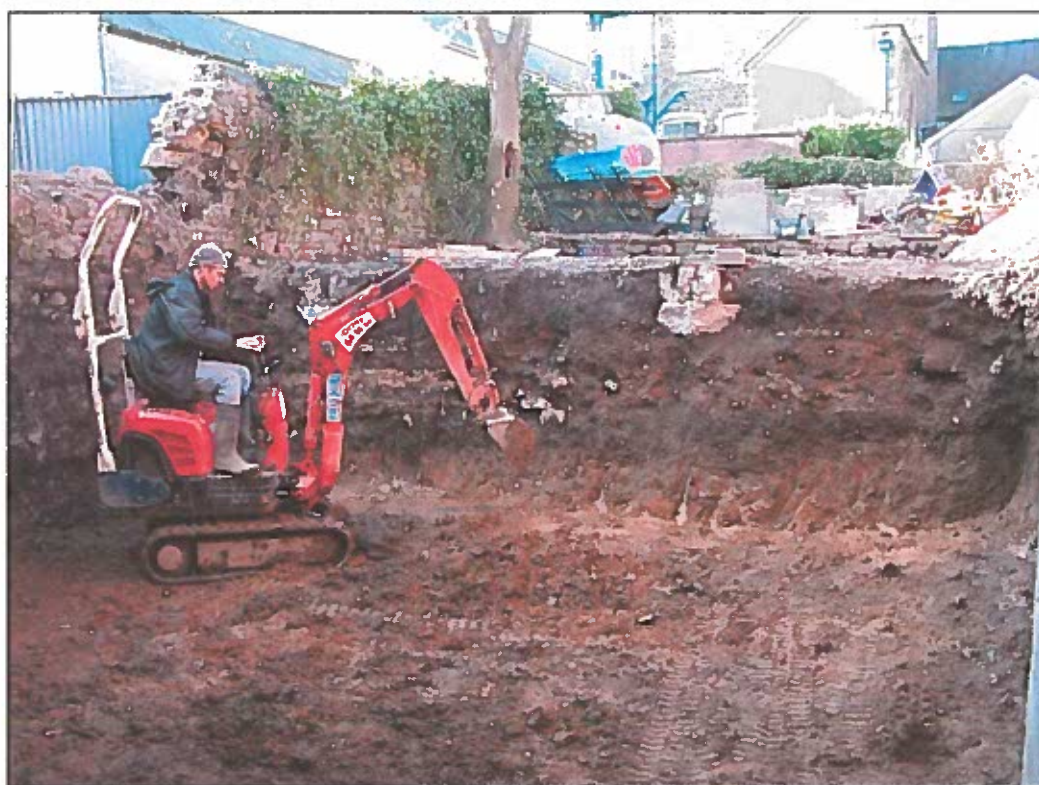
Plate 4. Working shot showing ground level reduction. Looking north-west.
