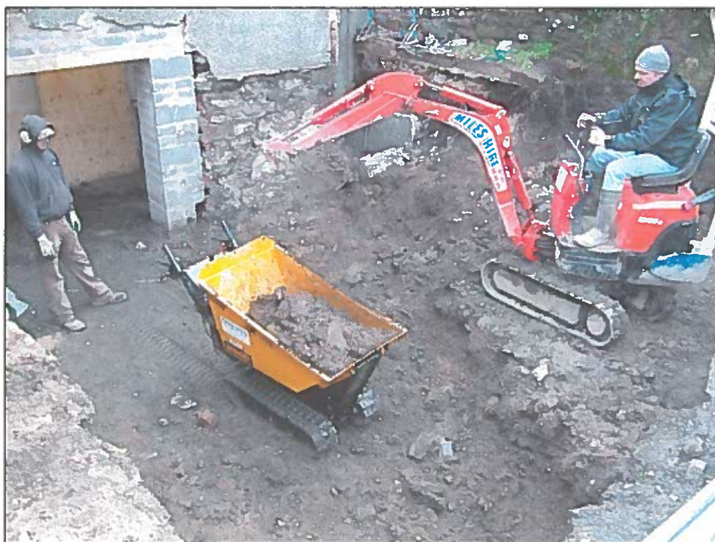
Plate 2. Working shot showing ground level being reduced and entrance way inserted through rear wall of pub.
