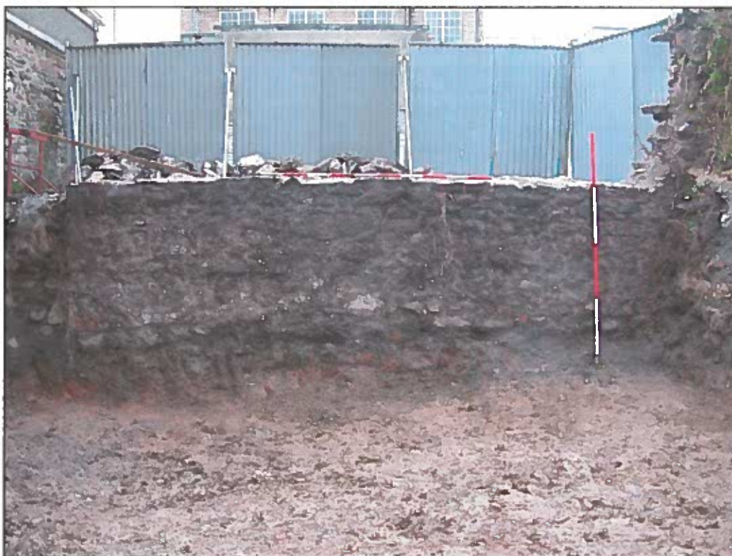
Plate 7. East facing garden stone wall with ground levels reduced. Upper half of wall removed for safety.
