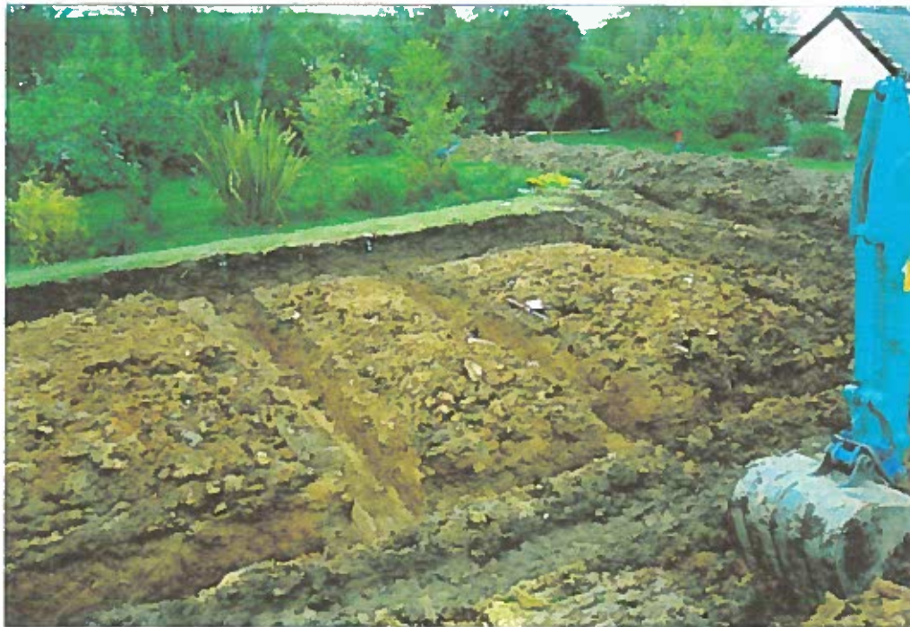
General observation of the foundation trenches for the new dwelling
