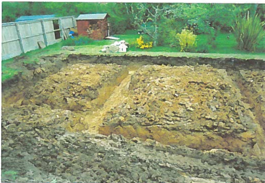
General observation of the foundation trenches for the new dwelling
