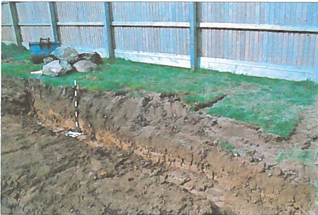
Test trench for foundations looking West
