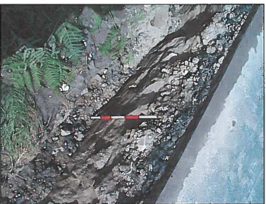
Plate 2. Side of trench showing section through stages of former road surfaces
