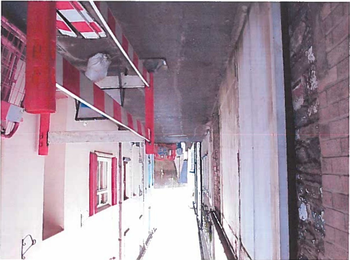
Plate 1: NW view along Eben's Lane
