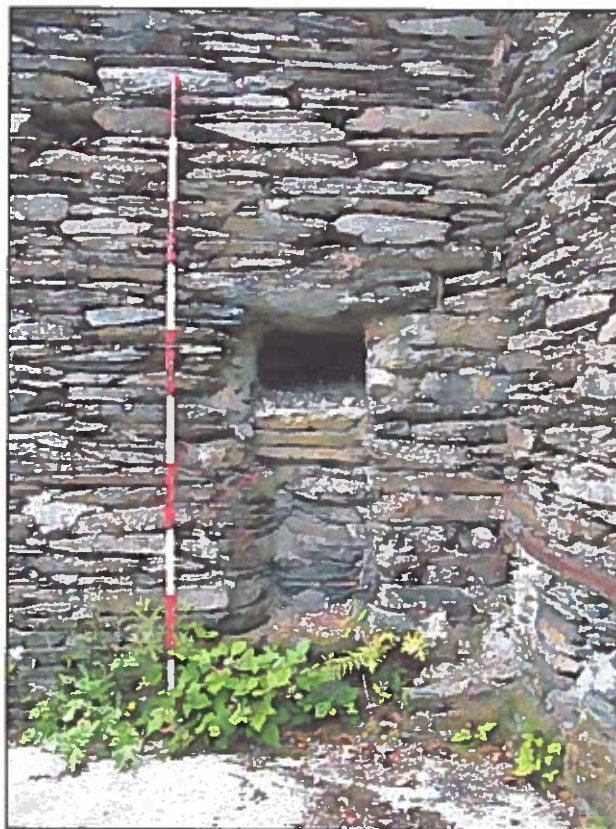
Plate 14. Chimney flue opening within north wall interior.
