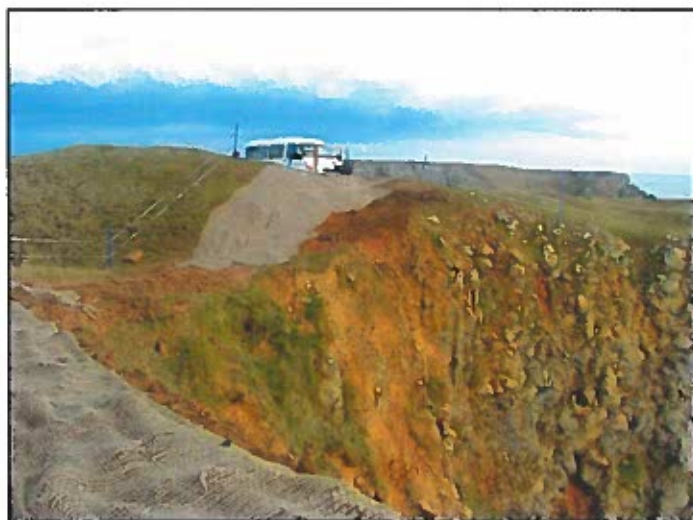
Inner rampart after repair, view to east
