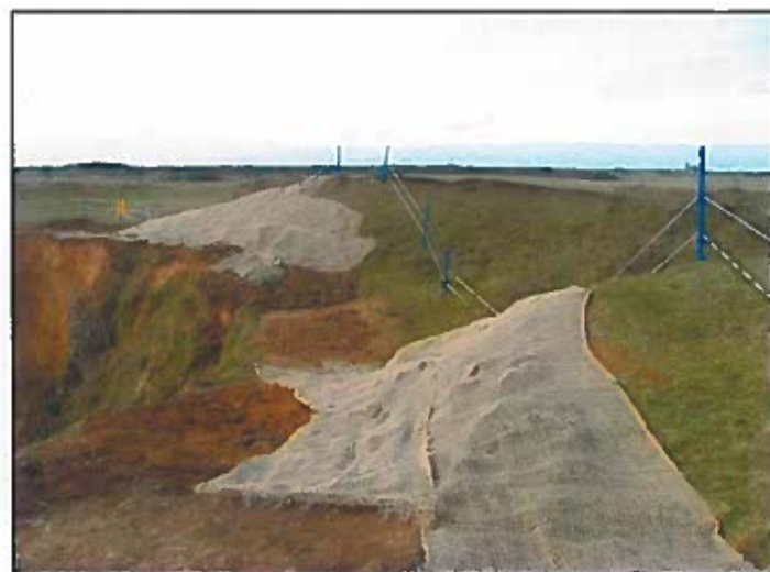
Inner and outer ramparts after repair, view to west
