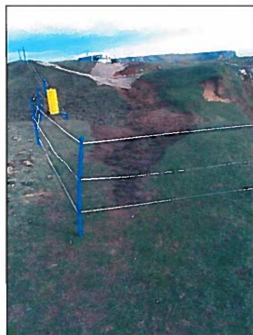
View of all repair sites, to the east
