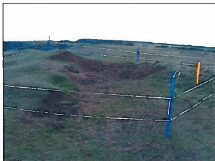
Outermost rampart and footpath, after re-turfing and repair
