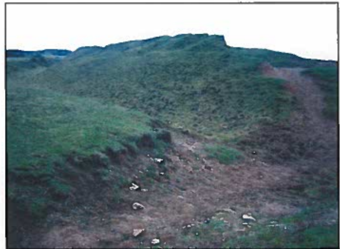
Coastal footpath, through the inner and outer banks, showing erosion
