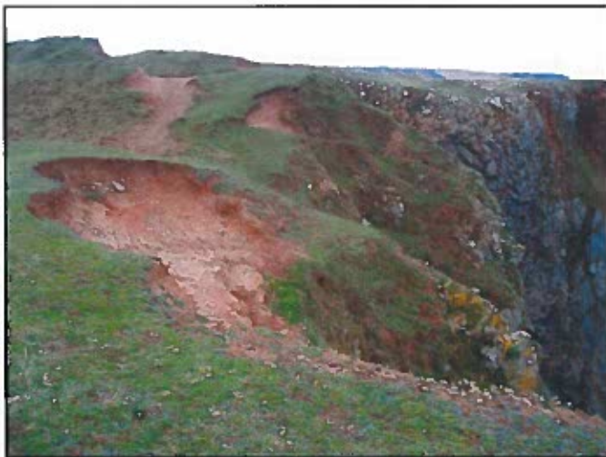
Erosion damage along the footpath, with ramparts in the background
