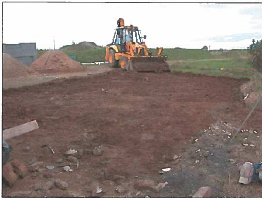
Plate 01: Area of development looking northwards after ground clearance of site to required depth.
