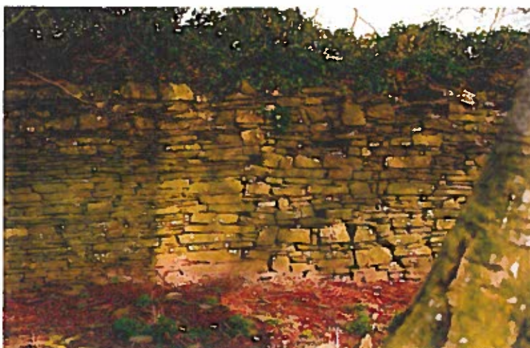
S2b The vertical junction between the wall which was new in 1748, left, and the long wall built in 1773, right.
