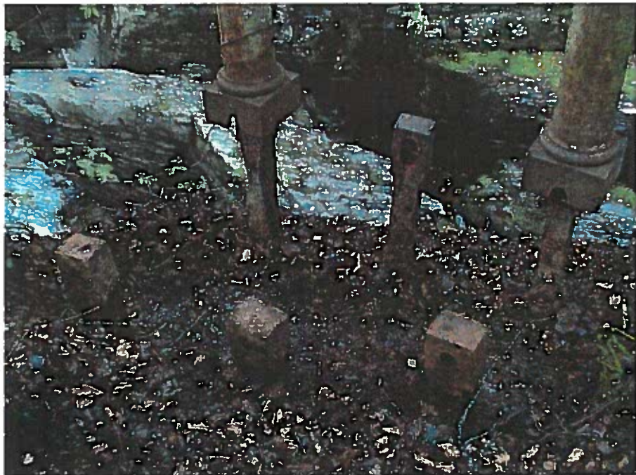
a) Before removal of anchorage rods.
