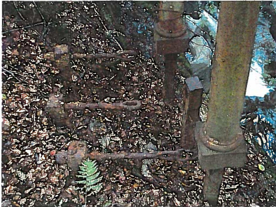
a) Before removal of anchorage rods.
