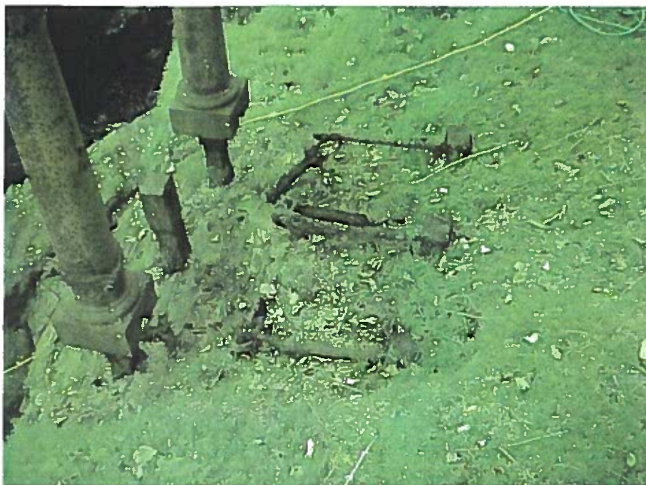
a) Before removal of anchorage rods.
