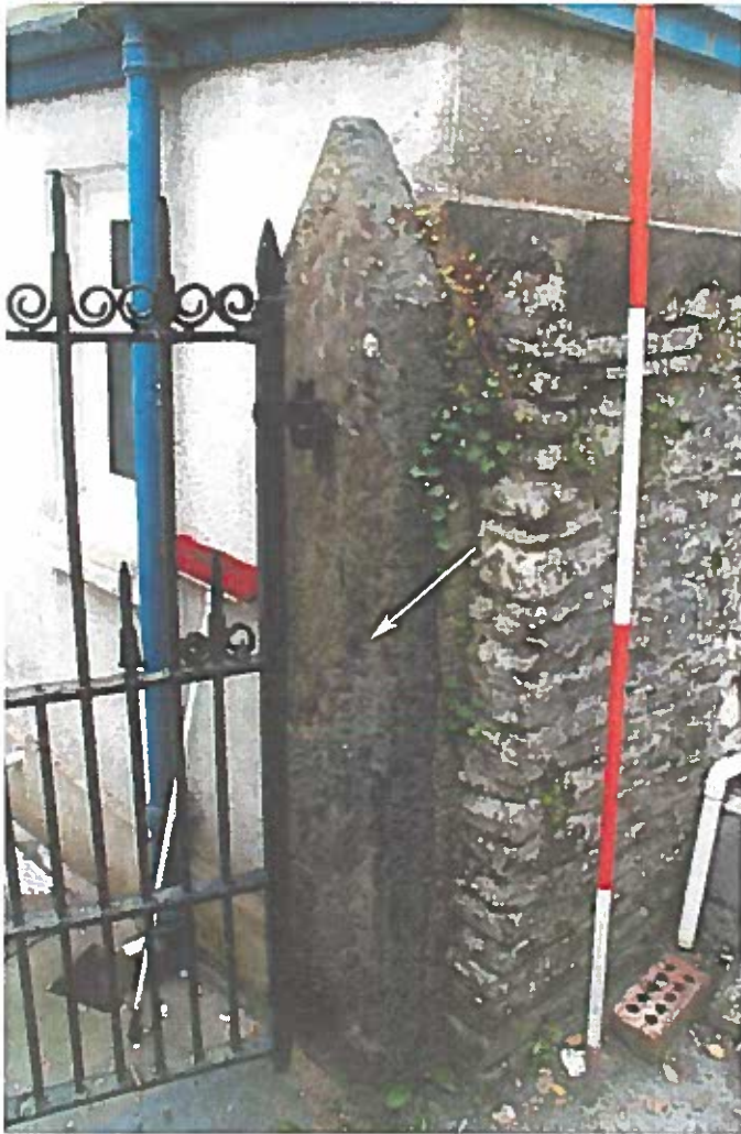
Fig. 2. Showing hole where another gate has been hung
