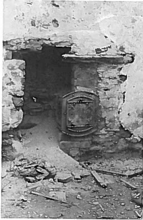
Fig. 16 Oven and inserted chimney in the East wall
