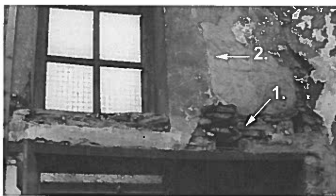
Fig. 11 Shows mortice cut beam (1), replaced by later iron girder, and probable line of gallery balustrade (2).
