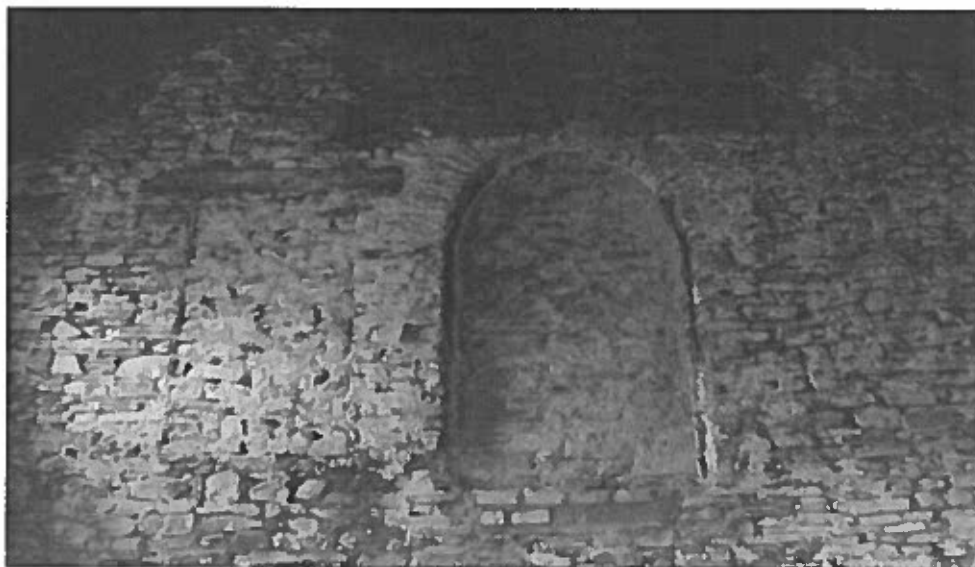
Fig. 5. Interior of west wall, when plaster was removed, showing two blocked openings. White shows location of plaster.
