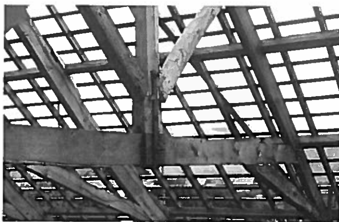
Fig. 9. King post of roof tree
