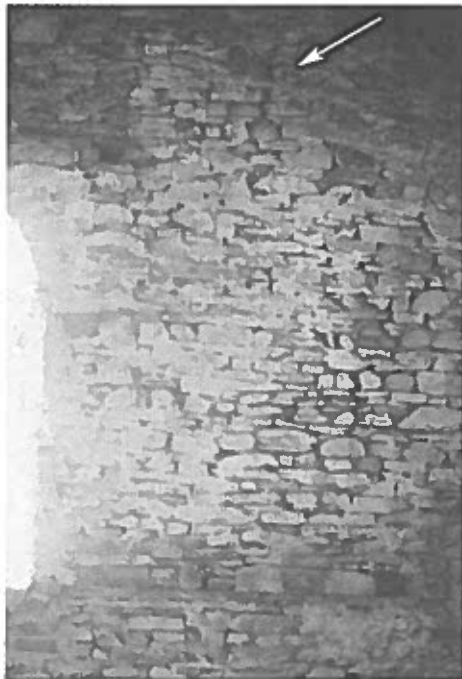
Fig. 6. Possible window in east wall. Arrow indicates line of previous gable
