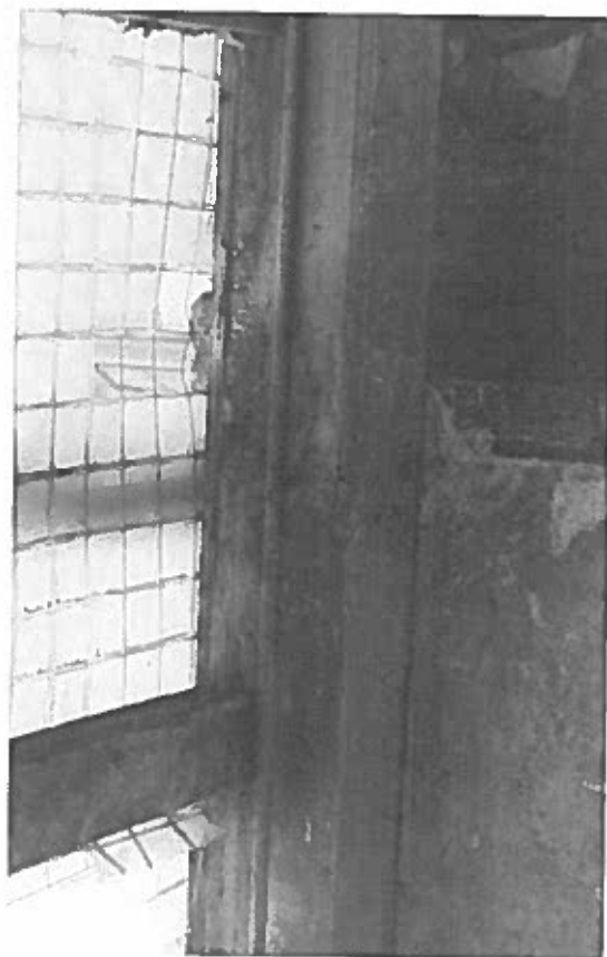
Fig. 15. Beaded jamb on central window, North wall.
