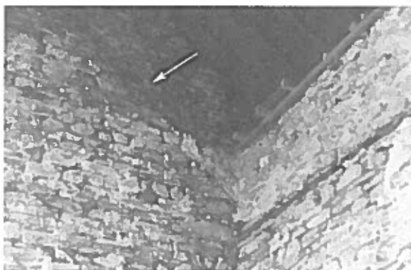
Fig. 8. Interior of west wall after removal of plaster. Arrow indicates previous line of gable.
