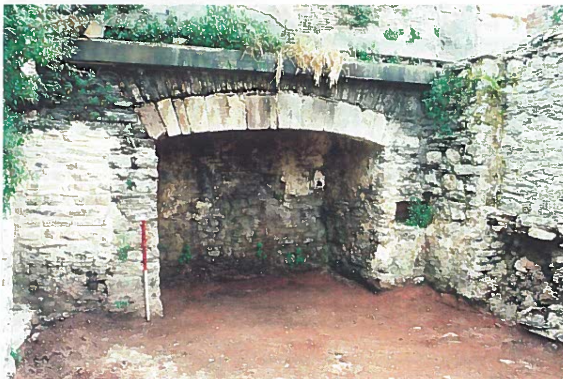
PLATE 2 CHIMNEY CUT INTO SOUTHERN GABLE FORMING THE LOWER SECTION OF AN EXTERNAL STACK
