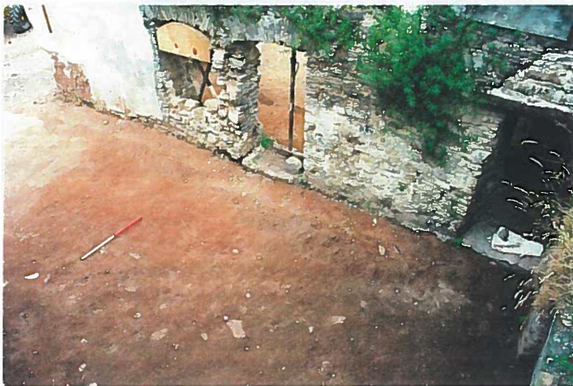
PLATE 5 KITCHEN AREA SHOWING FLOOR - FLAGSTONES ARE REMOVED
