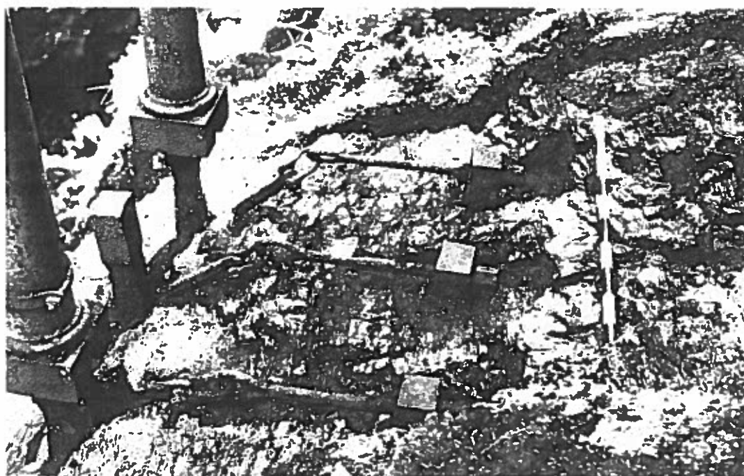
3/28a North excavation trench. View of the anchor pins, anchor rods and bolts, cable stirrups, corroded ends of cables which supported the bridge gangway, and the guide pins and columns. Also cuts in the bedrock to accommodate the anchor pin heads and rods. Looking west.
