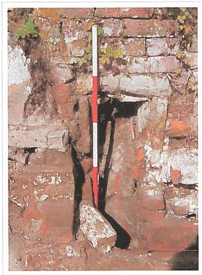
Plate 27: Wall Flue taking furnace gases out of Glass House. (Scale 1m. looking west)
