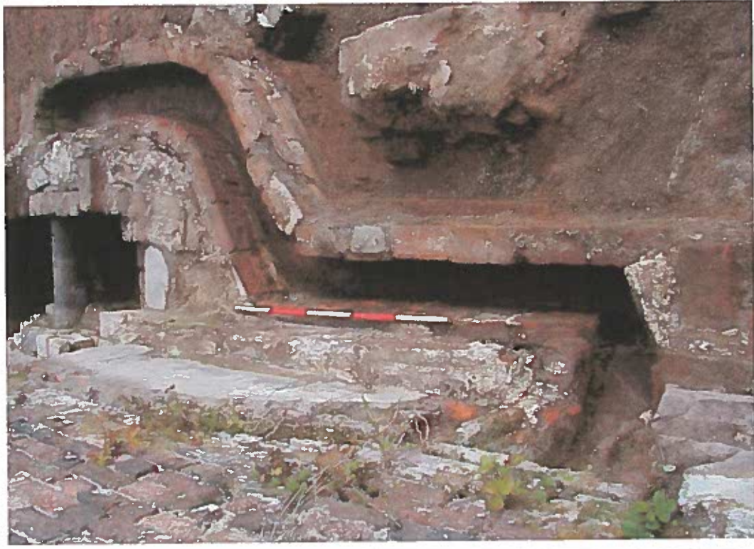
Plate 26: Gas Flue for Southern Furnace with capping removed. (Scale 1m. looking north)
