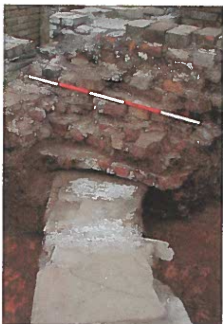
Plate 15: Cold air return flue with capping, entering hot air chamber of southern furnace. (Scale 1m. looking west)
