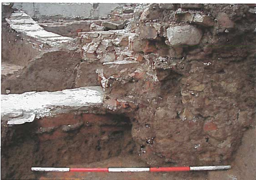
Plate 17: Cold air return flue entering hot air chamber of southern furnace. (Scale 1m. looking south)
