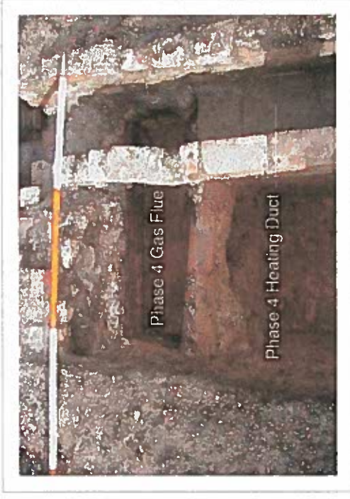
Plate 3: Detail of hot air and gas vents, revealed during 2000 excavations. (Scale 2m. looking west)
