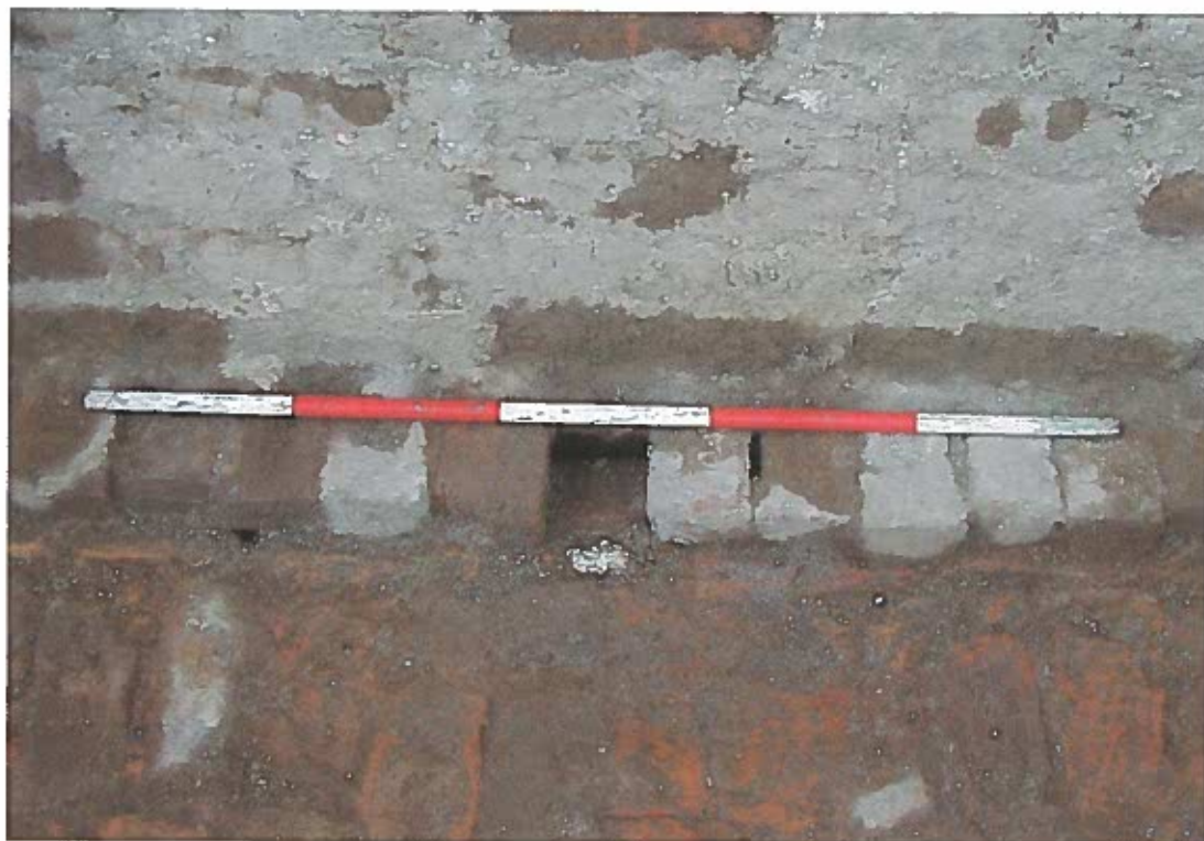
Plate 31: Brick culvert at base of west wall, southern room of Glass House. (Scale 1m. looking west)
