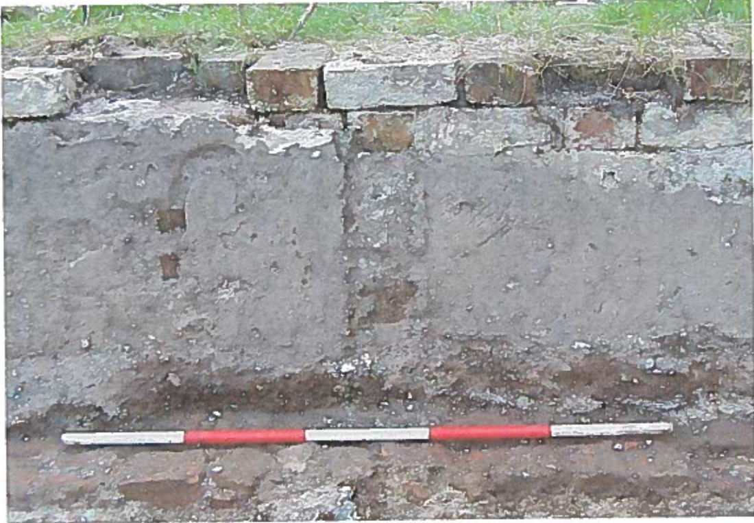
Plate 38: Detail of upper south wall of southern room (phase 4) showing upright beam impression in mortar. (Scale 1m. looking south)
