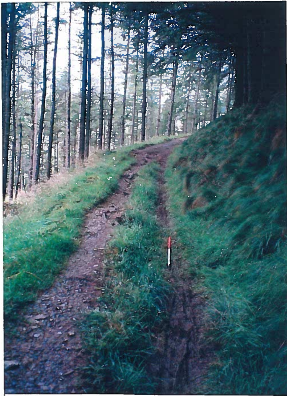
Plate 3 Section through conifer crop showing much disturbed section of leat, prior to work being undertaken. The spread of the outer bank inwards has included total removal of the topsoil and the leat is seen to be extremely silted-up.
